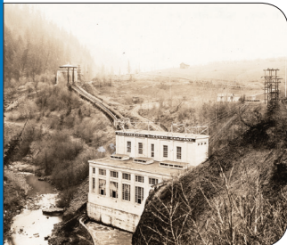
Condit Powerhouse during the early years of operation
