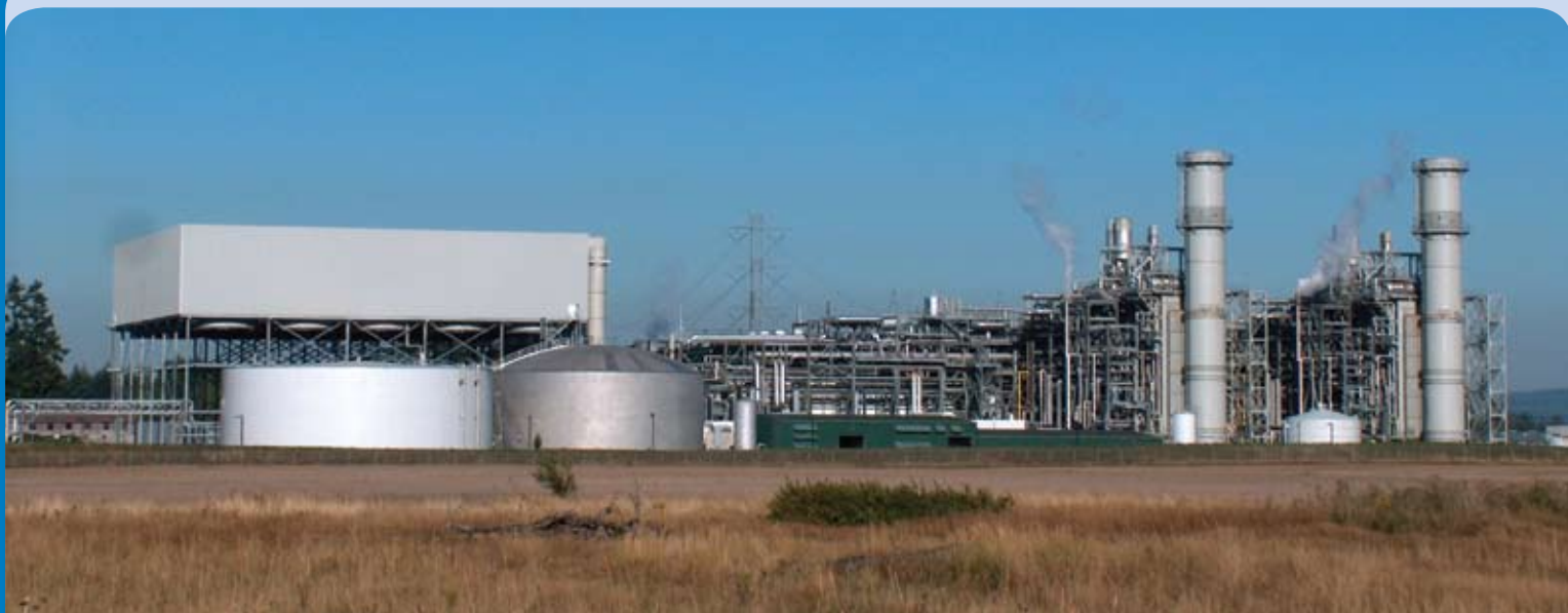
Chehalis Generation Facility
