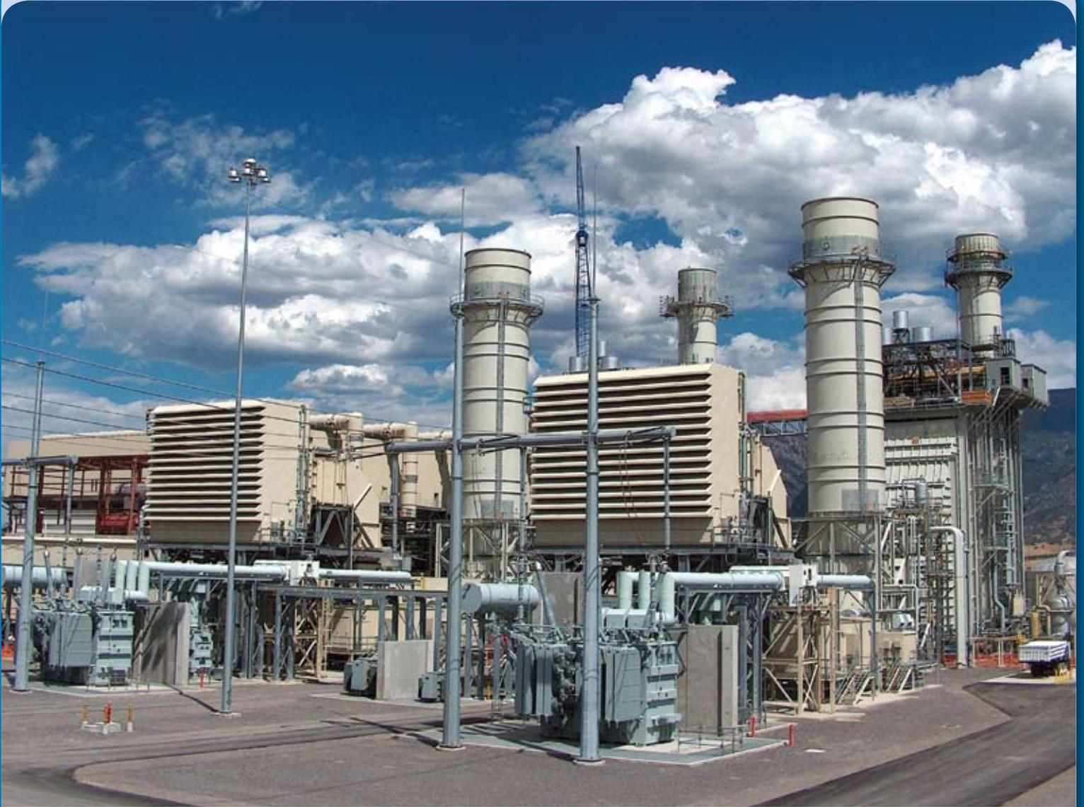
**Currant Creek Plant blends modern technology with environmental stewardship on a 160-acre site in an area of the same name near Mona, Utah. Our twin combined-cycle gas turbines and steam turbine are capable of generating 550 megawatts of electricity and the plant is 30 to 48 percent more efficient than a comparable coal-fueled steam plant.**
