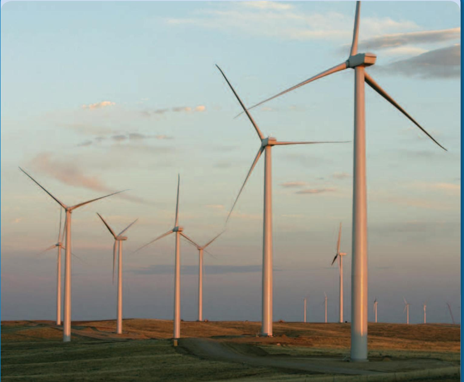
Sixty-six turbines near Glenrock, Wyo., borrow the wind to generate as much as 99 megawatts of energy. Completed in 2008, they stand on land that PacifiCorp retired and reclaimed from surface coal mining operations. We believe this is the first wind facility in the West to recycle land that once provided fossil fuels into one that captures renewable energy.
