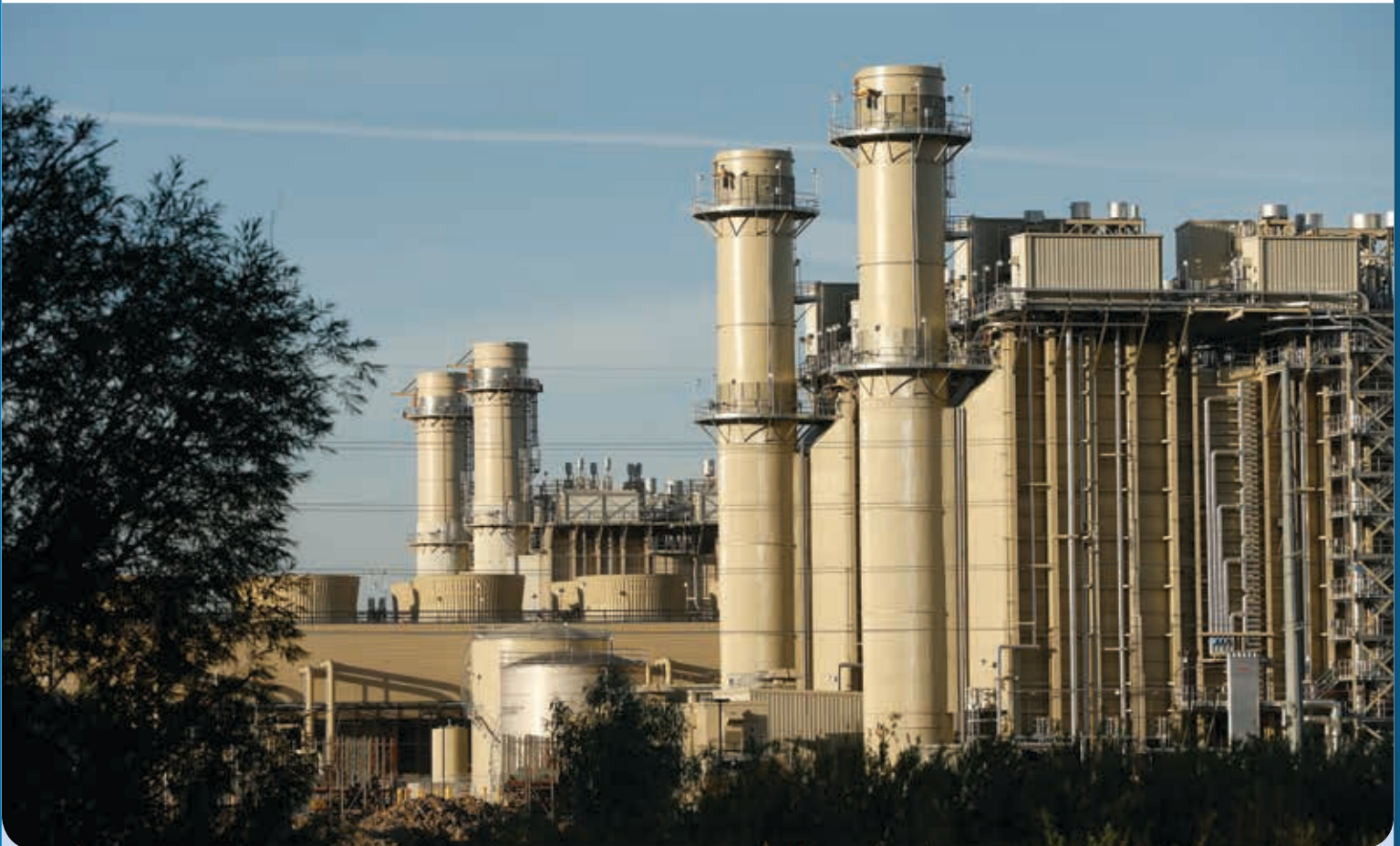
Lake Side 1 and Lake Side 2 (foreground) Generation Facilities
