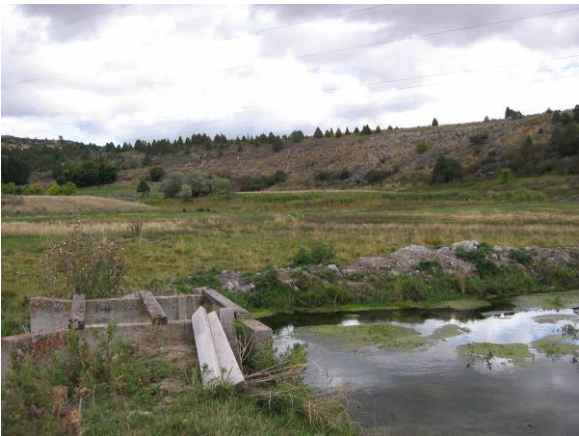
Photo 20. Kackley Spring water control structure.
