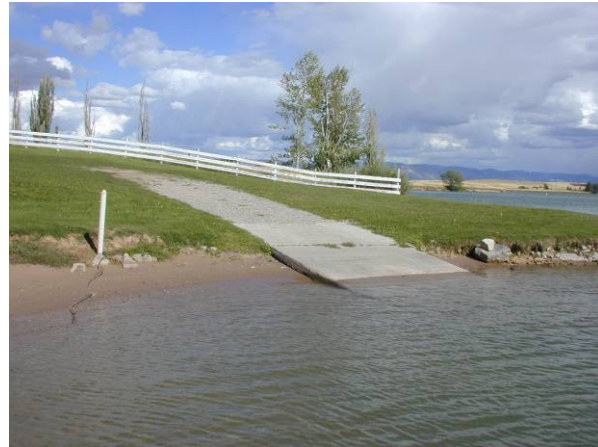
Photo 9. Hand boat launch at Soda Powerhouse DUA.
