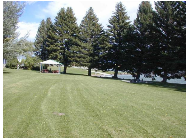
Photo 5. Soda Powerhouse DUA.
