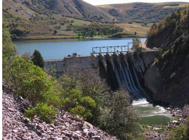
Photo 1. Oneida Reservoir and dam.
