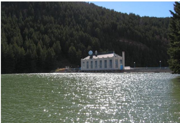
Photo 2. Soda Powerhouse and Alexander Reservoir.
