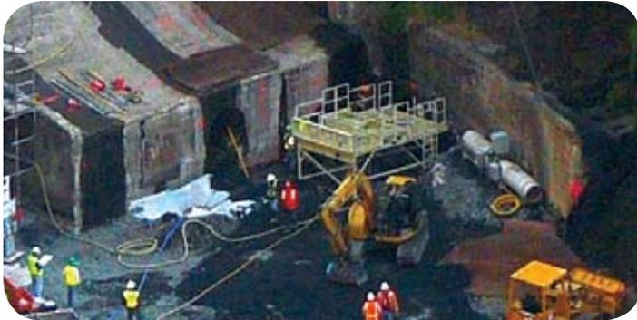
Workers constructing the drain tunnel at Condit Dam – September 2011
