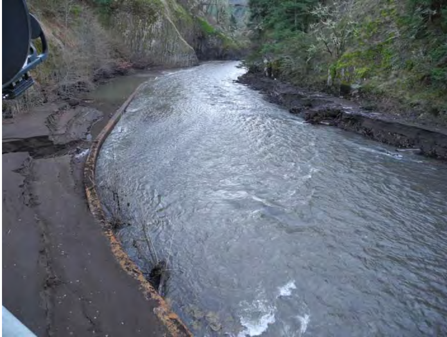
White Salmon River at the powerhouse. View downstream. Temporary bed sediment levels can be inferred from the deposition on river right. On river left the powerhouse tailrace is presently filled with sediment. 12-7-2011.
