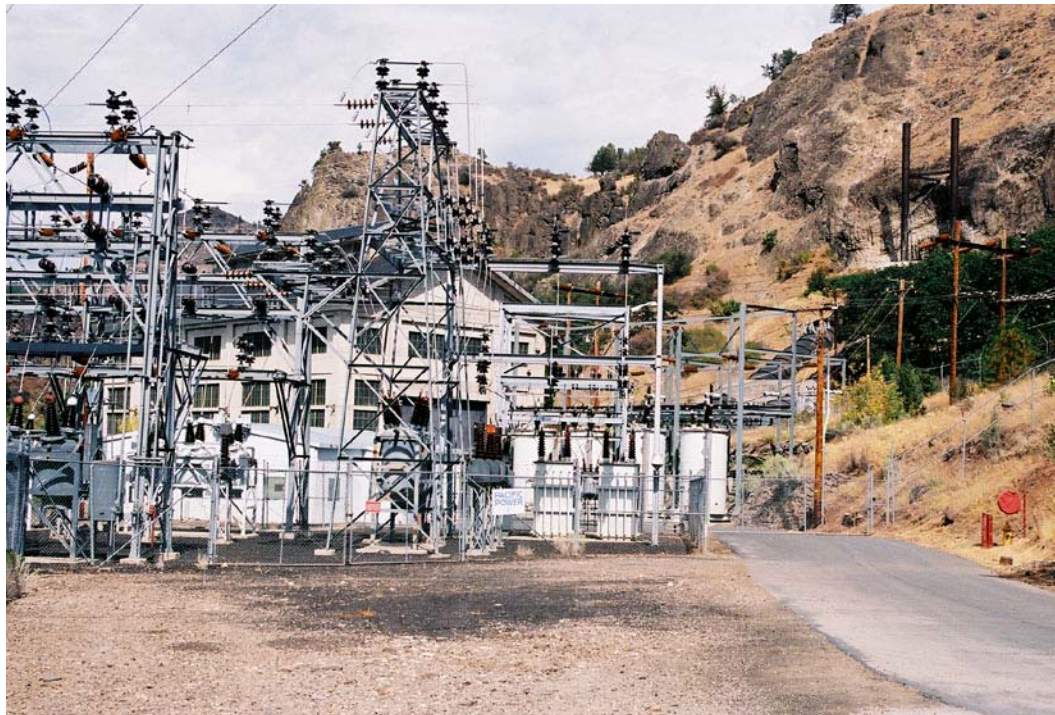
C6: COPCO NO. 2 POWERHOUSE
