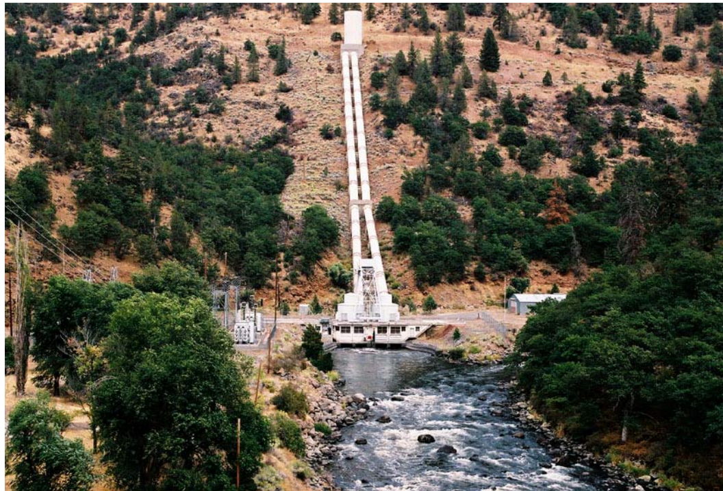
BB8: J.C. BOYLE POWERHOUSE AND PENSTOCKS
