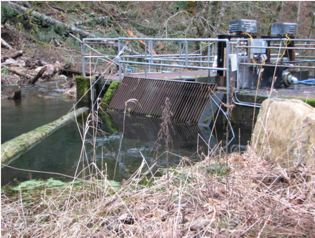
Photograph 2. Upstream View of the Intake
