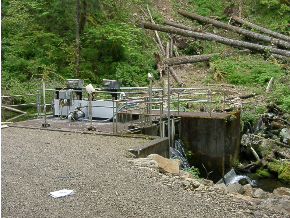
Photograph 1. Downstream View of the Intake
