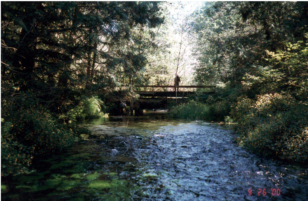
Figure 4.9-12. Typical low clearance log stringer bridge in lower Speelyai Creek. (Habitat Unit 32, approximately 0.8 mile upstream from Speelyai Hatchery intake)
