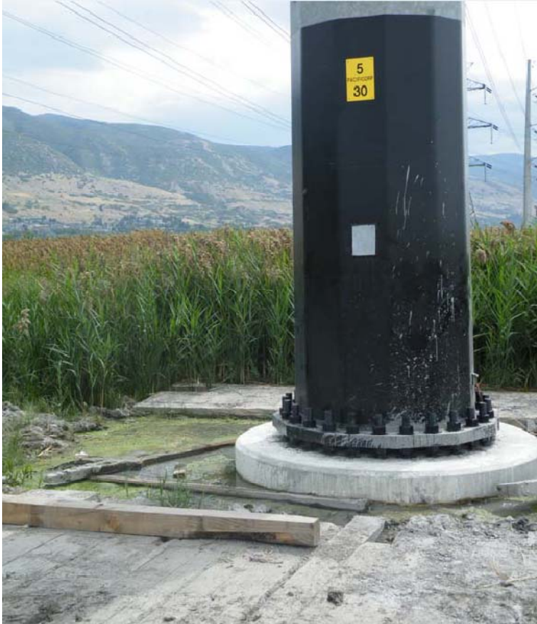
Wetlands area while under construction
