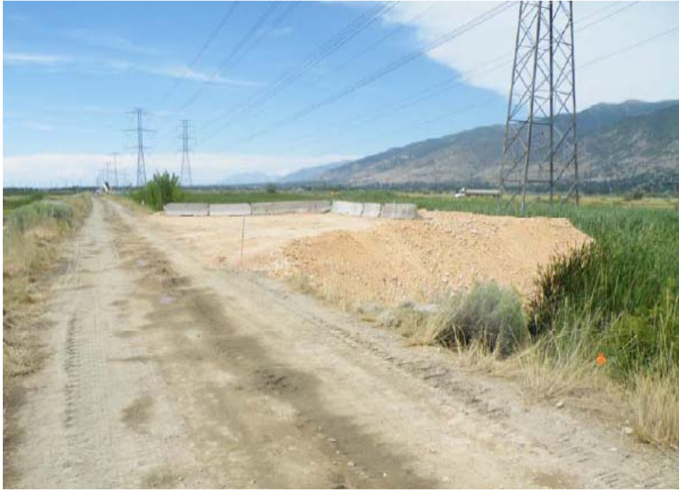
Temporary fill for construction
