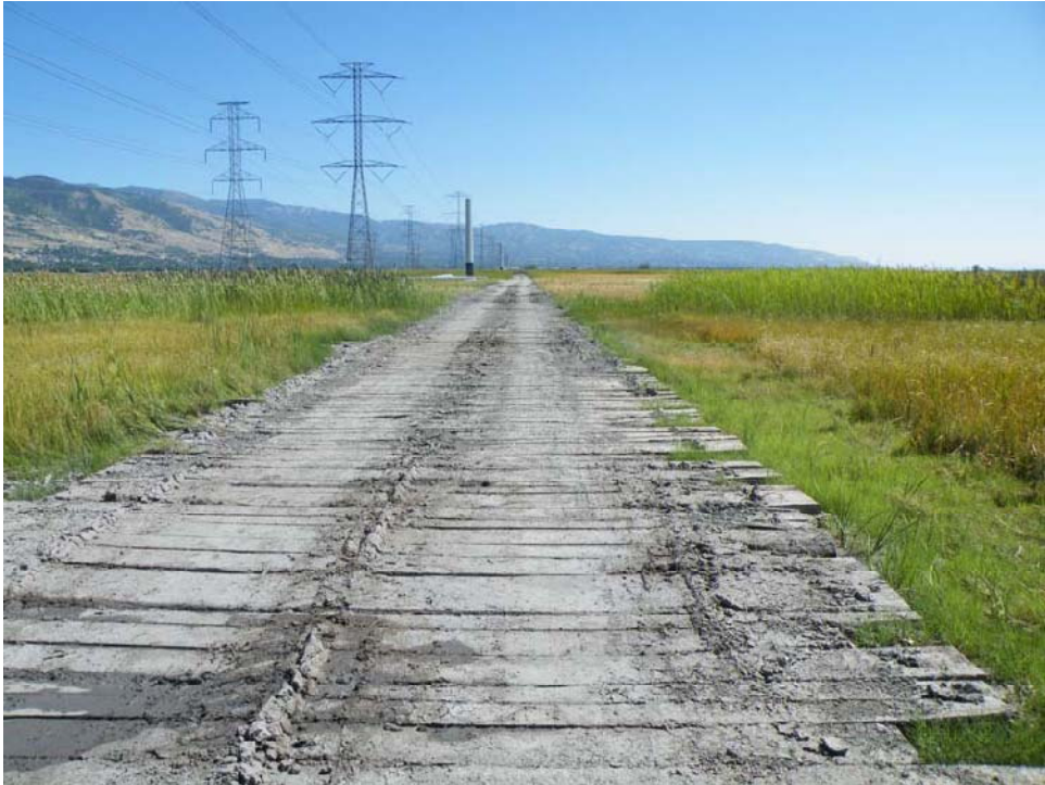
Crane mat access to construction site
