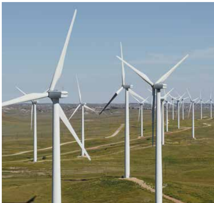
The single painted blade stands out prominently among the non-painted blade turbines.
