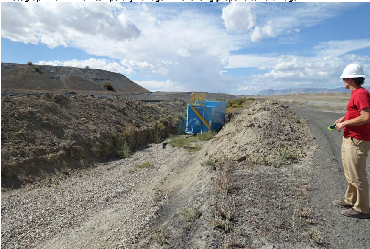
Photograph No. 22 View of frac tank. Installed in perimeter ditch.
