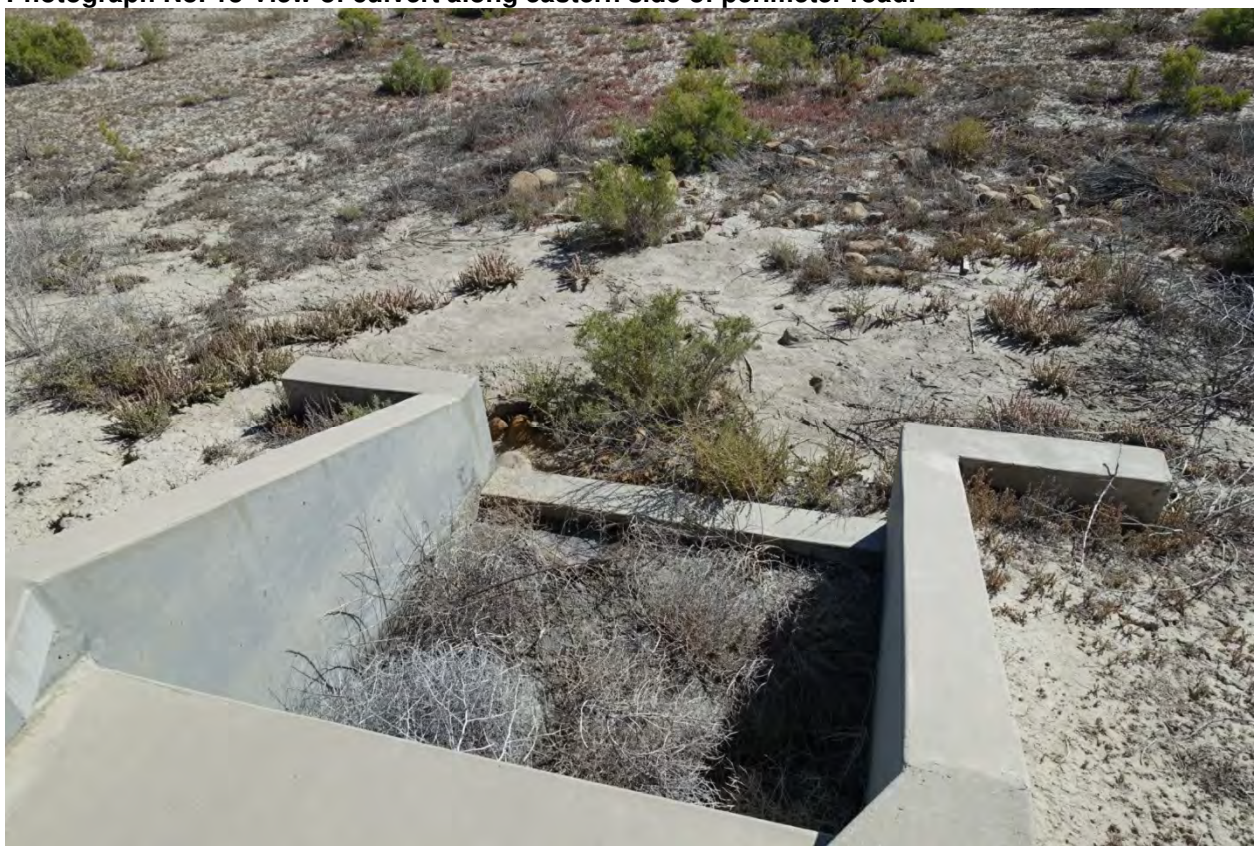
Photograph No. 14 View of retention basin outlet.
