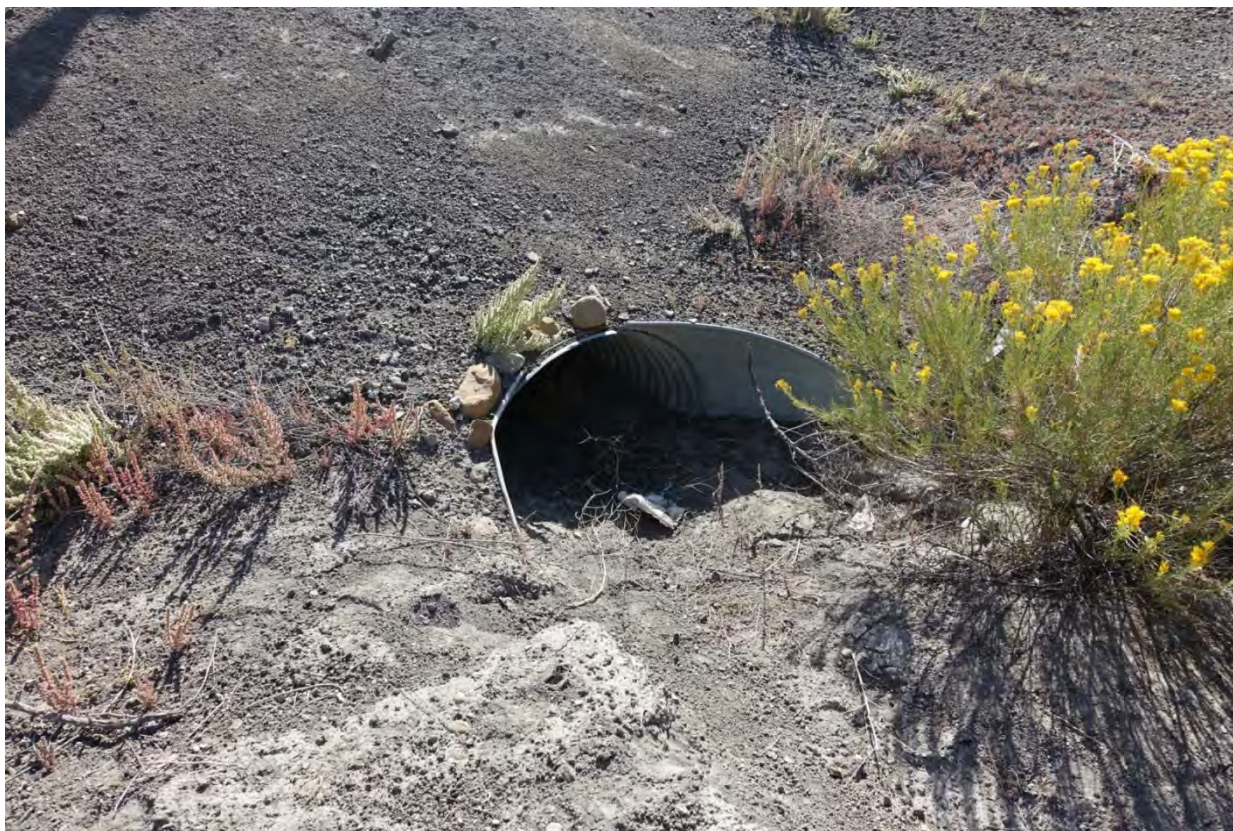
Photograph No. 17 View of plugged culvert along northern slope. East side of road.
