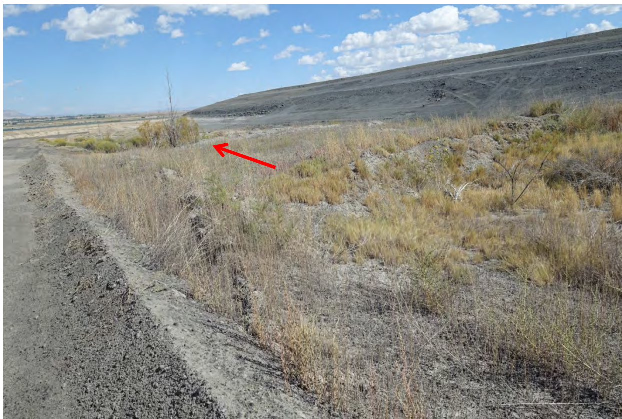
Photograph No. 21 View temporary “bridge.” Preventing proper ditch drainage.
