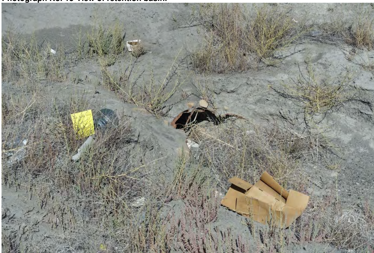
Photograph No. 16 View of plugged culvert along northern slope. West side of road.
