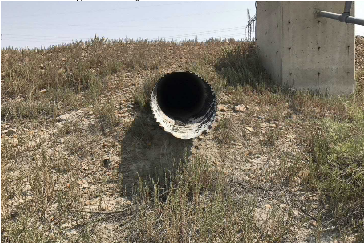
Photograph No. 31 View of auxiliary spillway (upstream end) adjacent to the slide gate control structure, looking approximately east. The pipe is unobstructed at this end.
