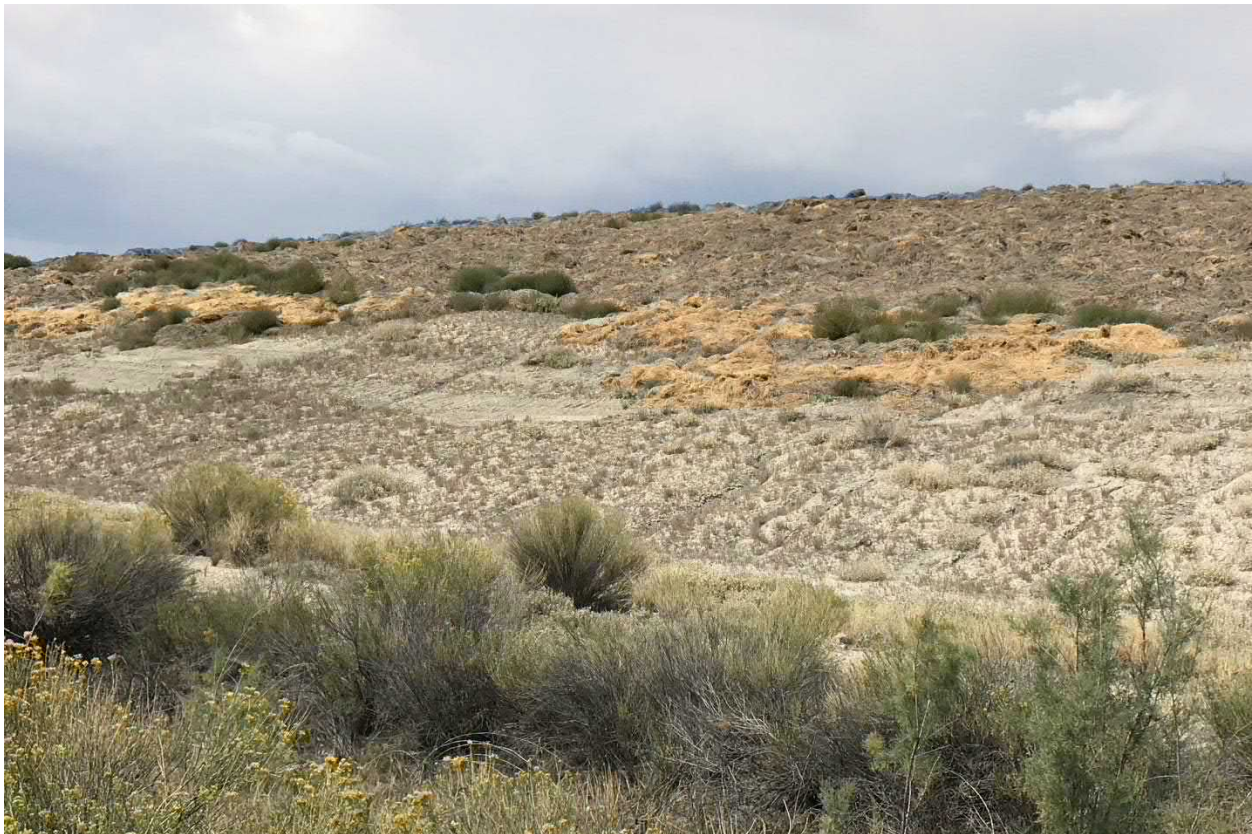
Photograph No. 21 View of southeast ash slope, looking west. Slope has been treated with straw for erosion protection on the top portion of the slope.
