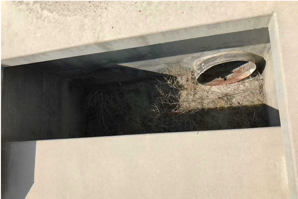
Photograph No. 32 View of auxiliary and primary spillway (downstream end), looking down into energy dissipation structure. Inspection team did not inspect downstream end of pipes.
