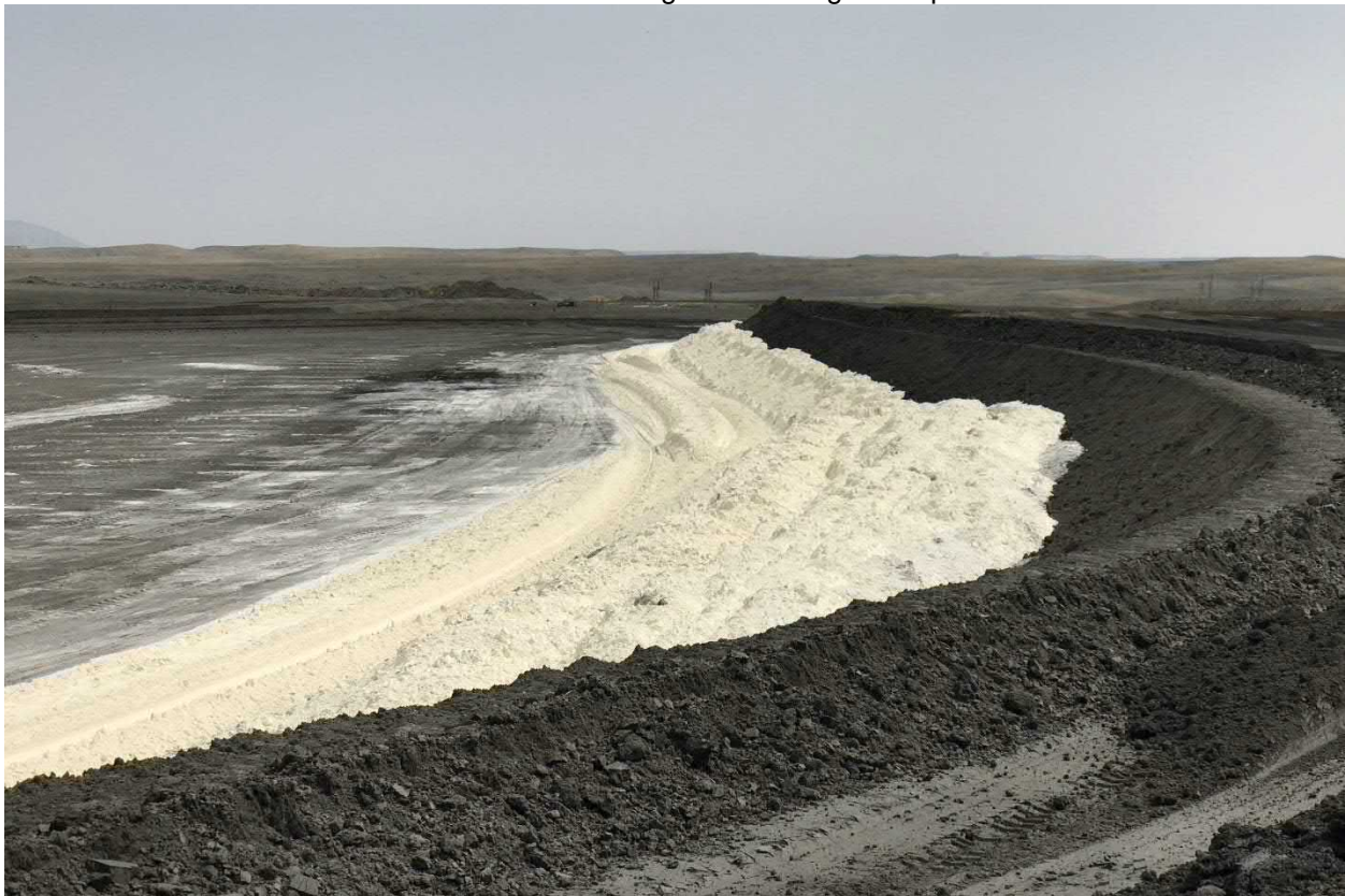
Photograph No. 40 View of FGD gypsum disposed of in the active area of the CCR Landfill, looking approximately southeast.
