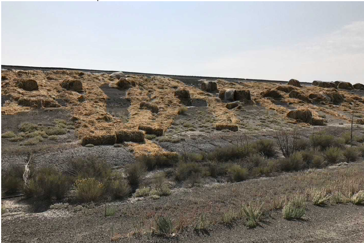
Photograph No. 7 View of straw on west ash slope to help with erosion control and establishment of vegetation, looking approximately south.
