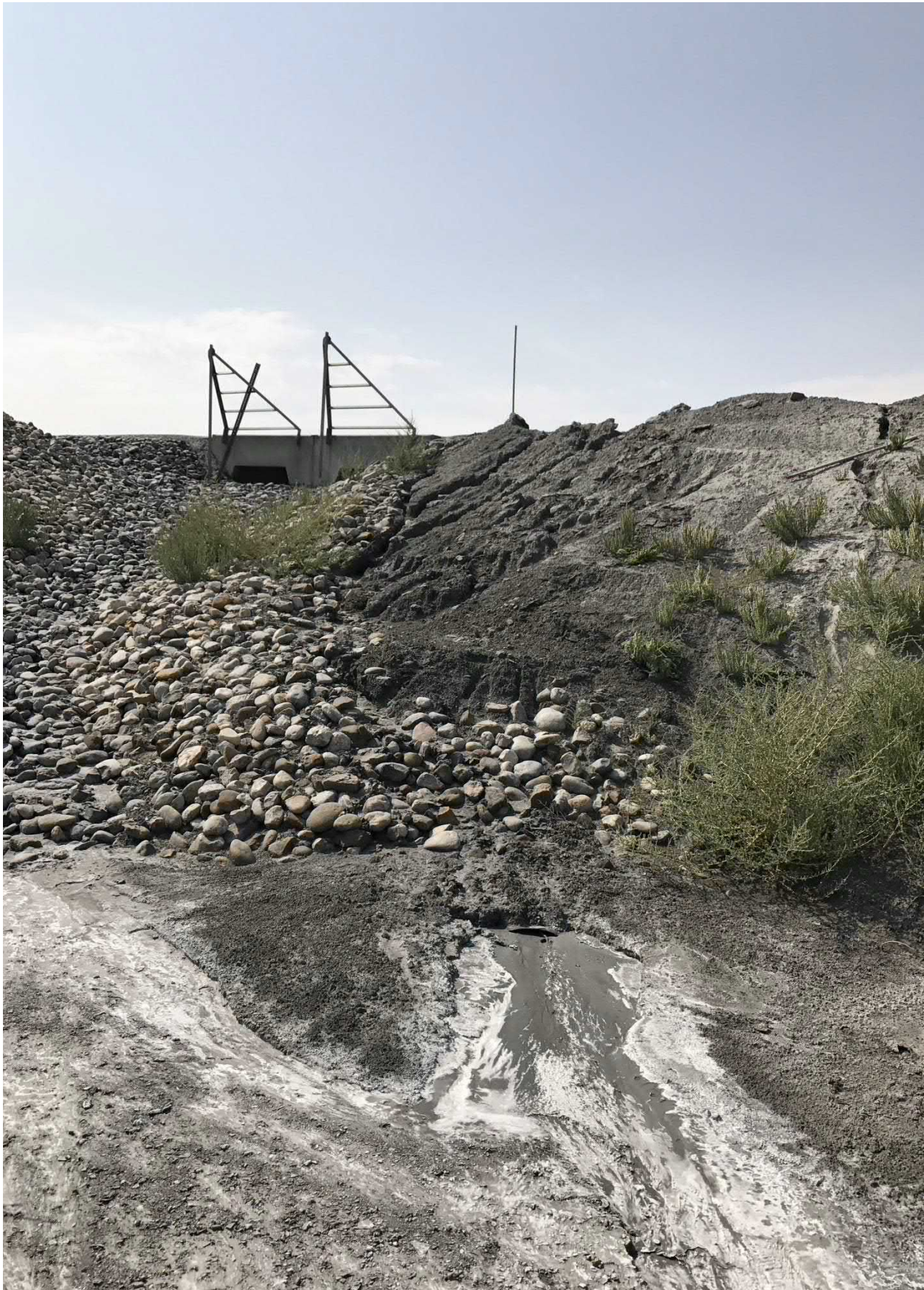
Photograph No. 5 View of rumble rack as tire cleanout and runoff break at entrance/exit to CCR Landfill on south haul road, looking southwest. Note armored ditch for runoff.
