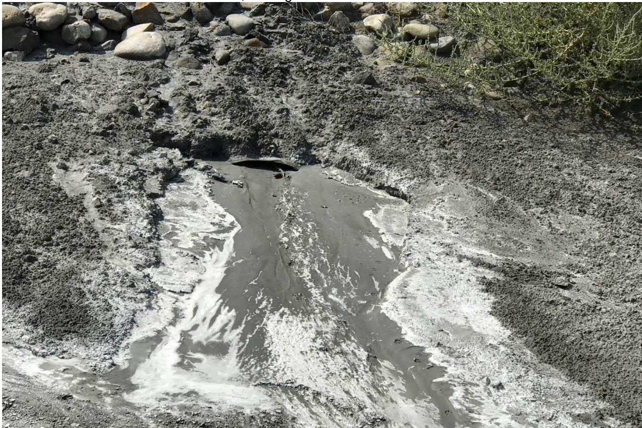
Photograph No. 4 View of pipe culvert (downstream side), which was almost completely blocked, under south haul road, looking southwest.
