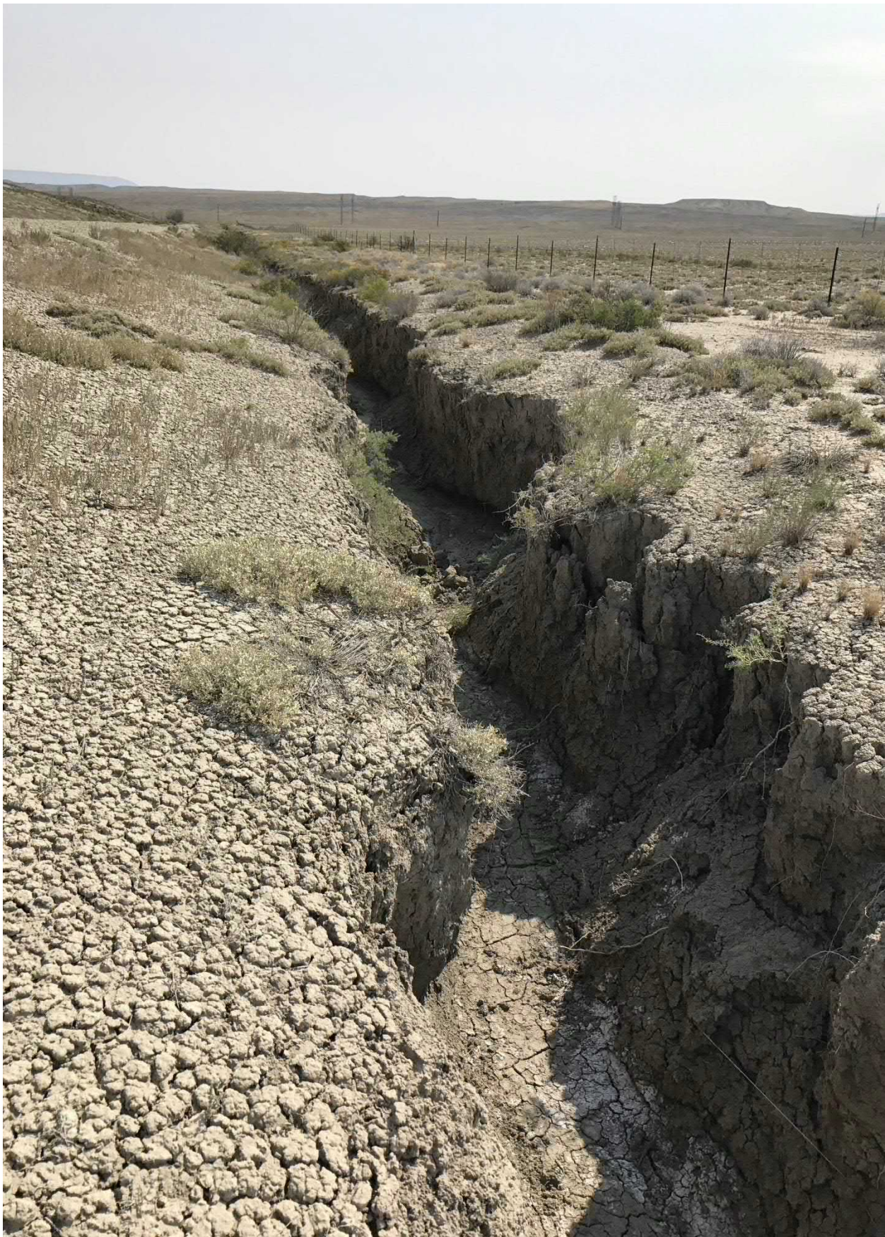
Photograph No. 12 View of drainage ditch diverting offsite runoff around permitted CCR Landfill, looking east. Note erosion and steepened earthen sides of the channel.
