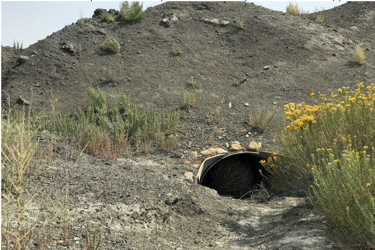
Photograph No. 33 View of retention basin north inlet pipe (upstream end), looking east-southeast. Pipe culvert was partially obstructed by soil and debris.
