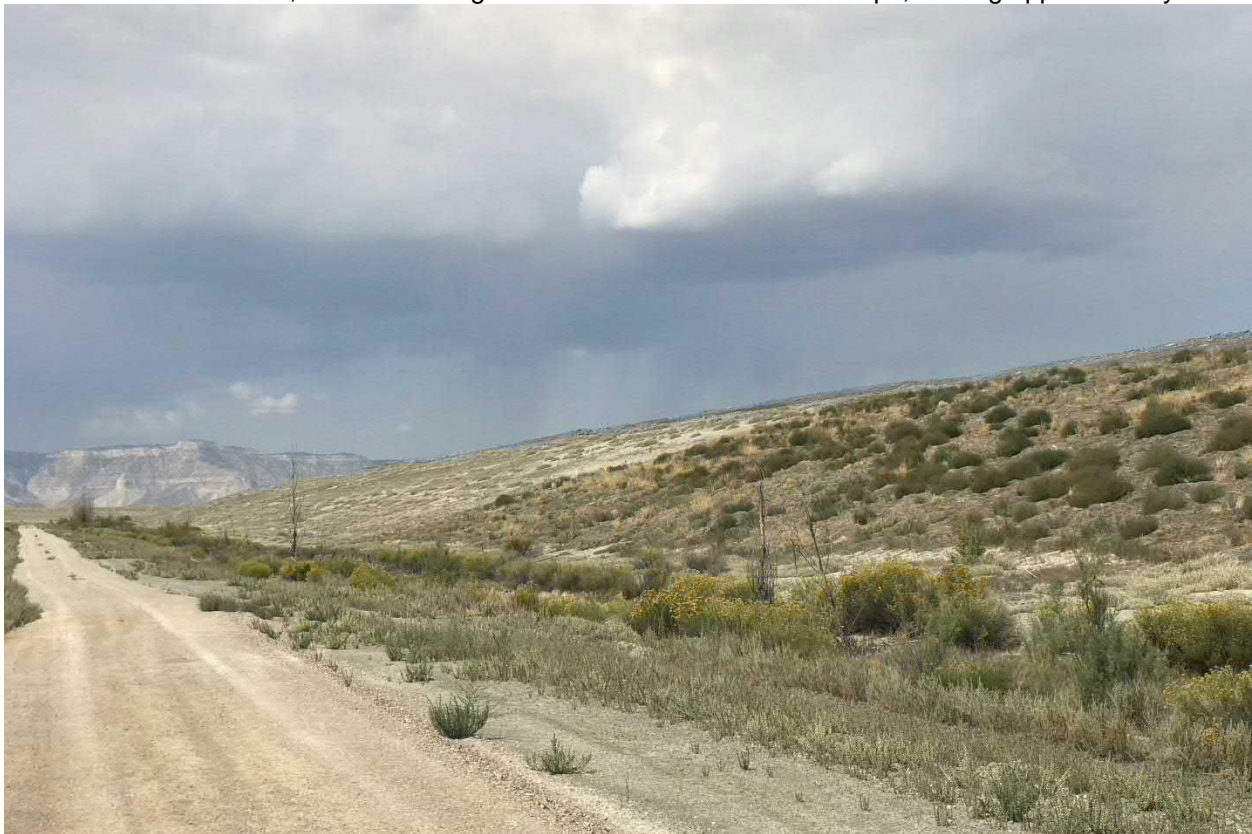
Photograph No. 16 View of south exterior slope of landfill. Note vegetation growth on straw-treated slope compared with untreated slope.
