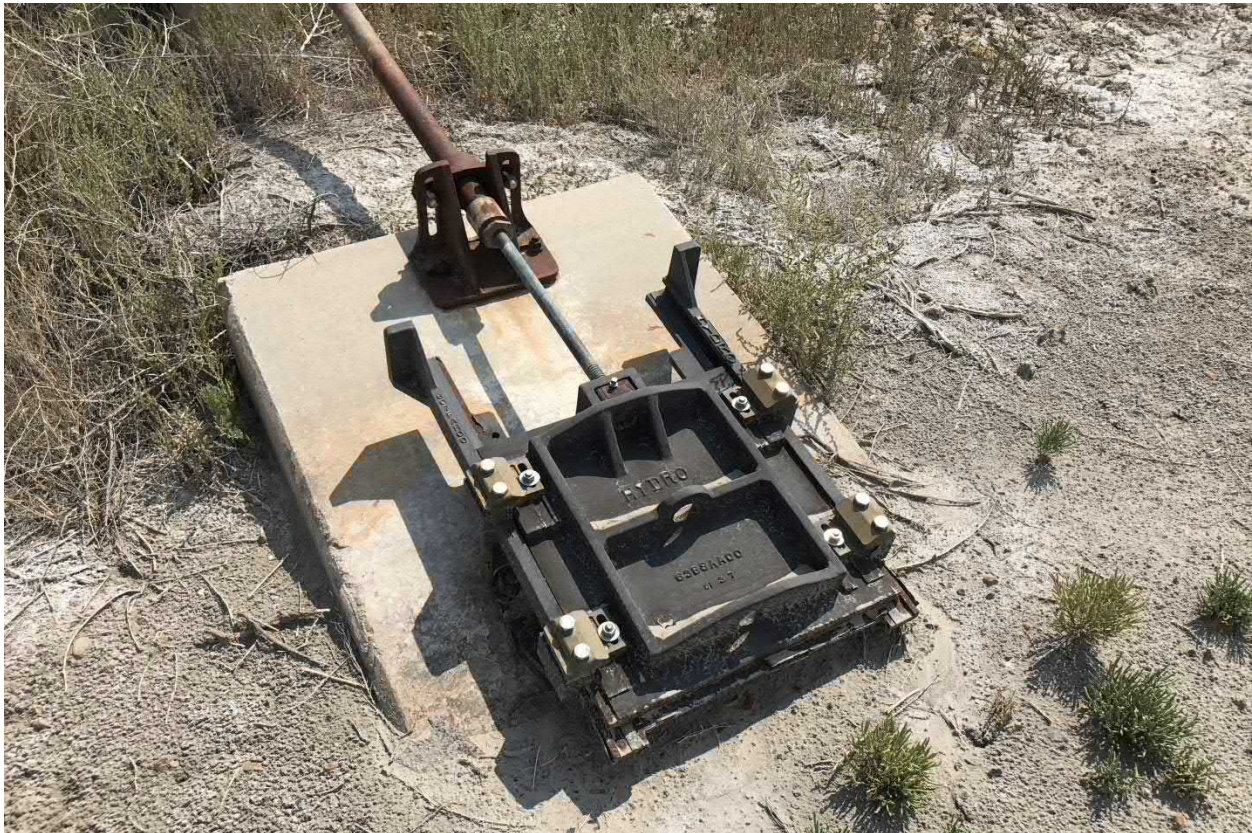
Photograph No. 30 View of outlet slide gate and outlet pipe structure, looking southeast. The slide gate appeared to be in good condition.
