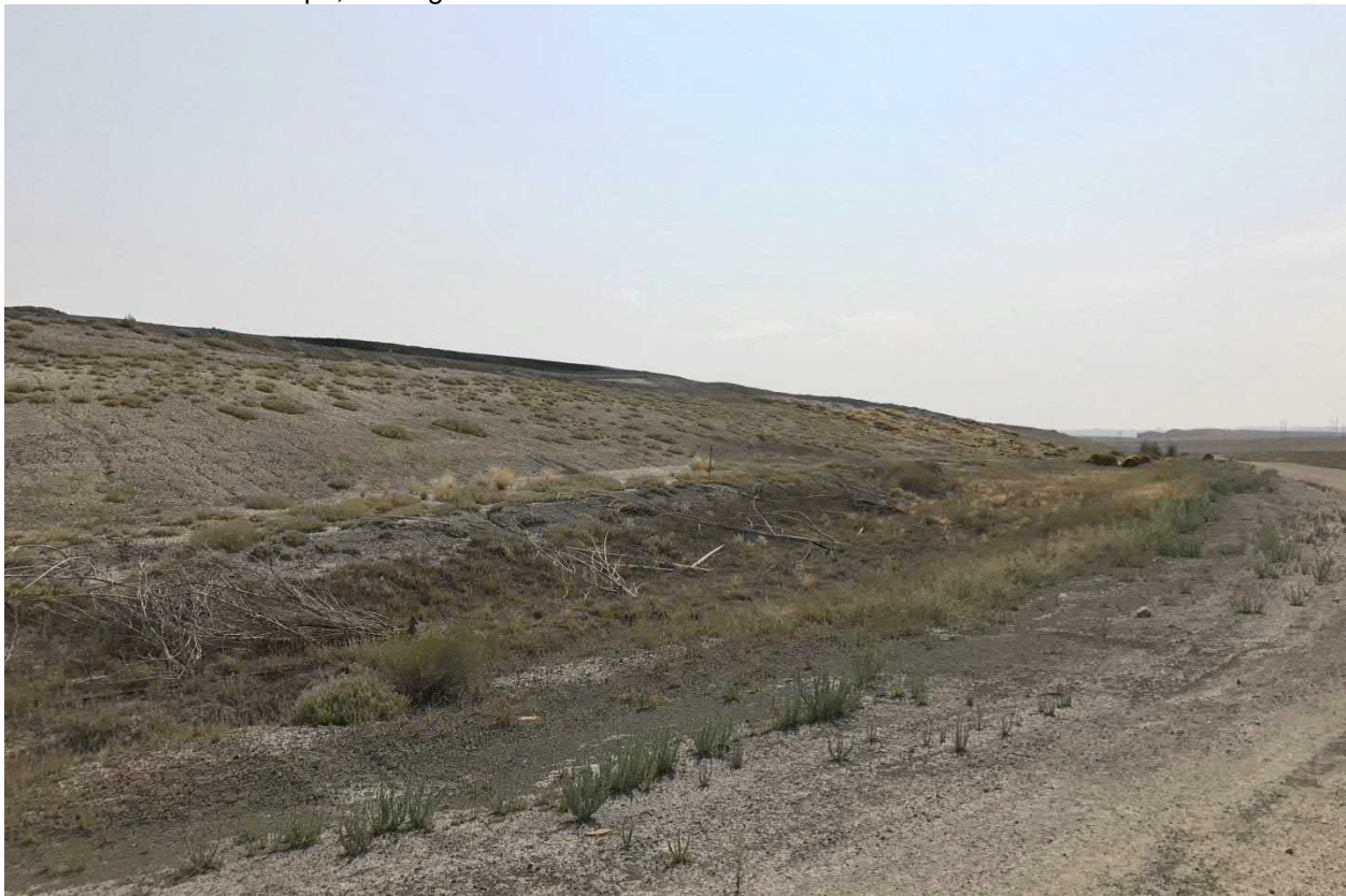
Photograph No. 9 View of southwest ash slope and onsite runoff collection ditch running along the toe of the slope, looking southeast.
