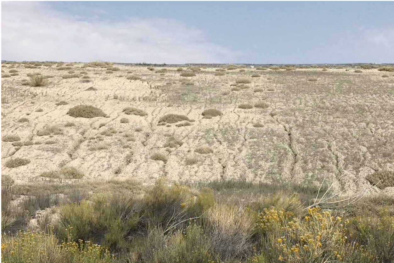
Photograph No. 15 View of typical south exterior slope with sparse vegetation, widespread erosional rills, and thicker vegetation beneath the toe of the slope, looking approximately north.
