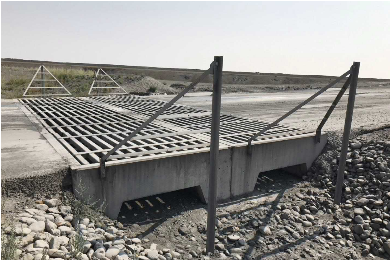
Photograph No. 3 View of rumble rack as tire cleanout and runoff break at entrance/exit to CCR Landfill on south haul road, looking northeast.
