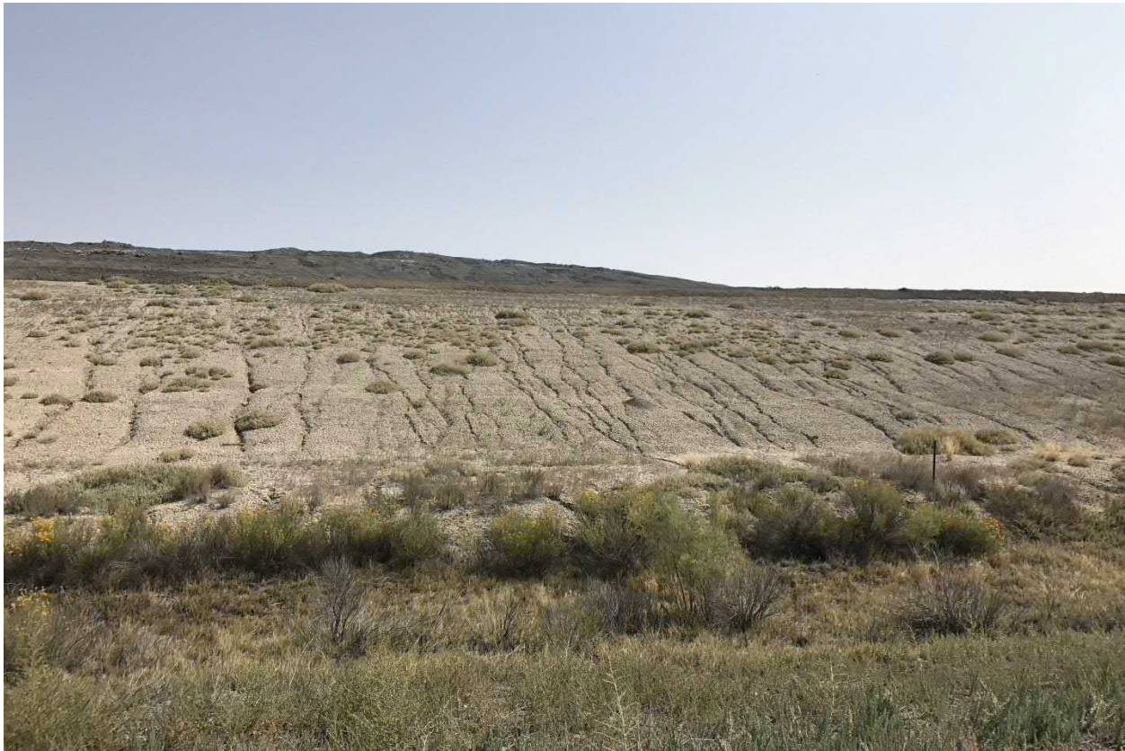
Photograph No. 10 View of typical west exterior slope with sparse vegetation, widespread erosional rills, and thicker vegetation beneath the toe of the slope, looking approximately northeast.
