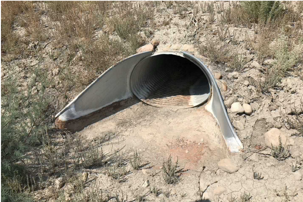
Photograph No. 24 View of south retention basin inlet pipe (upstream end). Pipe culvert was unobstructed and free of debris, looking northwest.
