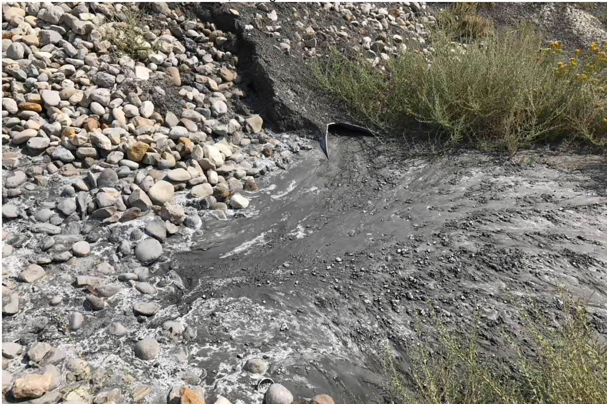
Photograph No. 2 View of pipe culvert (upstream side), which was almost completely blocked, under south haul road, looking southeast.
