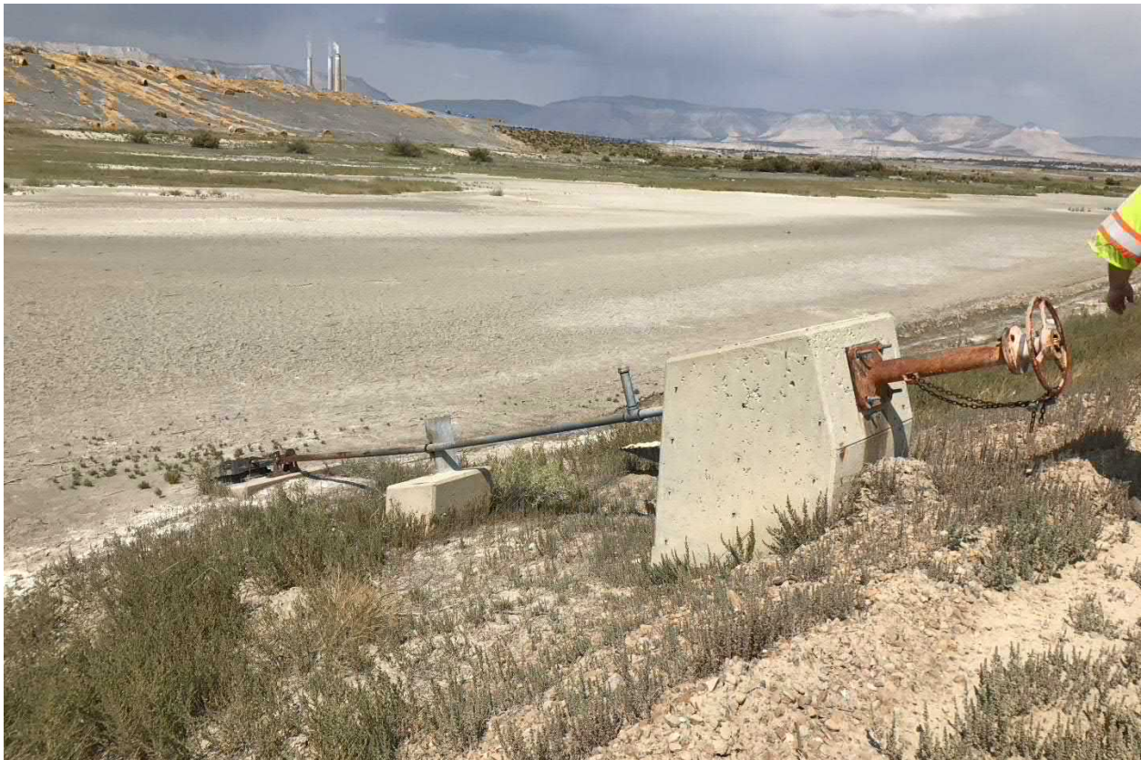
Photograph No. 29 View of outlet gate and gate control, looking northwest. This facility is a zero-discharge facility and gate remains closed.
