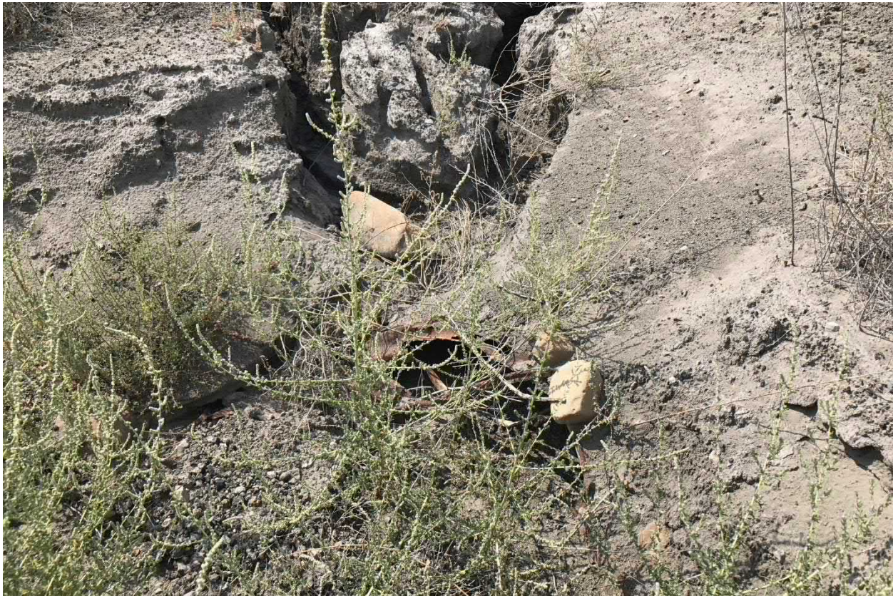
Photograph No. 35 View of retention basin north inlet pipe (downstream end), looking southwest. Pipe culvert was almost completely obstructed by debris. Pipe outlet partially collapsed.
