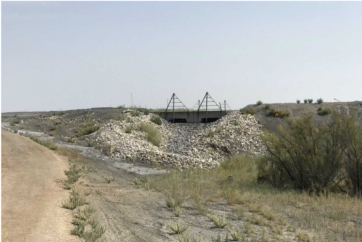
Photograph No. 1 View of rumble rack as tire cleanout and runoff break at entrance/exit to CCR Landfill on south haul road, looking northeast. Note armored ditch for runoff.
