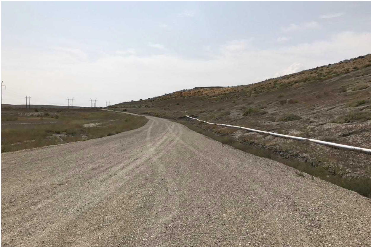
Photograph No. 26 View of drain line from underdrains to Frac tank (see Photograph No. 27), looking south-southwest.
