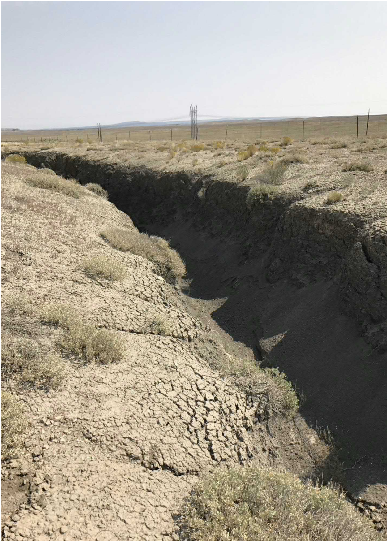
Photograph No. 19 View of drainage ditch diverting offsite runoff around permitted CCR Landfill, looking approximately east. Note erosion and steepened earthen sides of the channel.
