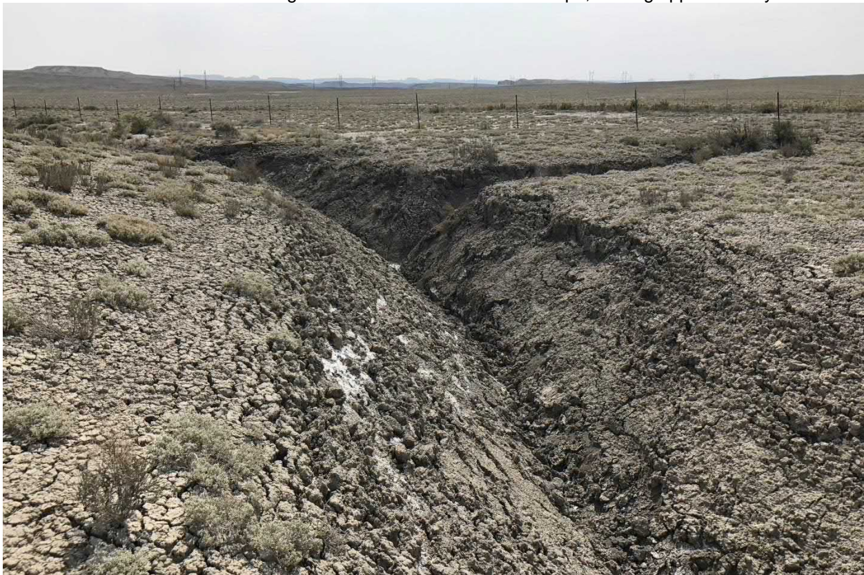
Photograph No. 11 View of drainage ditch diverting offsite runoff around permitted CCR Landfill, looking south-southeast.
