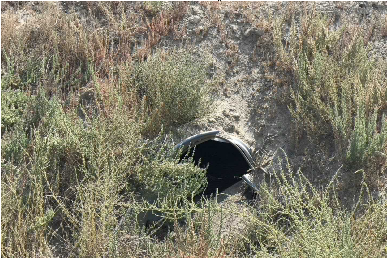
Photograph No. 25 View of south retention basin inlet pipe (downstream end). Pipe culvert was partially obstructed at this end, looking southeast.
