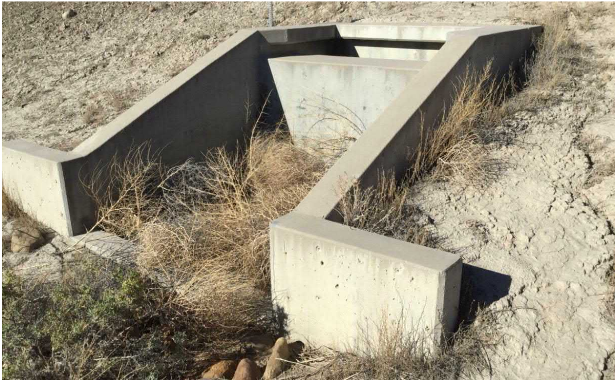
Photograph No. 23 View of energy dissipation structure at downstream end of retention pond outlet conduit, looking southwest. This facility is a zero-discharge facility and gate remains closed.
