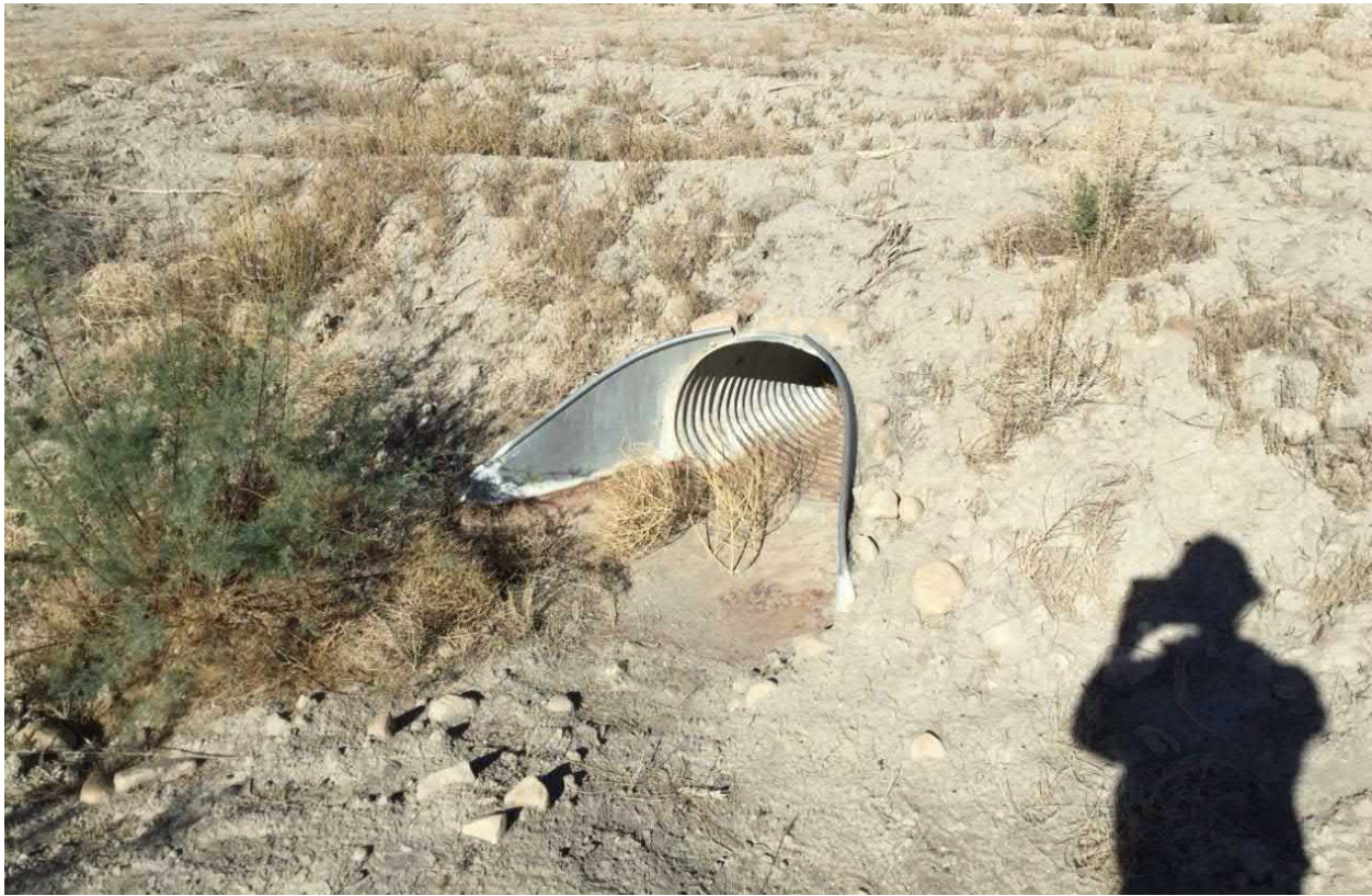
Photograph No. 15 View of south retention basin inlet pipe (upstream end). Pipe culvert was unobstructed and free of debris, looking west-northwest.
