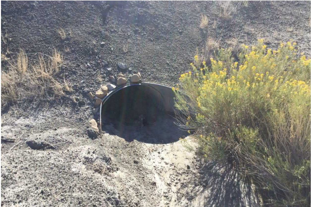
Photograph No. 29 View of retention basin north inlet pipe (upstream end), looking east. Pipe culvert was partially obstructed, but has since been cleared.
