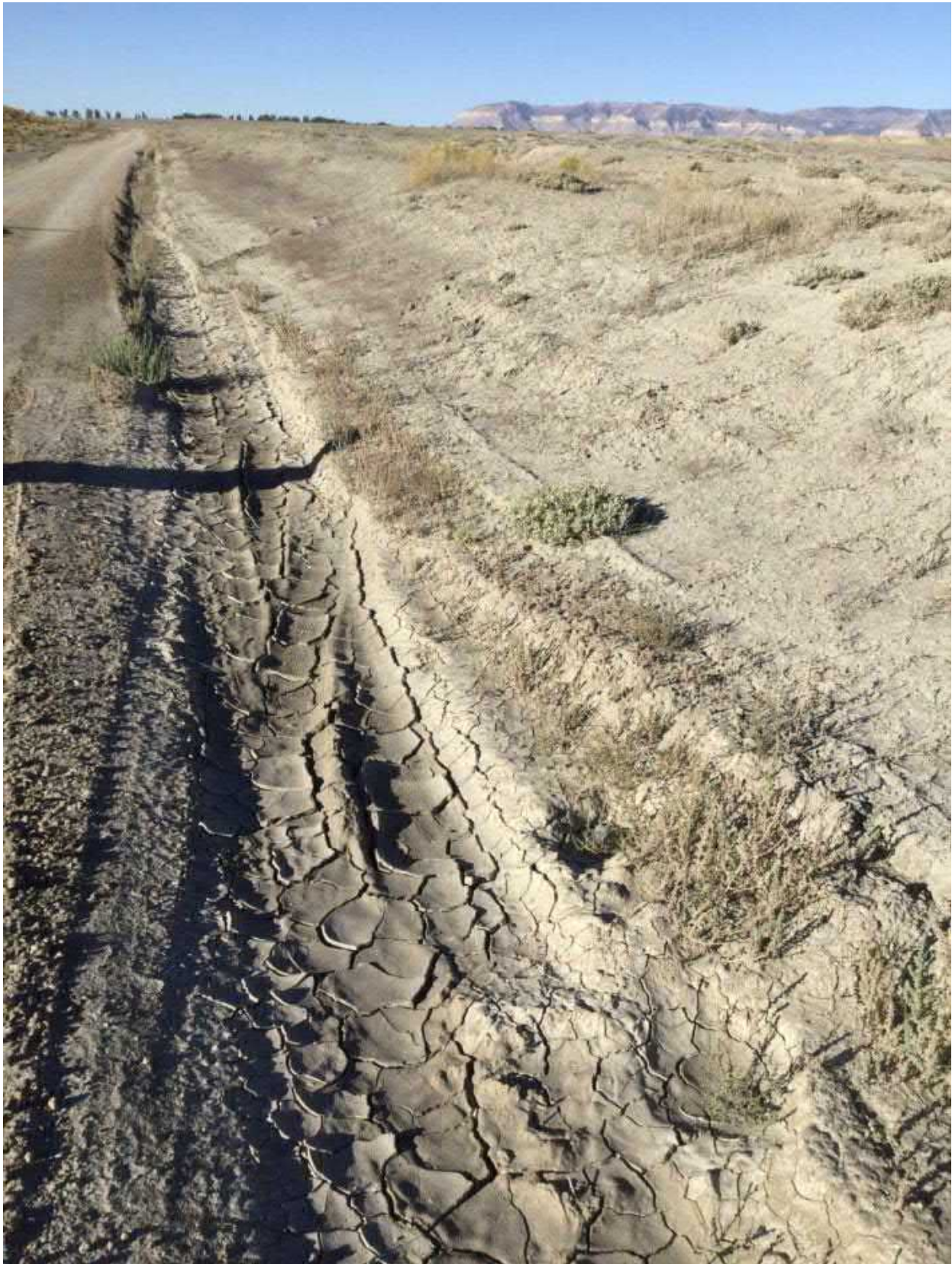
Photograph No. 1 View of depression on outside edge of perimeter road south of main haul road entrance to CCR Landfill, looking south.
