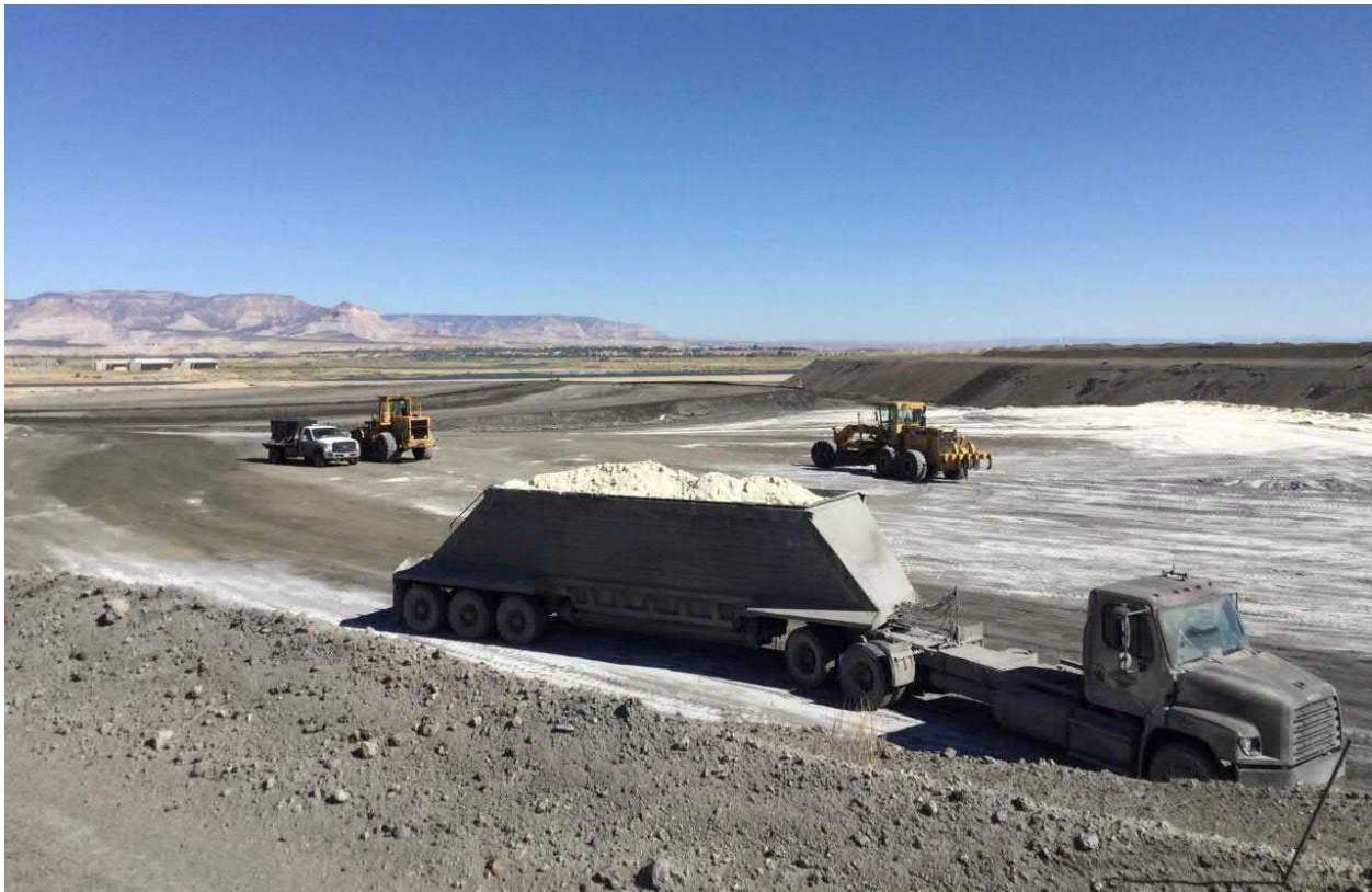
Photograph No. 32 View of recently-placed CCR material near west edge of CCR Landfill near main haul road entrance. Note FGD material placement.
