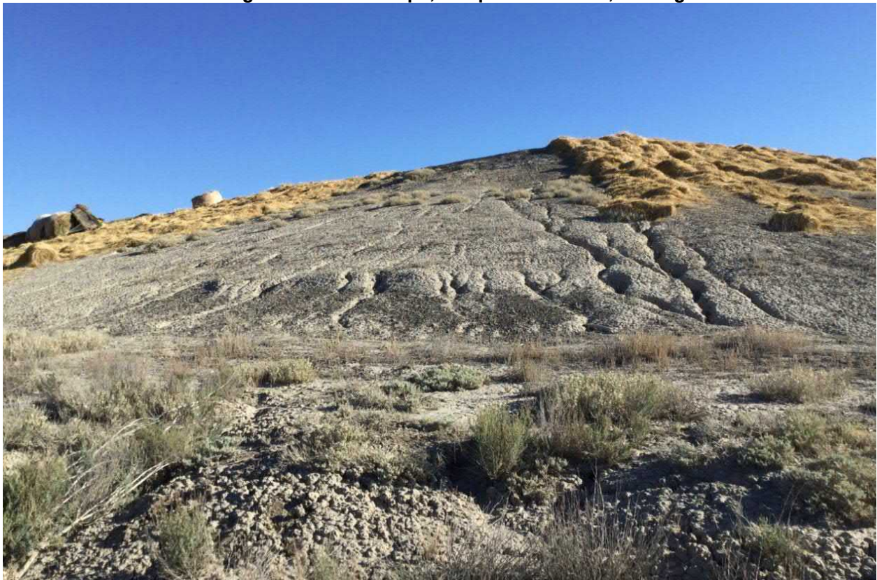
Photograph No. 10 View of southwest slope of CCR Landfill, looking northeast. Note erosion rills and hay placed on slope.
