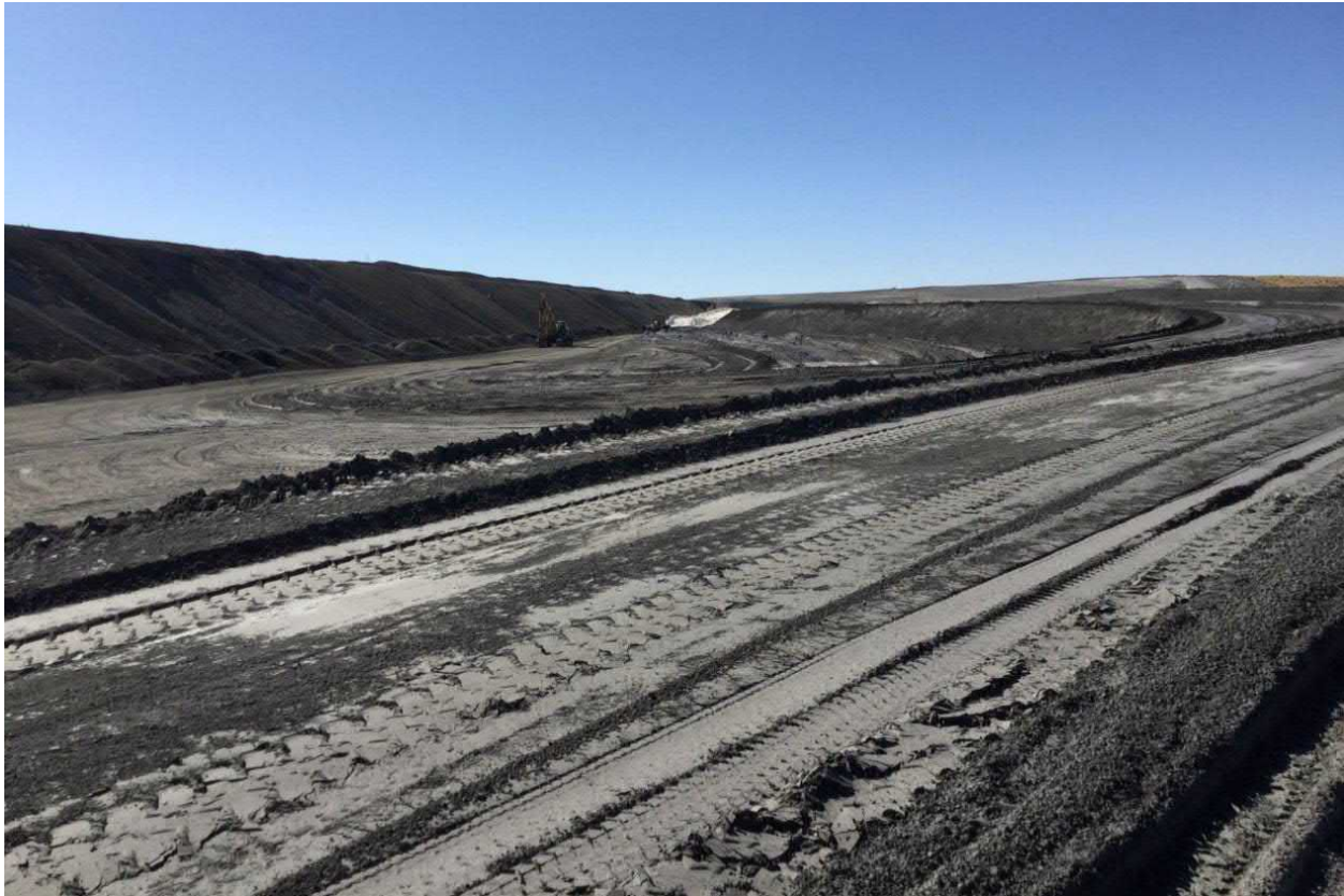
Photograph No. 31 View of recently-placed CCR material near west edge of CCR Landfill.
