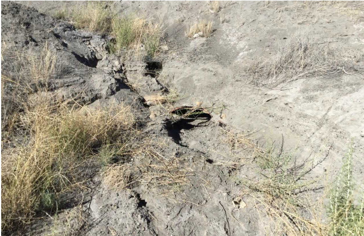
Photograph No. 28 View of erosion gully above north inlet pipe (downstream end), looking approximately south-southwest. Pipe was partially obstructed, but has since been cleared.
