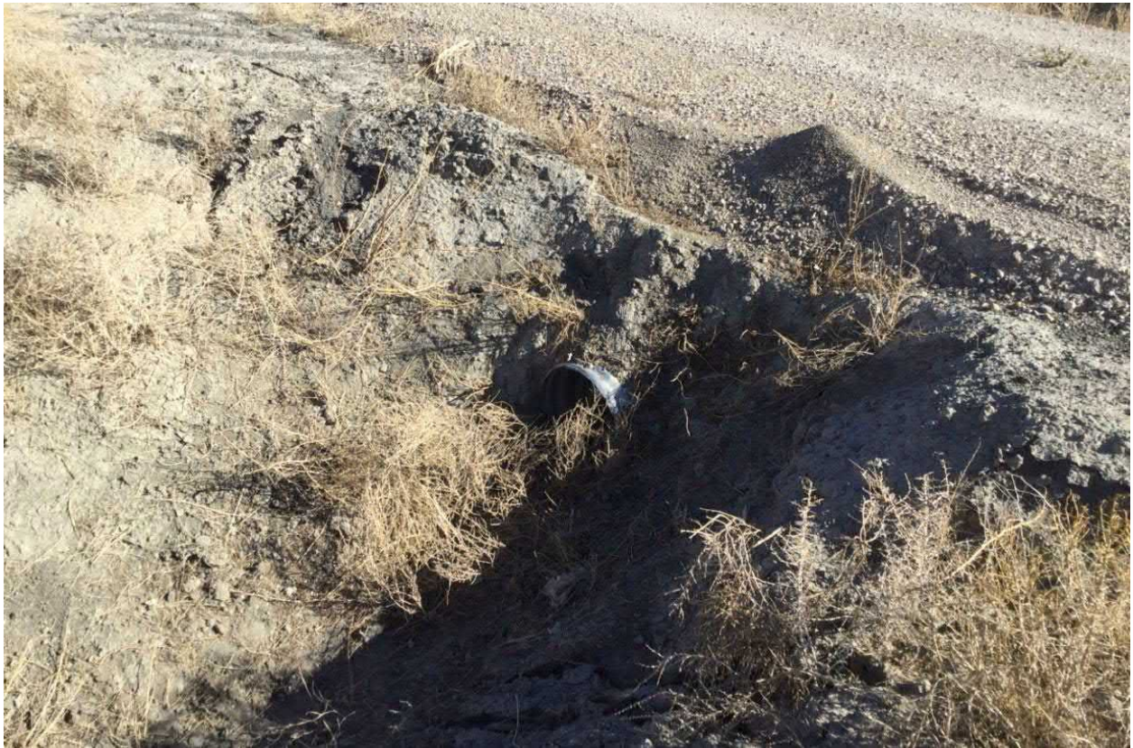
Photograph No. 17 View of pipe culvert passing under perimeter road (downstream end), looking southeast.
