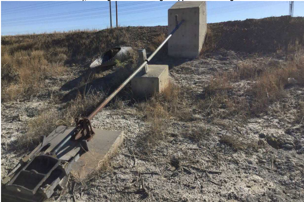
Photograph No. 22 View of slide gate control and auxiliary outlet conduit, looking east. The slide gate control appeared to be straight and in good condition.
