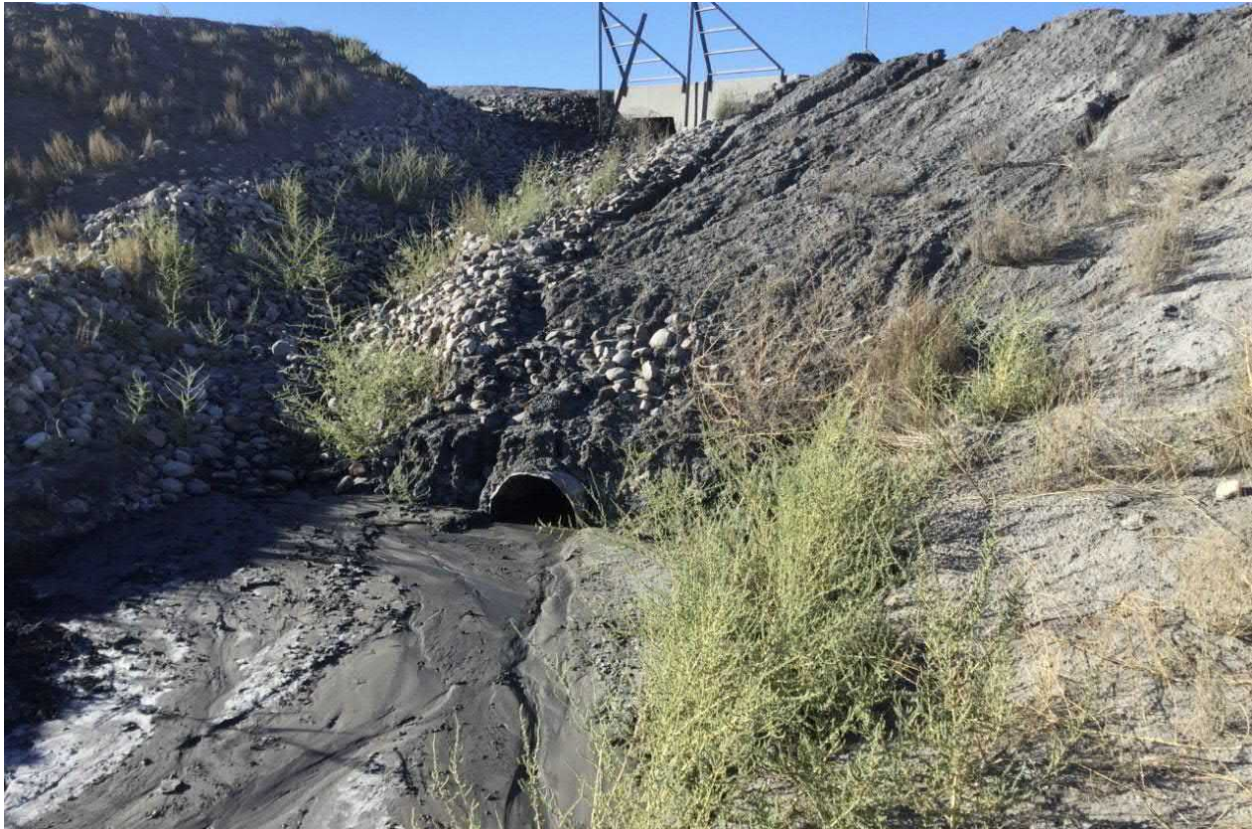
Photograph No. 33 View of pipe culvert (downstream end) under main haul road near entrance to CCR Landfill. Note rumble rack in the background. Culvert was partially obstructed by sediment, but has since been cleared.
