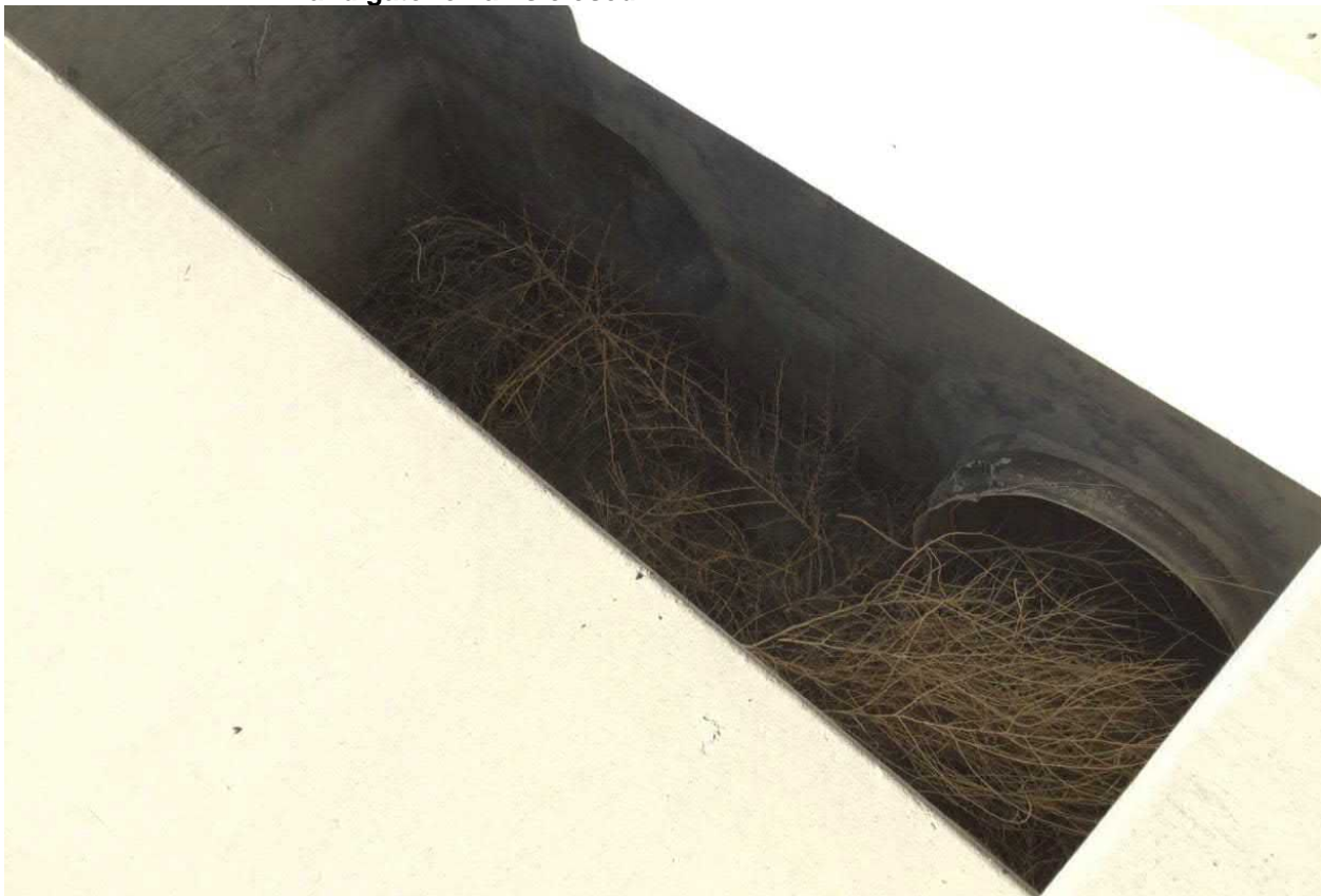
Photograph No. 24 View of energy dissipation structure at downstream end of retention pond outlet conduit and upstream of baffle. Note discharge conduit from auxiliary spillway.
