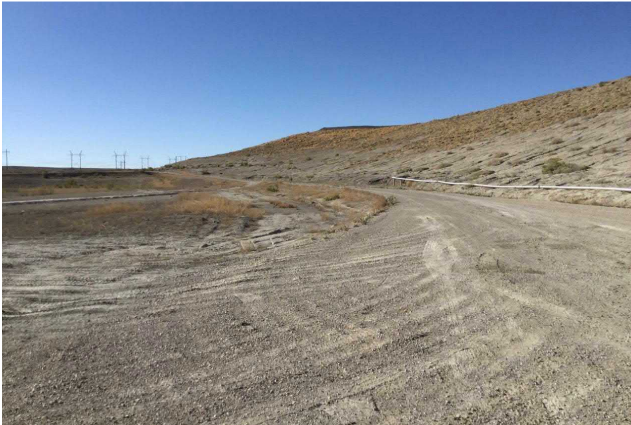
Photograph No. 19 View of east slope of CCR Landfill and drain line from underdrains to Frac tank (see Photograph No. 20), looking south.
