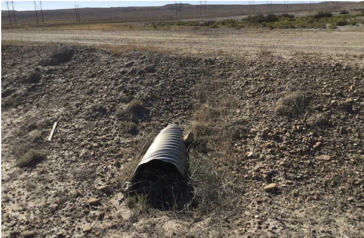
Photograph No. 26 View of pipe culvert (upstream end) under perimeter road through retention pond embankment. The purpose of the pipe is unclear, but has since been removed.
