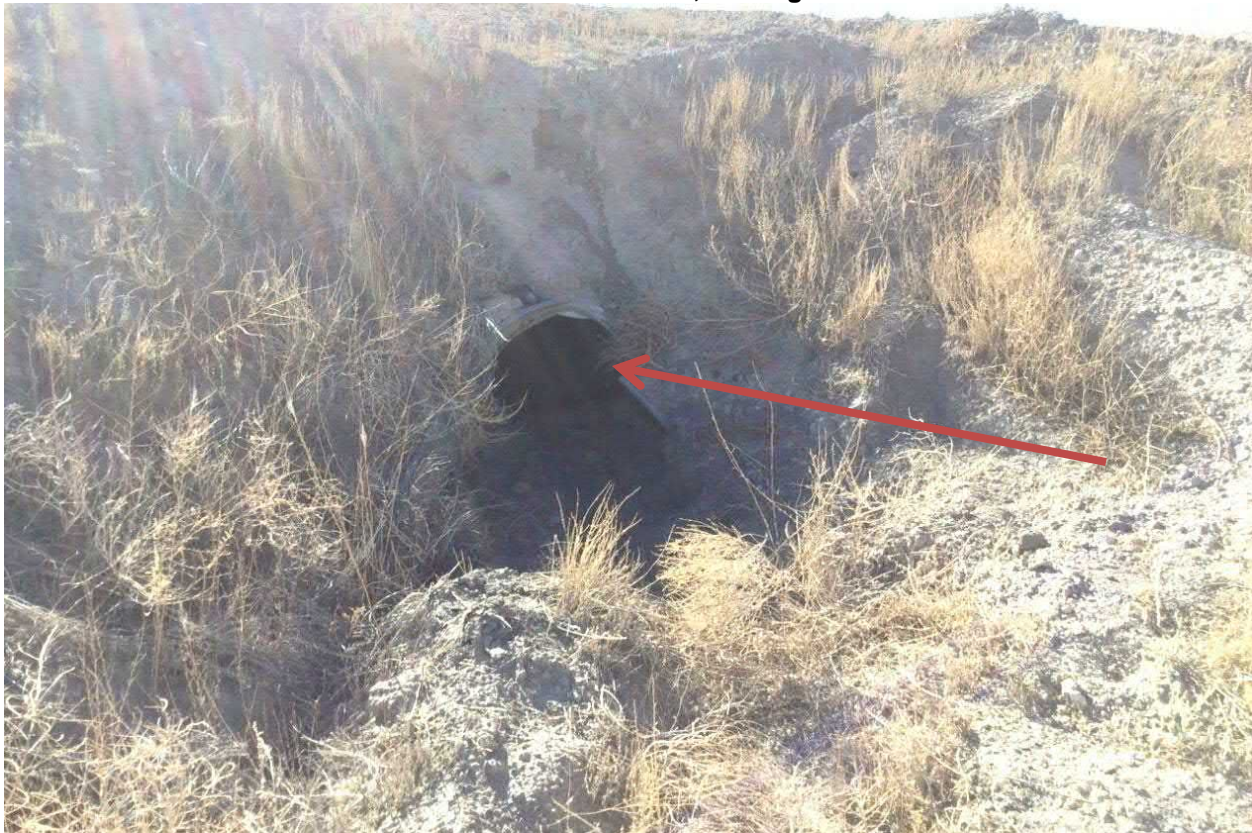
Photograph No. 16 View of south retention basin inlet pipe (downstream end). Pipe culvert was partially obstructed at this end at time of inspection, looking southeast.
