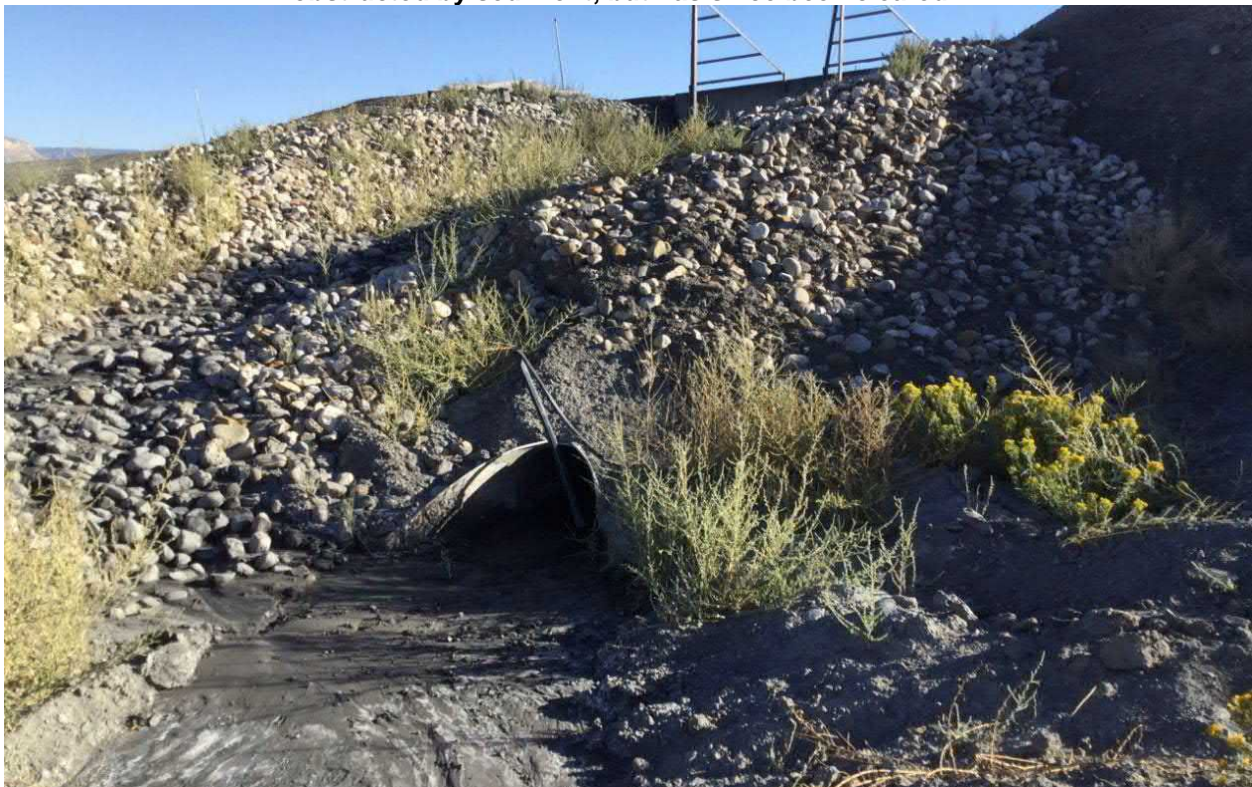
Photograph No. 34 View of pipe culvert (upstream end) under main haul road near entrance to CCR Landfill. Culvert was partially obstructed, but has since been cleared.
