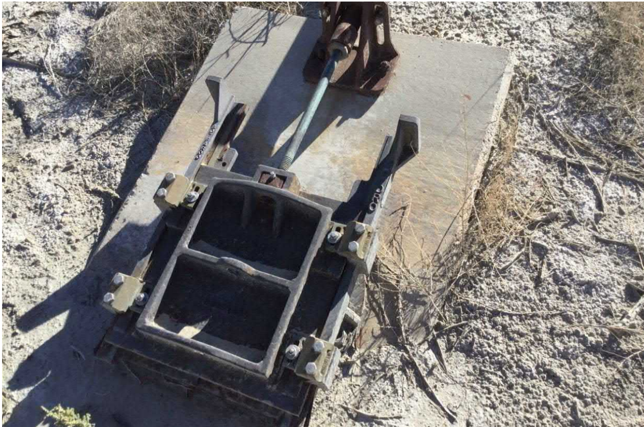
Photograph No. 21 View of retention pond outlet and slide gate control structure (upstream end), looking east. The slide gate appeared to be in good condition.
