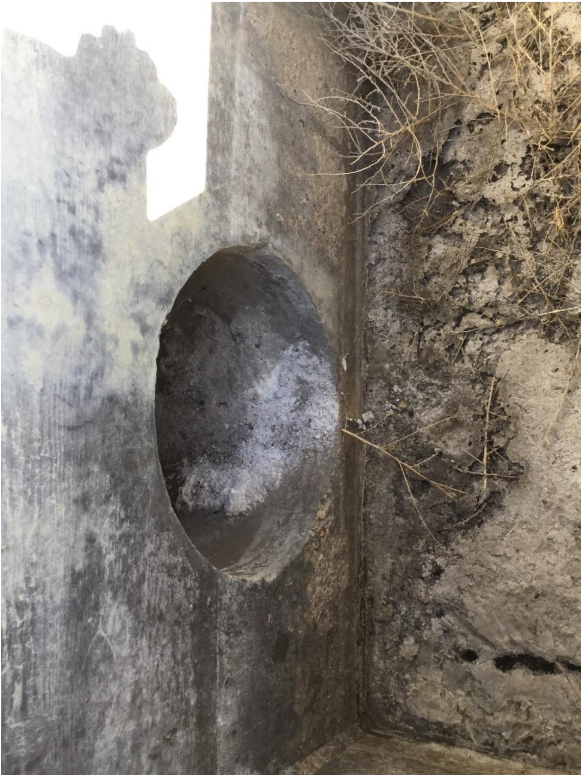
Photograph No. 26 View of energy dissipation structure at downstream end of retention pond outlet conduit and upstream of baffle. Note dry material in outlet conduit.
