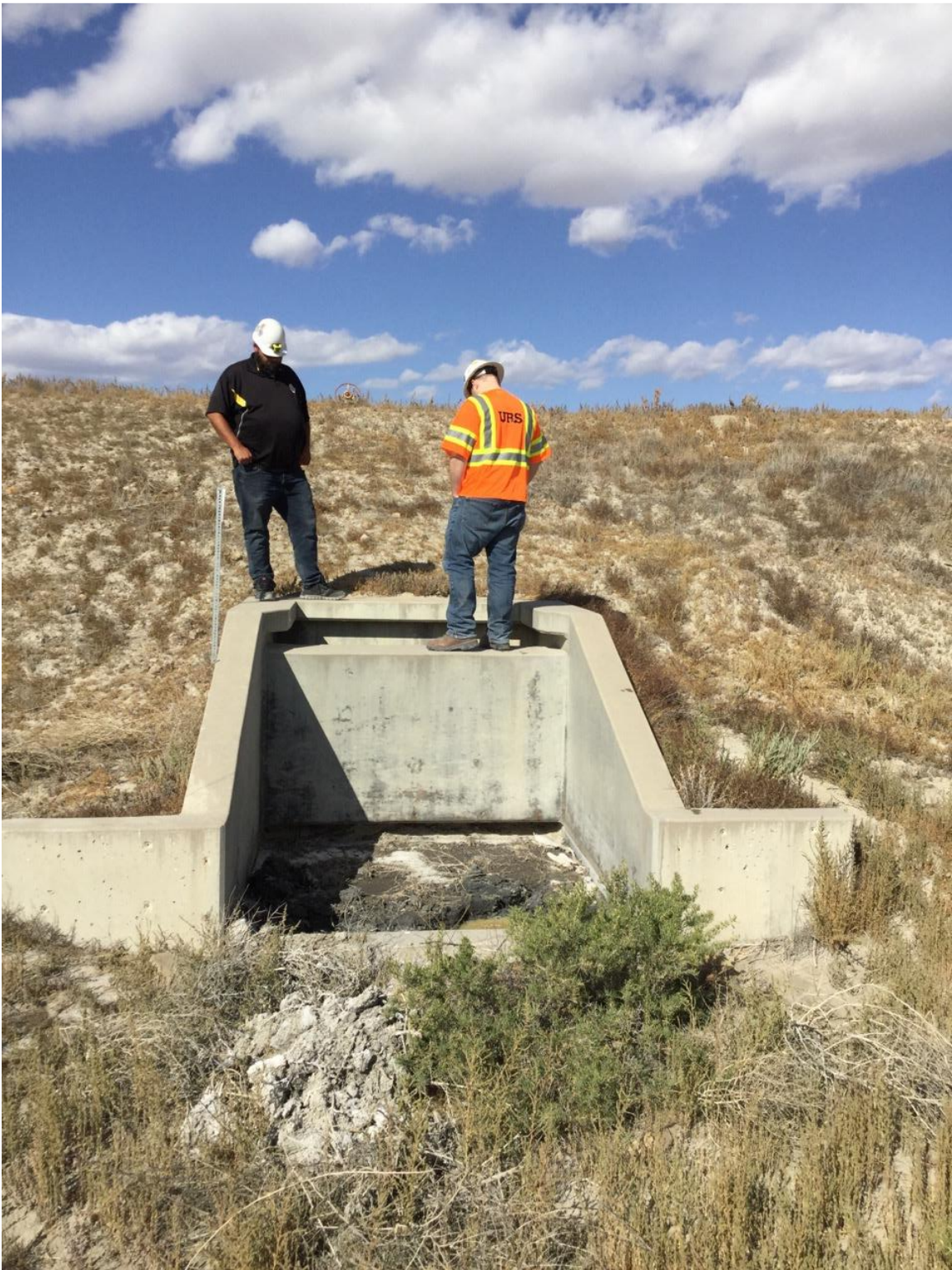
Photograph No. 23 View of energy dissipation structure at downstream end of retention pond outlet conduit, looking west. This facility is a zero-discharge facility and gate remains closed.
