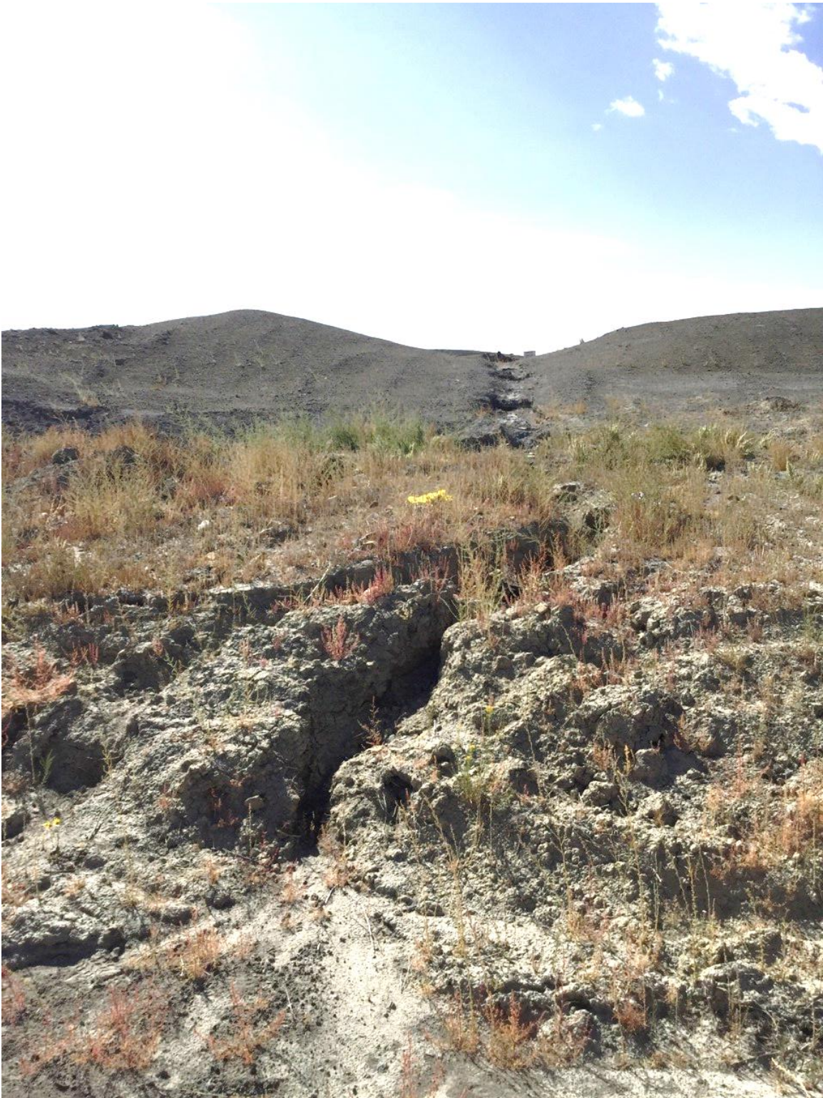
Photograph No. 29 View of erosion from snowmelt on north slope of CCR Landfill, looking southeast.
