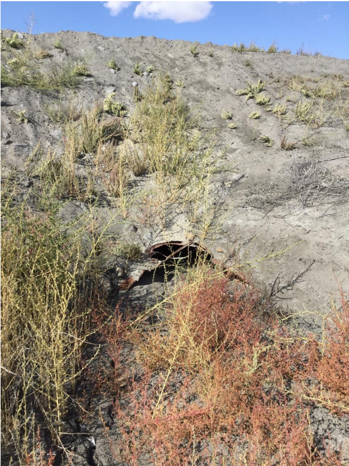
Photograph No. 27 View of north inlet pipe (downstream end), looking approximately south-southwest. Pipe was partially obstructed.
