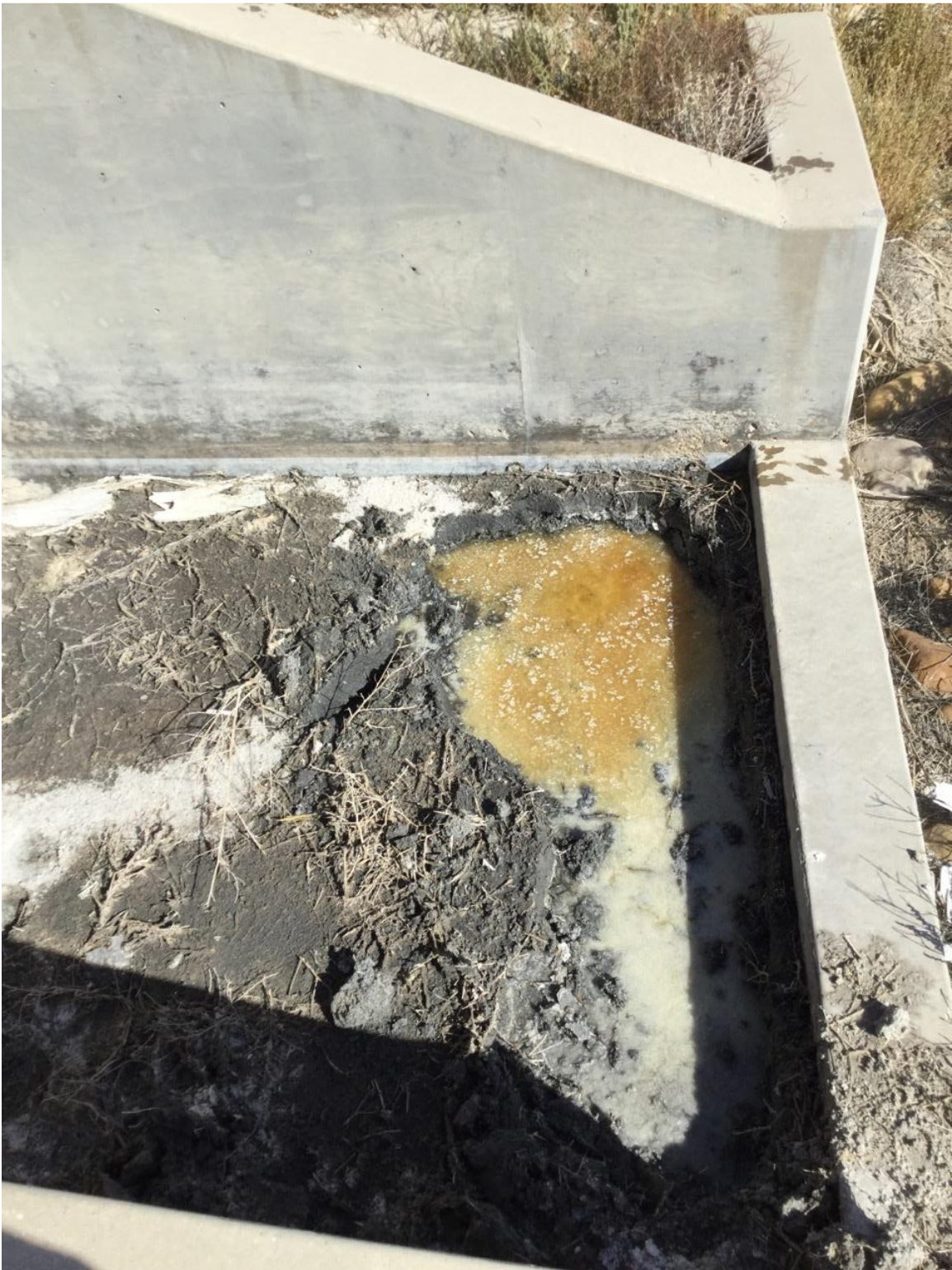
Photograph No. 24 View of energy dissipation structure at downstream end of retention pond outlet conduit and downstream of baffle. Note ponding water despite no water present at upstream end.
