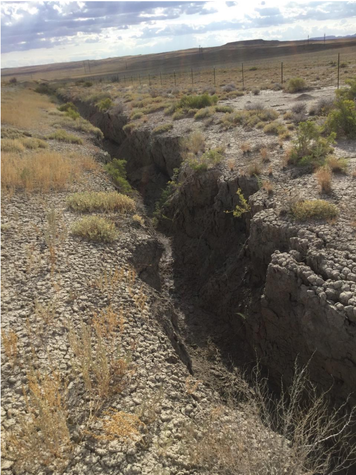
Photograph No. 11 View of offsite diversion channel around permitted CCR Landfill, looking east. Channel is approximately 6 feet deep.
