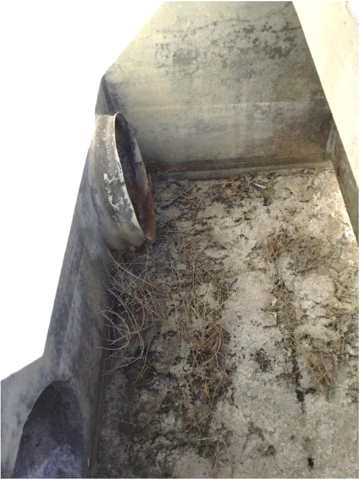
Photograph No. 25 View of energy dissipation structure at downstream end of retention pond outlet conduit and upstream of baffle. Note discharge conduit from auxiliary spillway (top).
