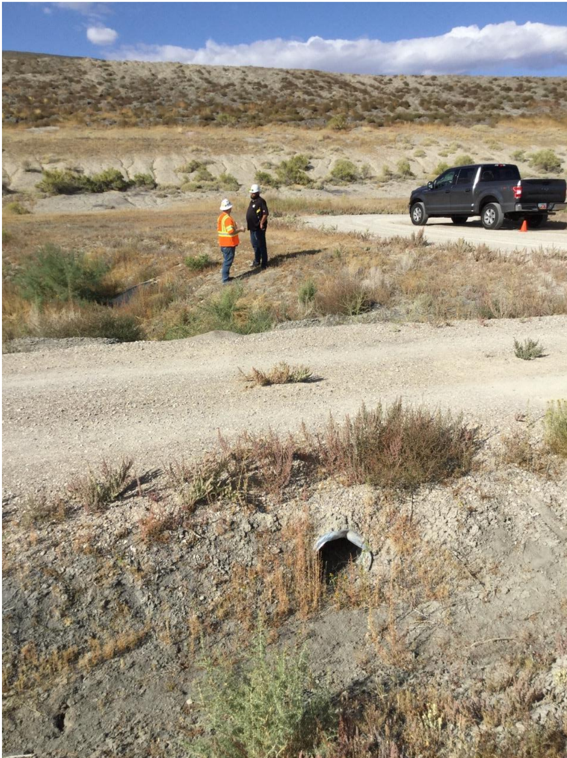
Photograph No. 17 View of pipe culvert passing under perimeter road (upstream end), looking west.
