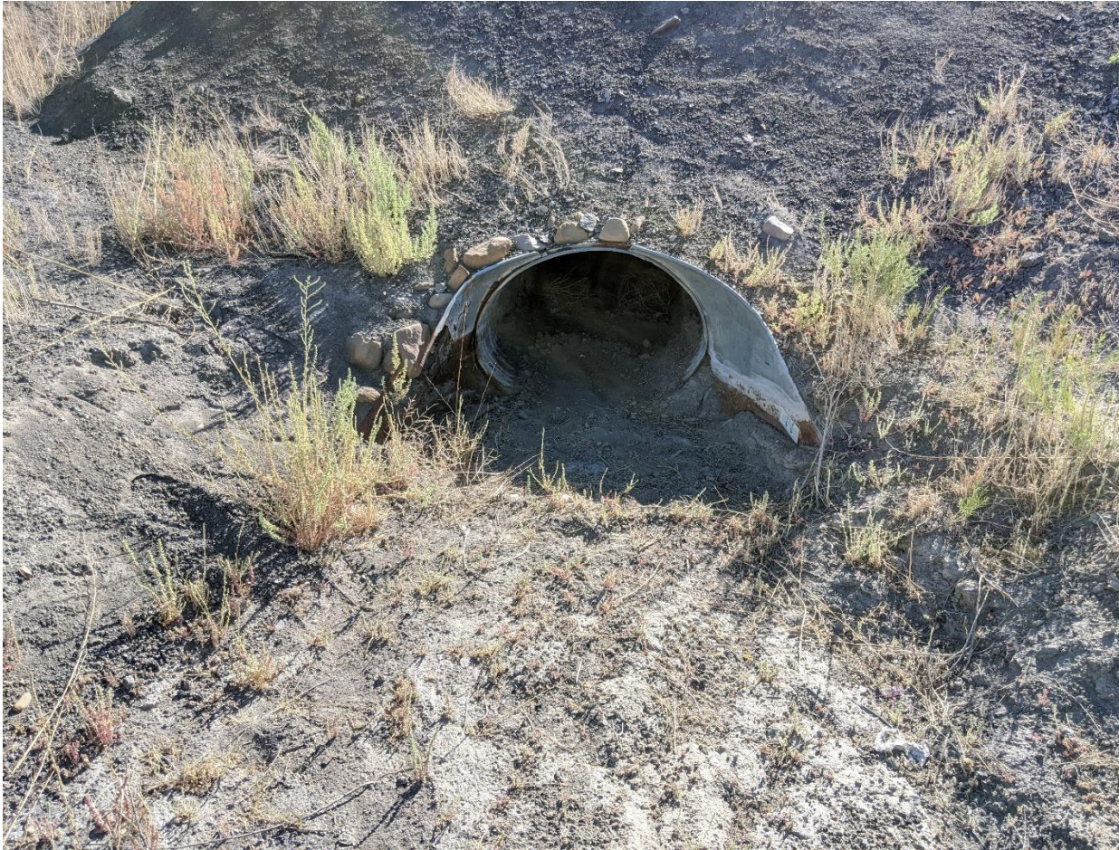
Photograph No. 25 View of upstream end of a culvert on the northern side of the CCR landfill, looking east. Note: The upstream end of the culvert appears to be mostly unobstructed.
