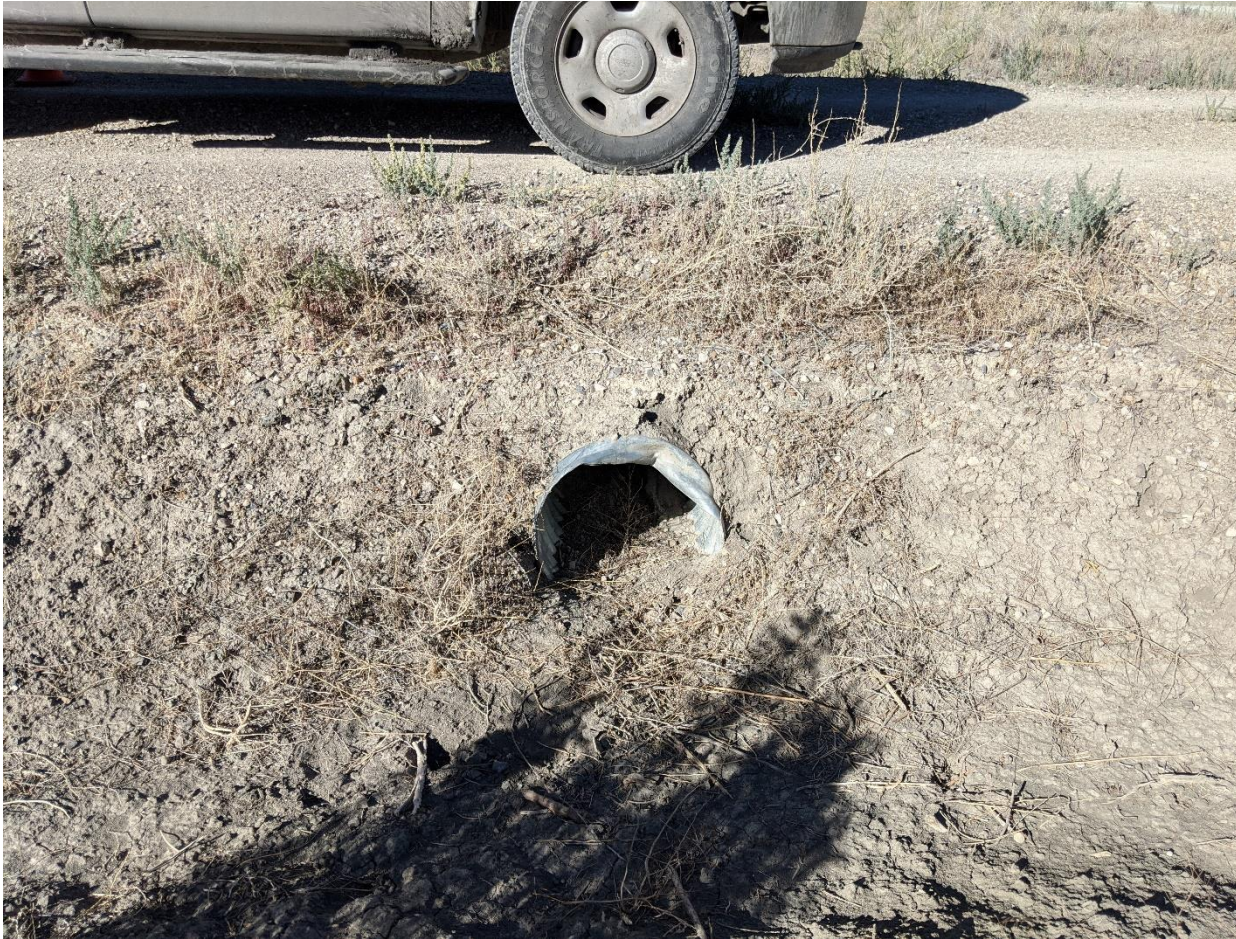
Photograph No. 15 View of upstream end of a culvert near the southern end of the retention basin, looking west. Note: The upstream end of the culvert appears to be mostly unobstructed.
