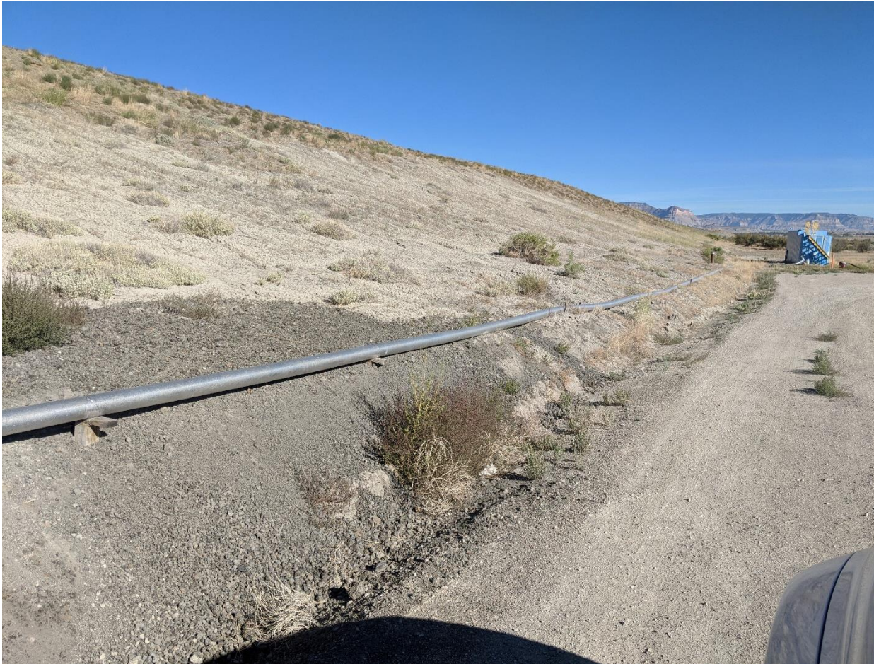
Photograph No. 19 View of dewatering collection system along east slope of CCR landfill, looking north.
