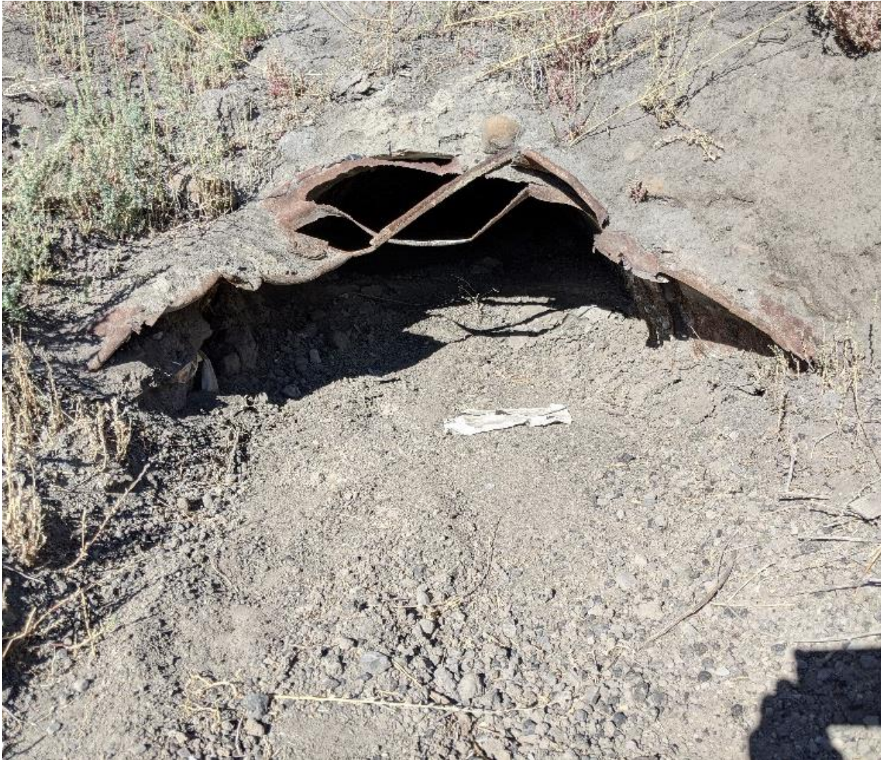
Photograph No. 24 View of downstream end of a culvert on the northern side of the CCR landfill, looking west. Note: The downstream end of the culvert appears to be partially obstructed.
