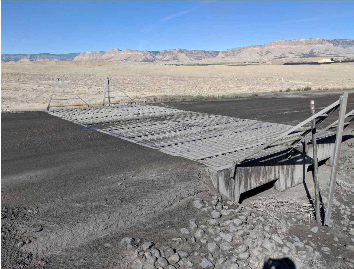
Photograph No. 28 View of main haul road and rumble rack showing dust control moisture, looking west.
