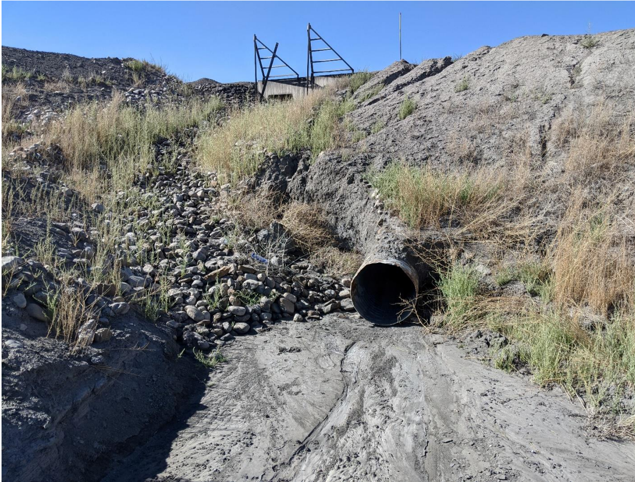
Photograph No. 1 View of downstream end of culvert under main haul road and rumble rack, looking southwest. Culvert unobstructed, but moderate erosion observed adjacent to culvert (left) from water introduced into the rumble rack from snowmelt or for dust suppression and cleanout.
