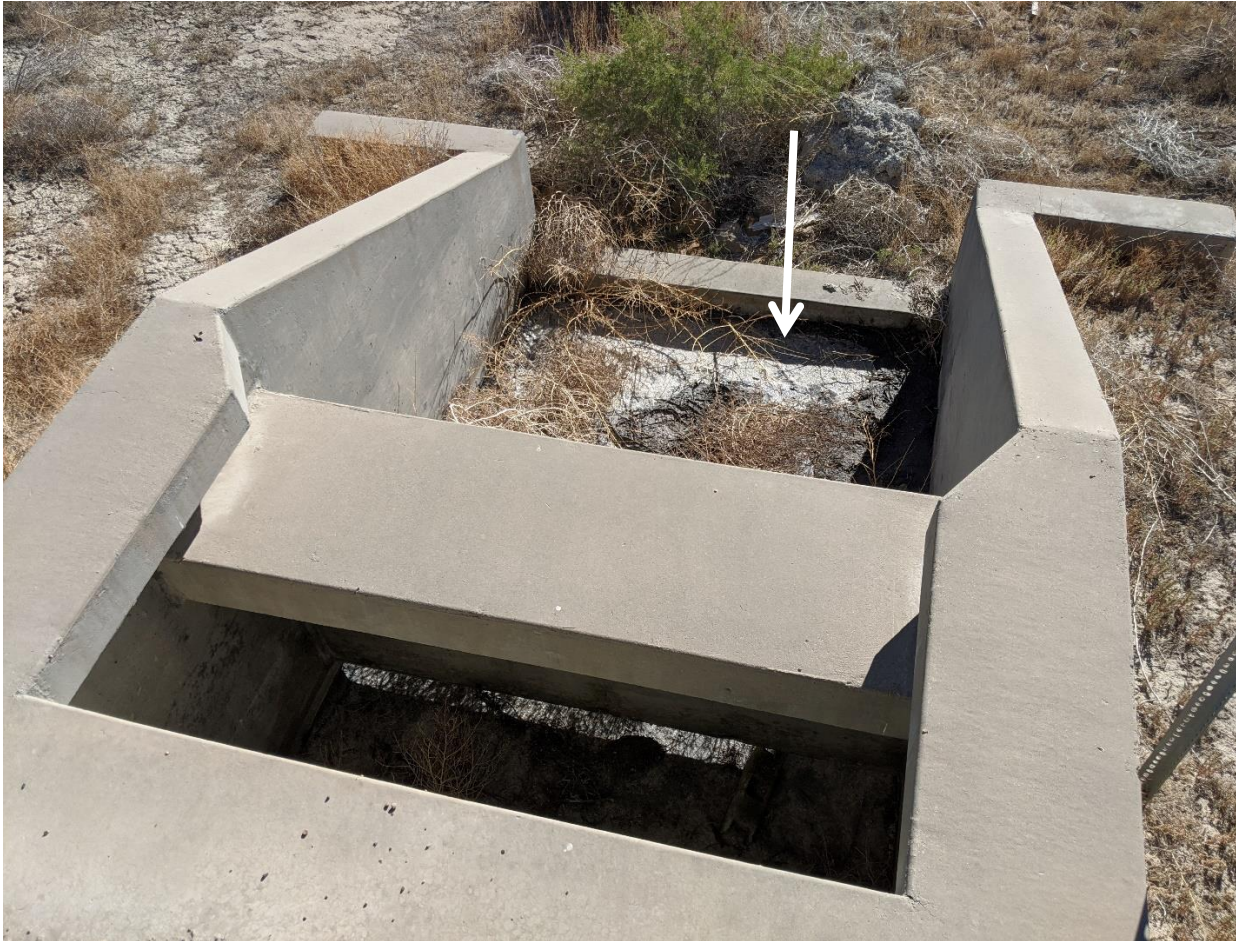
Photograph No. 22 View of retention basin stilling basin, looking east. Note salt cap and apparent moisture (arrow).
