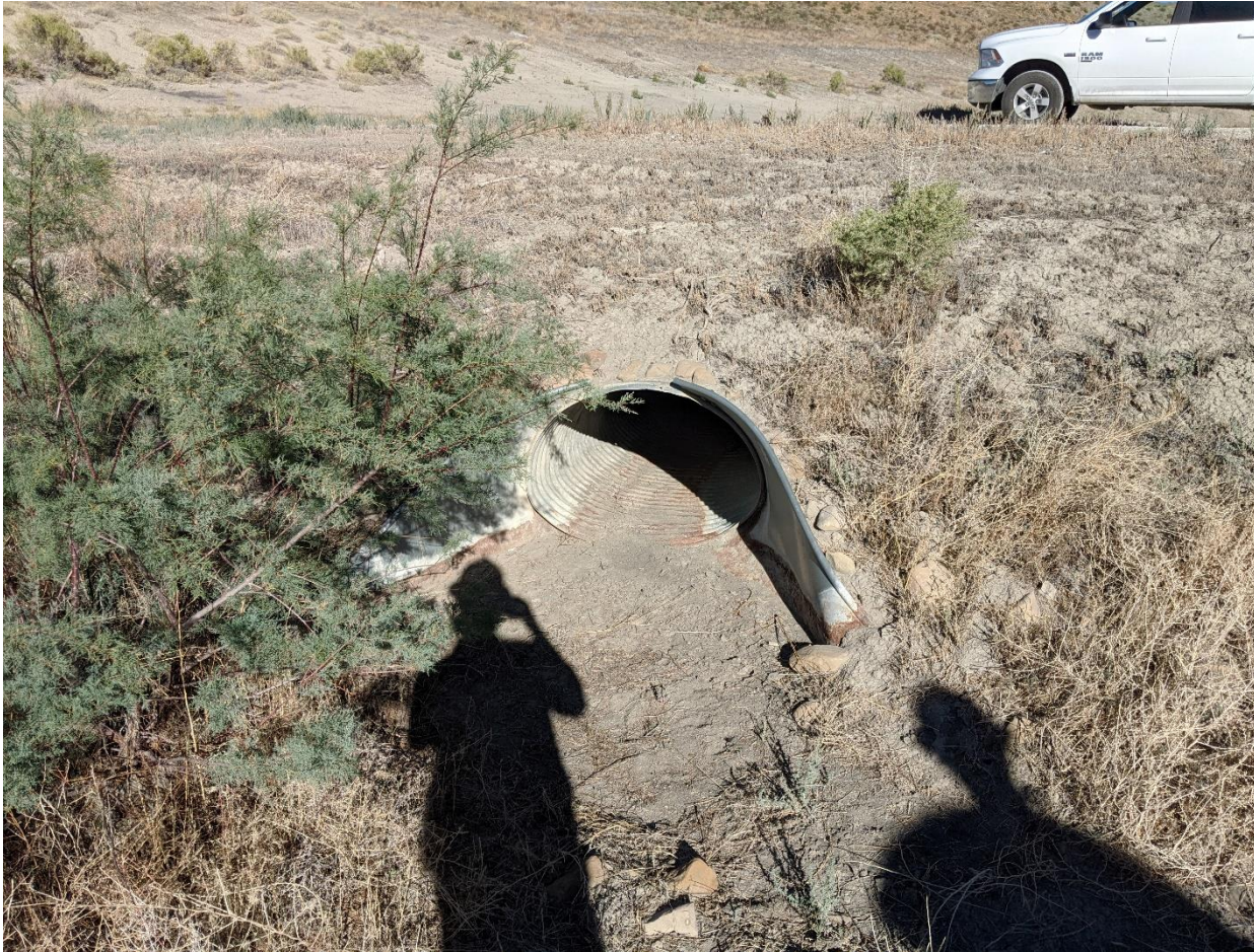
Photograph No. 17 View of upstream end of a culvert into the southern end of the retention basin, looking northwest. Note: The upstream end of the culvert appears to be mostly unobstructed.
