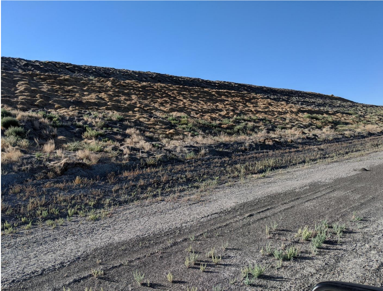
Photograph No. 3 View of western slope of CCR Landfill, looking south. Note vegetation and hay cover.
