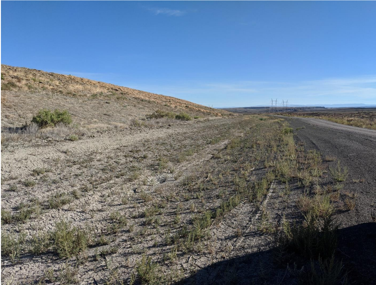
Photograph No. 13 View of southeastern slope of CCR landfill, looking northeast. Note the recent regrading and removal of brush at the toe of the slope.
