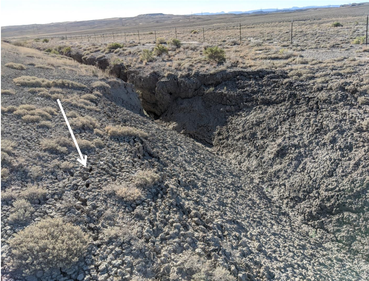
Photograph No. 8 View of erosion gully at outer slope of southwest perimeter berm, looking southeast. Note minor sloughing, desiccation, and possible tension cracking (arrow). The function and integrity of the diversion berm does not appear to be compromised at present.
