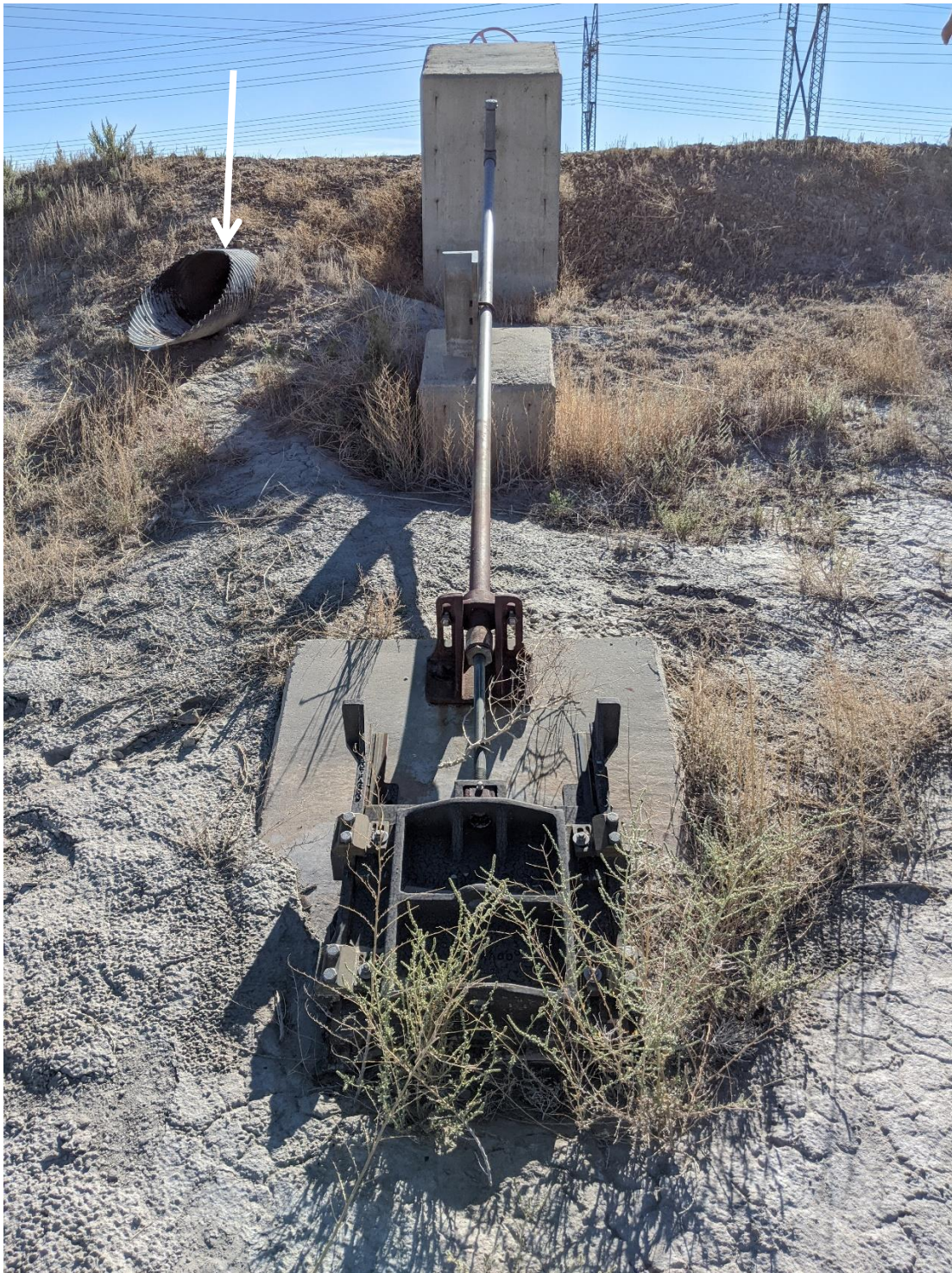
Photograph No. 21 View of retention basin outlet slide gate and overflow conduit (arrow), looking east.
