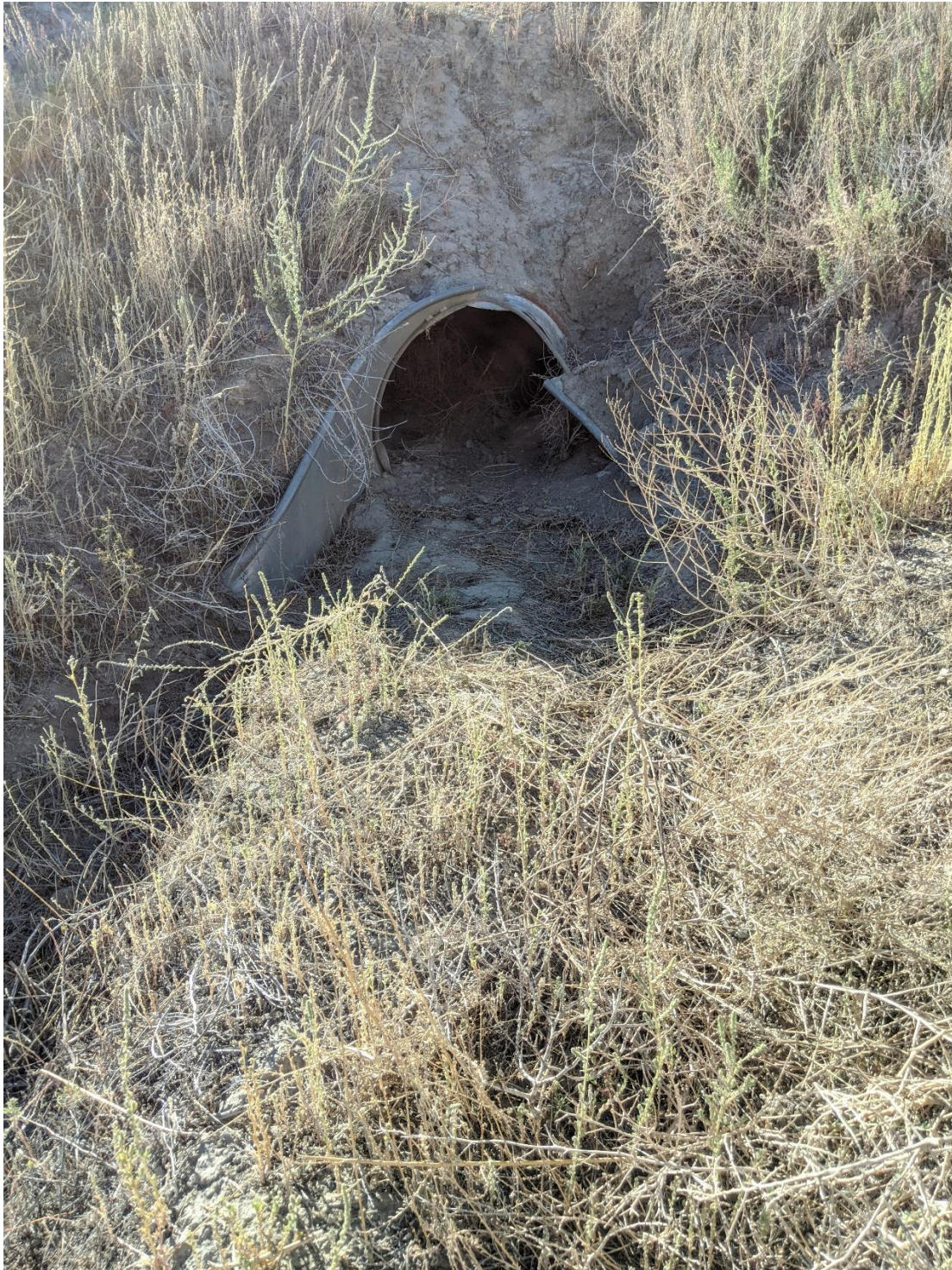
Photograph No. 18 View of downstream end of a culvert into the southern end of the retention basin, looking southeast. Note: The downstream end of the culvert appears to be mostly unobstructed.
