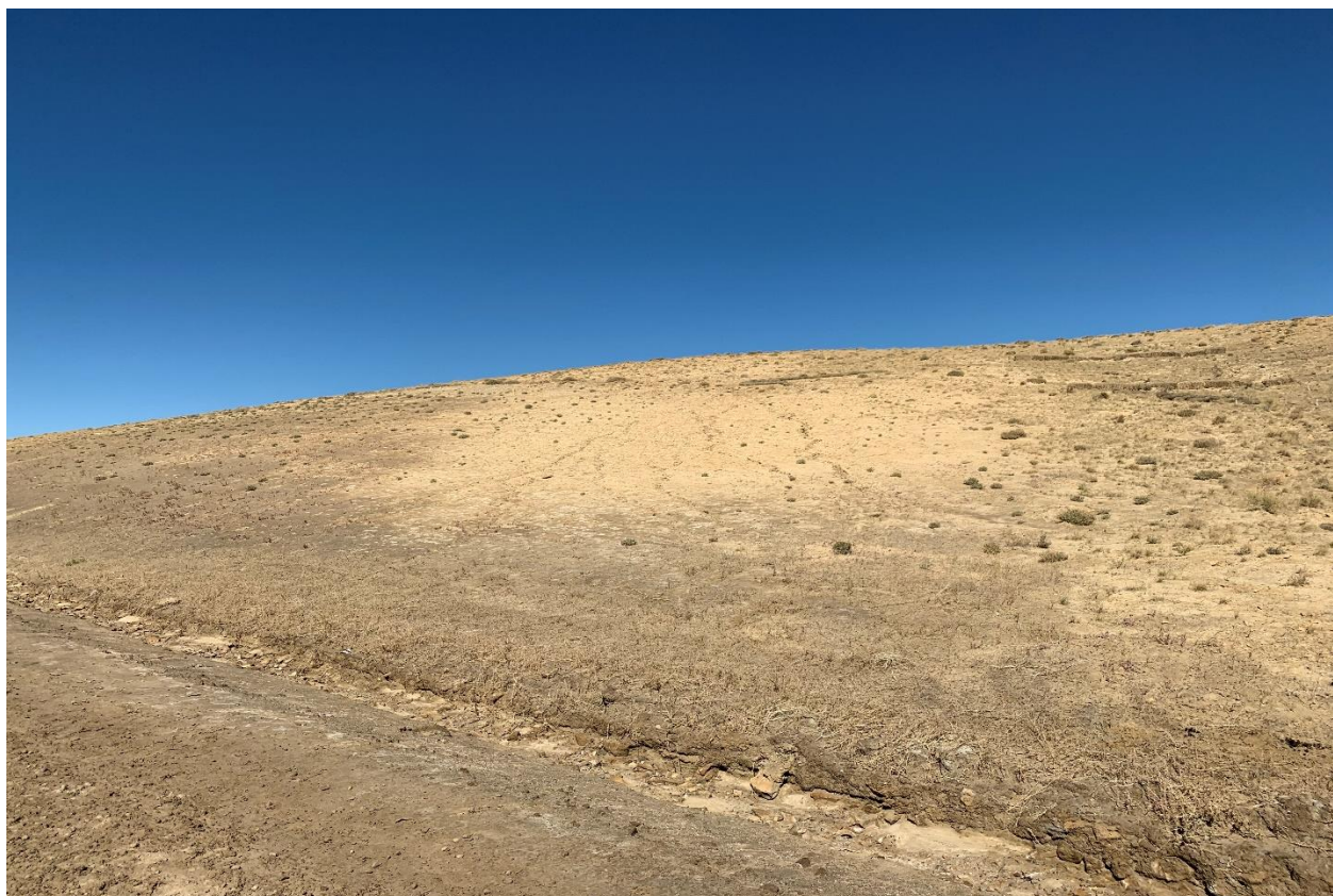
Photograph No. 2 View of minor erosional features of existing cap.
