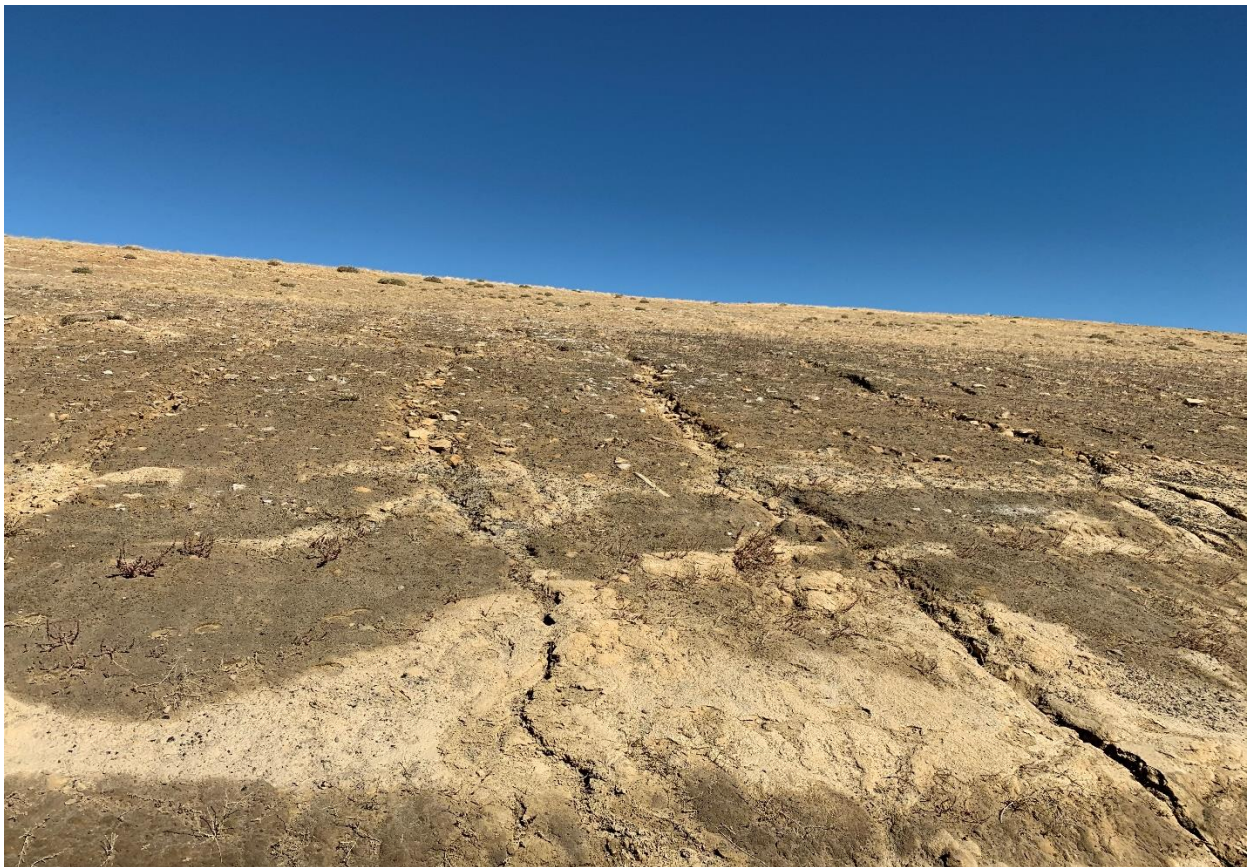
Photograph No. 4 View of minor erosional rill of existing cap.
