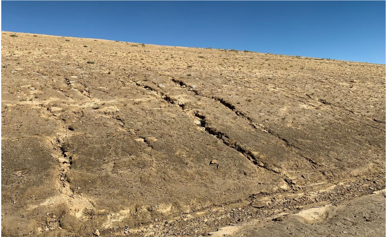
Photograph No. 3 View of minor erosional rill of existing cap.
