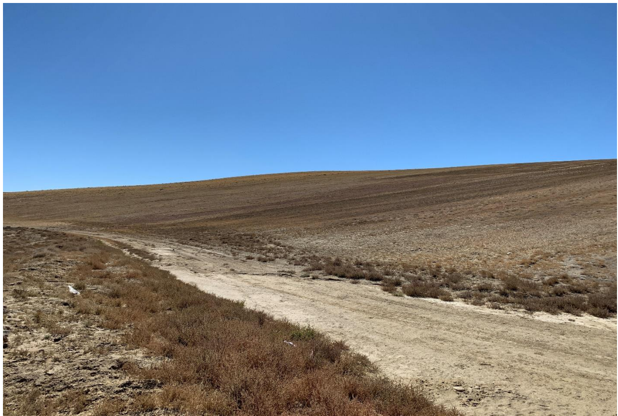
Photograph No. 10 View of final cap and sparse vegetation on eastern slope of landfill.
