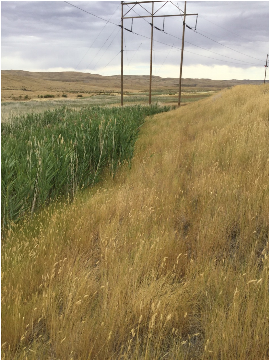
Photograph No.14 View of downstream slope of east embankment looking southeast. The vegetation appears to be approximately the same as 2017.
