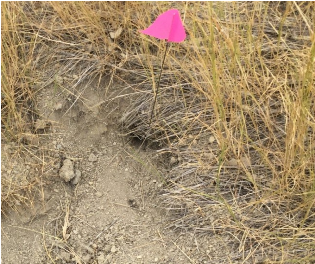
Photograph No. 11 Rodent hole on east embankment.
