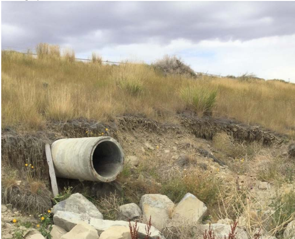
Photograph No. 6 Erosion around outlet.
