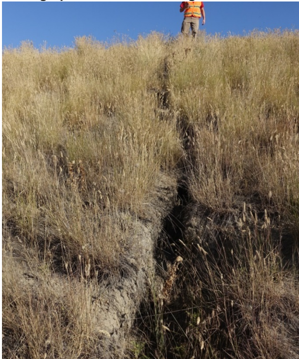
Photograph No. 2 Erosion gully on southeast embankment of North Ash Pond. Right photo is 2019. Compared to 2017 photo (left). It shows that this is nearly filled in with vegetation in 2019.
