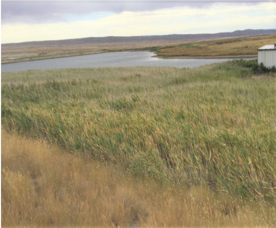
Photograph No. 1 View of vegetation on downstream toe of southeast embankment.
