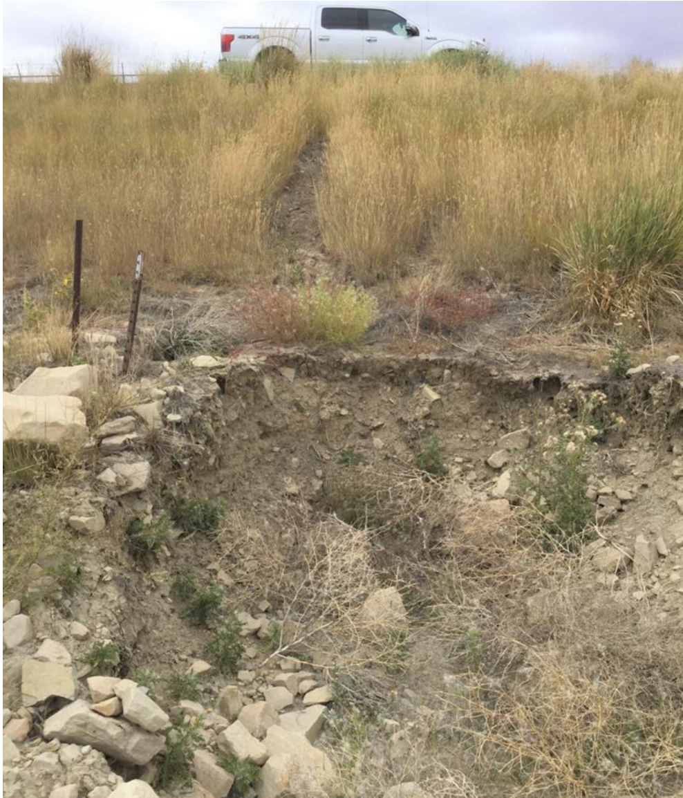
Photograph No. 7 Erosion from prior pump discharge. No on-going pumping.
