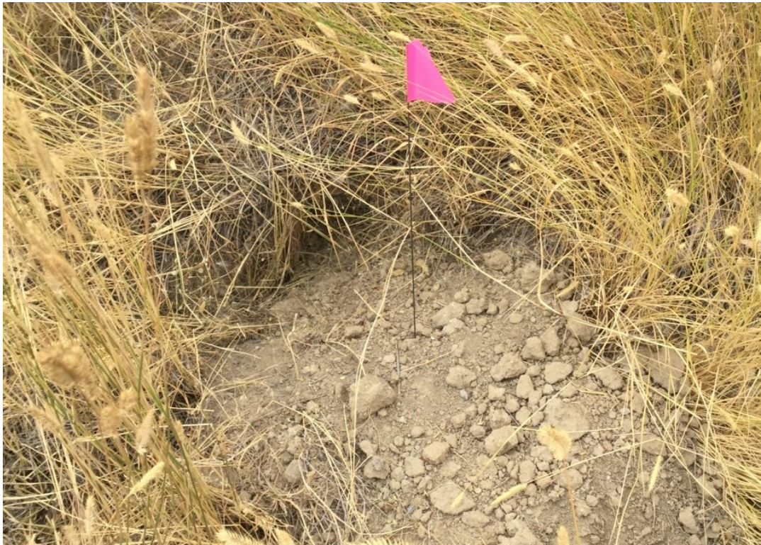
Photograph No. 12 Second rodent hole on east embankment.
