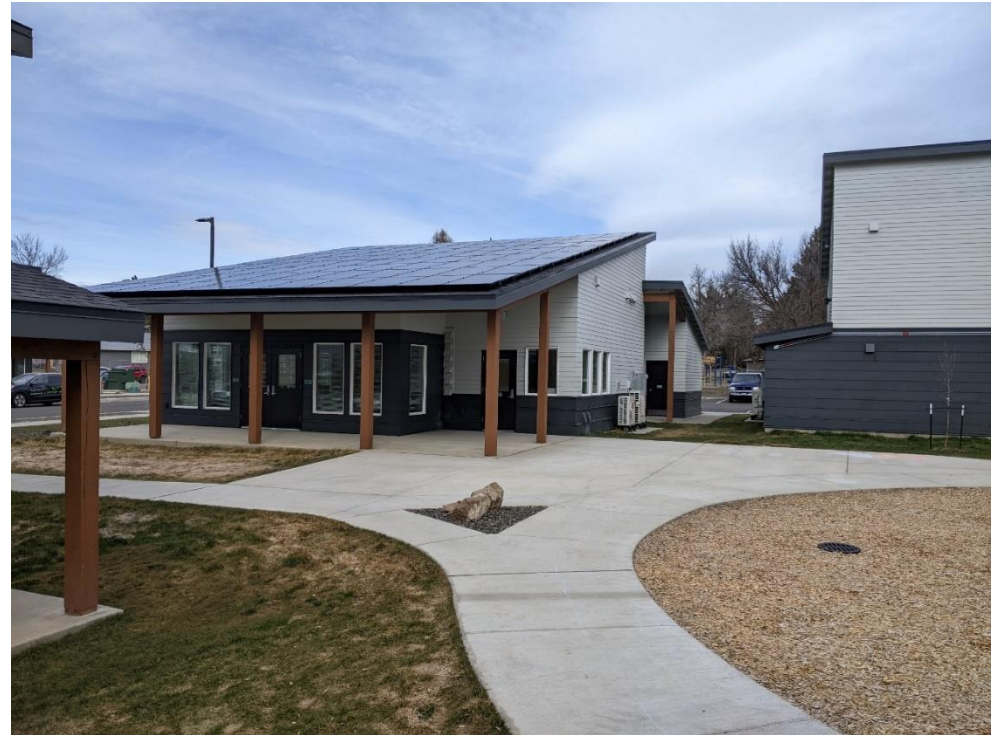
Commerce clean energy grant project – HopeSource, Ellensburg
