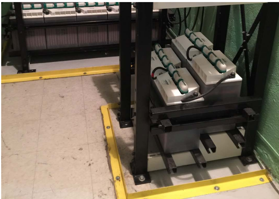
Photo 3. Battery bank with secondary containment in Ashton Powerhouse.
