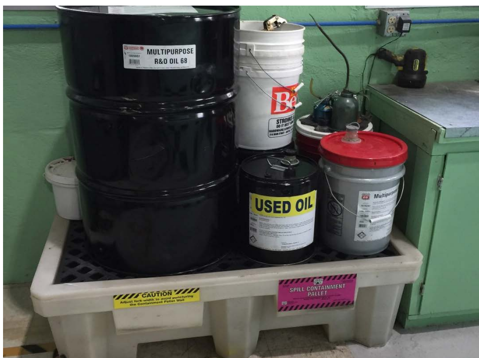
Photo 4. Hazardous materials with secondary containment system in Ashton Powerhouse.
