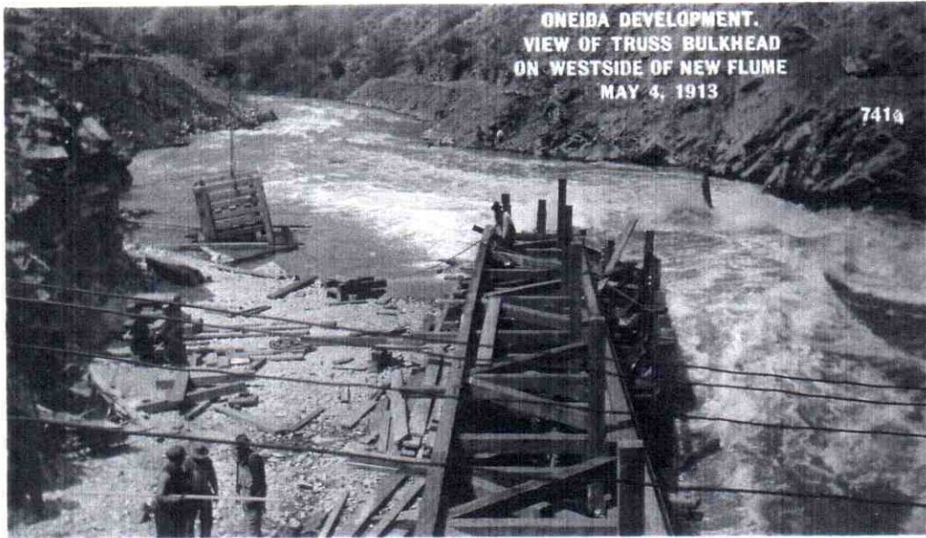
ONEIDA DEVELOPMENT. VIEW OF WOODEN CRIBS FOR FLUME MAY 4, 1913
