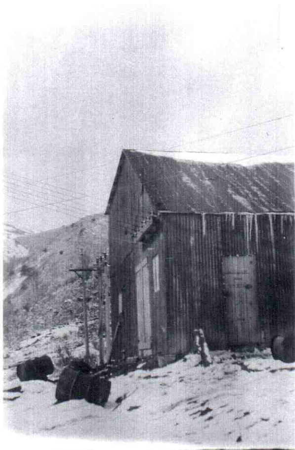
5364-Oneida-High voltage Transformer House - 3/14/12
