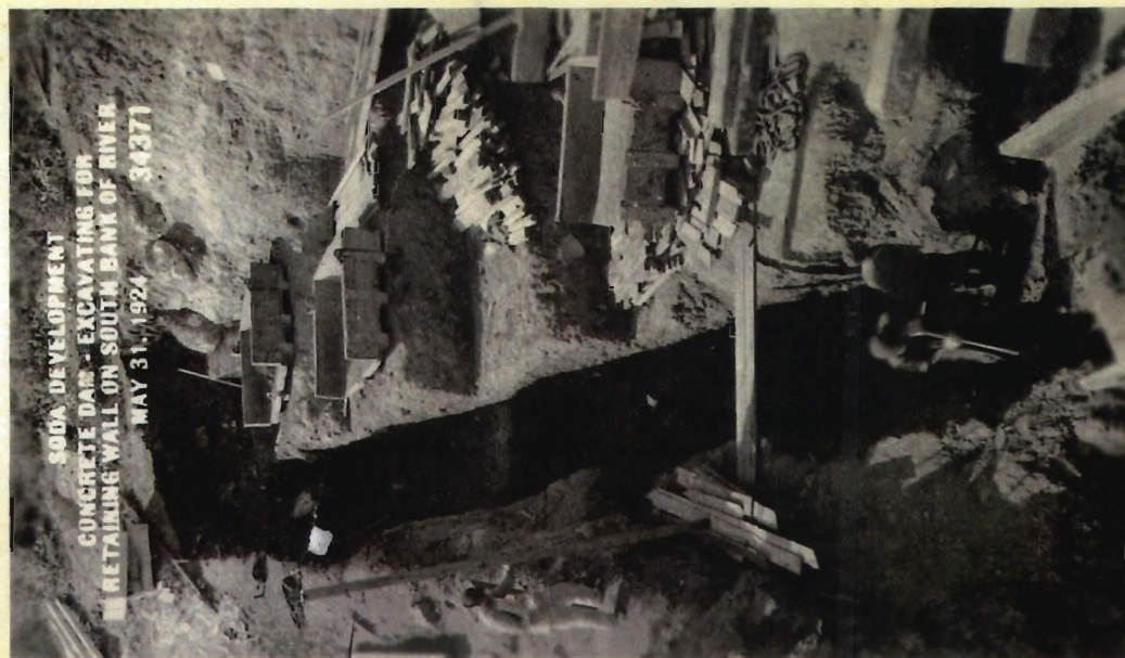
SODA DEVELOPMENT CONCRETE DAM - EXCAVATING FOR UPSTREAM RETAINING WALL ON SOUTH BANK OF RIVER JUNE 2, 1924 34372
