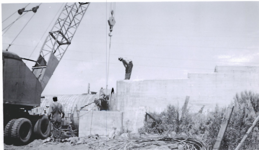
Lifting butterfly valve from old location.
