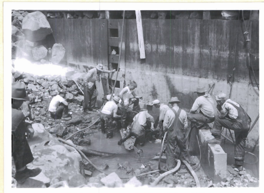
5-17-50 39/08 #72 Closing sluice gate on downstream face of dam. View northwesterly.
