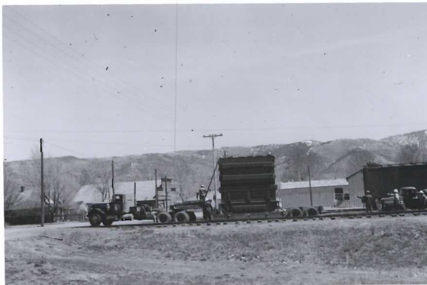
#2 - 132-161 Kv auto transformer loaded on transport ready to leave railroad yard at Grace, Idaho 12:50 P.M. Left yard 12:52 P.M. 5-10-55
