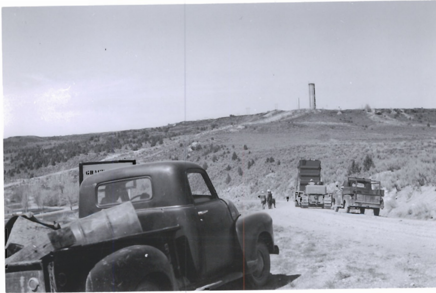
#5 - 132-161 Kv auto transformer starting down dugway with A.C.H.D.15 in rear as safety hold-back. Speed down dugway about 100 ft. per minute.
