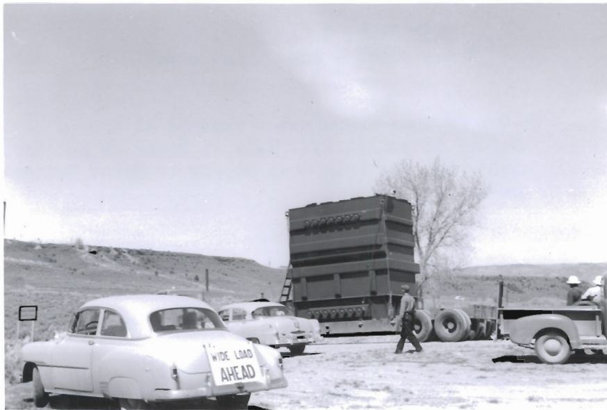
#3 - 132-161 Kv auto transformer stopped at top of dugway to attach A.C.H.D. 15 Dozer as safety hold-back for trip down dugway to Grace Switchyard. 5-10-55
