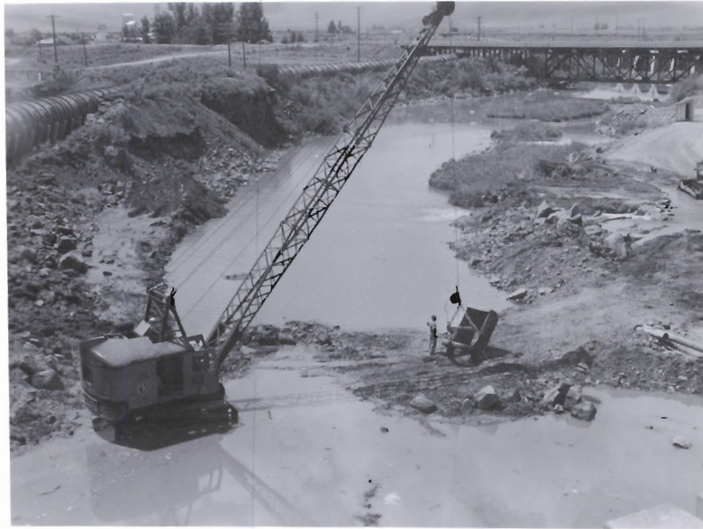
7-26-50 3/953 #119 Shows downstream channel excavation in progress.
