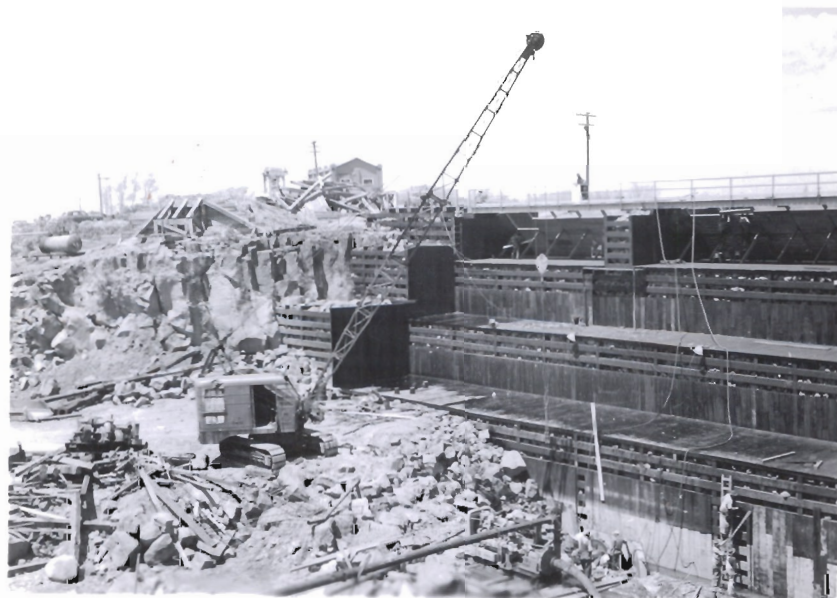
5-17-50 39110 #74 General view shows dam nearing completion. Sluice gate being bolted in place- lower right.
