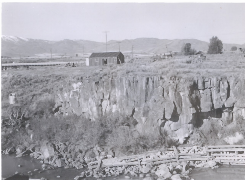
General view of west abutment area. White line indicates originally intended upstream face. Utah Construction Co. compressor house and tool shed in upper center.
