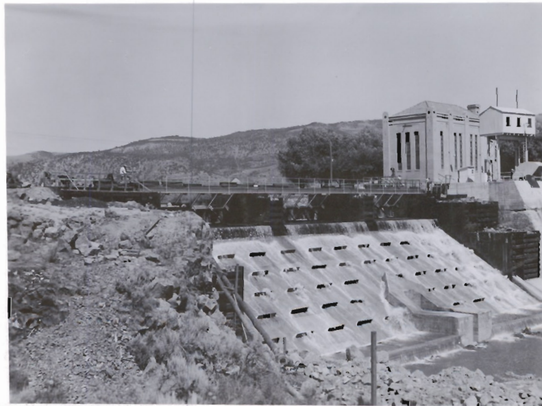
7-29-50 39157 #119-A View northeast of completed dam. Water just beginning to spill due to gates closed on pipes preparatory to taking No.2 flowline out for reconstruction.
