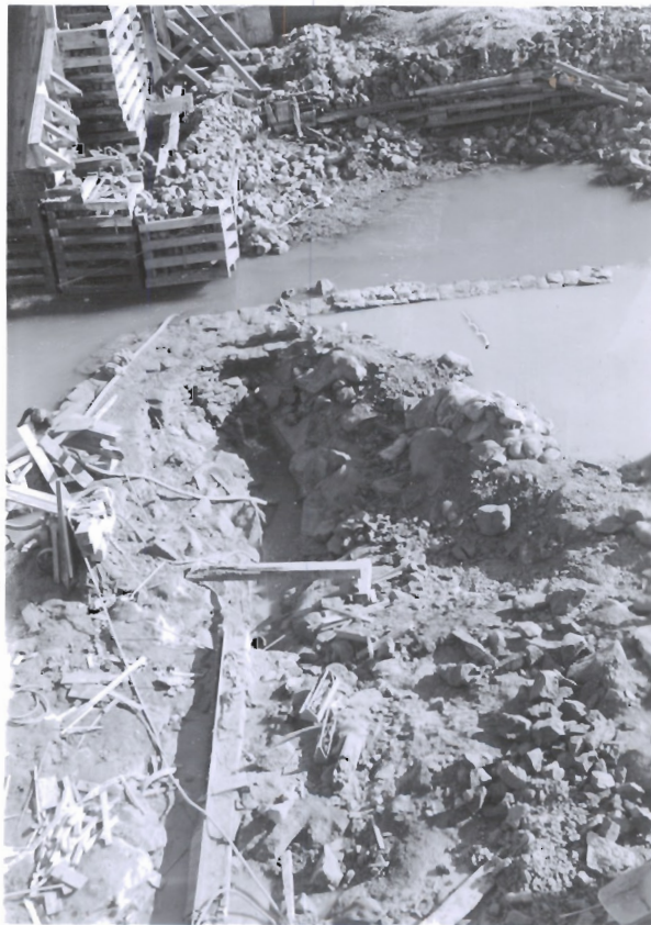
11-18-49 39059 #28 Shows finished excavation for cutoff wall to sta. 1+15 with end of poured wall to sta. 0+80. View east.
