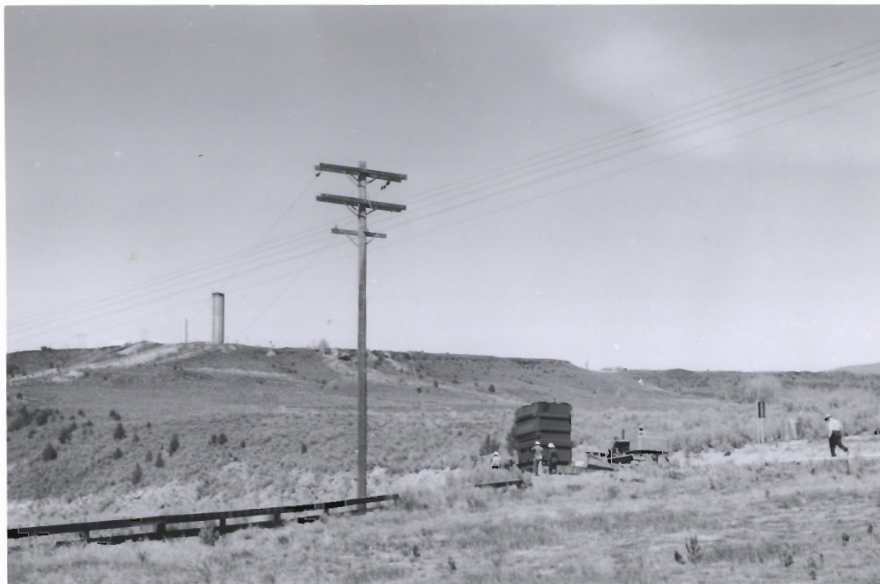
#4 - 132-161 auto transformer starting down dugway with A.C.H.D. 15 in rear as safety hold-back. Speed down dugway about 100 ft. per minute. 5-10-55
