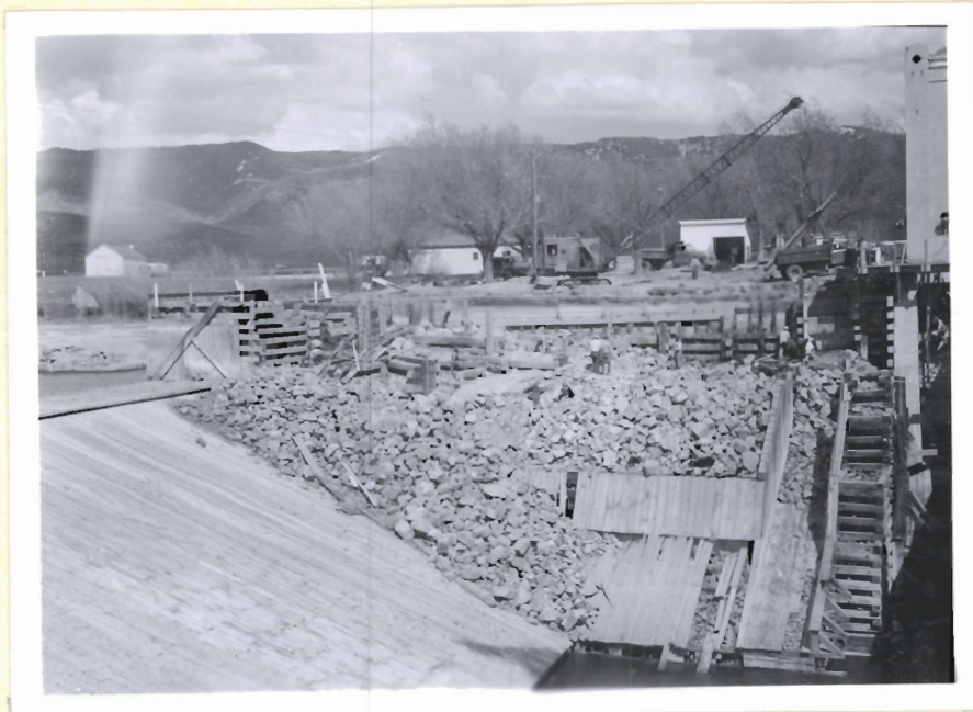
5-17-50 39/07 #71 Demolition of old dam down to elev. 1038 in progress. View easterly.
