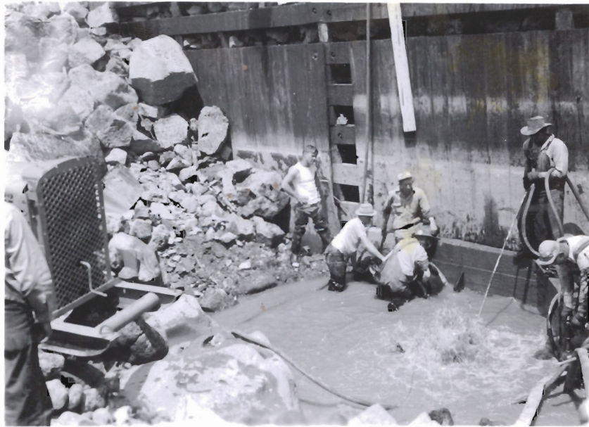
5-17-50 39109 #73 Closing sluice gate on downstream face of dam. View northwesterly.
