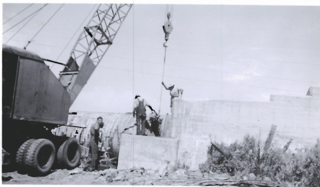
First hitch on valve to remove same to new location.
