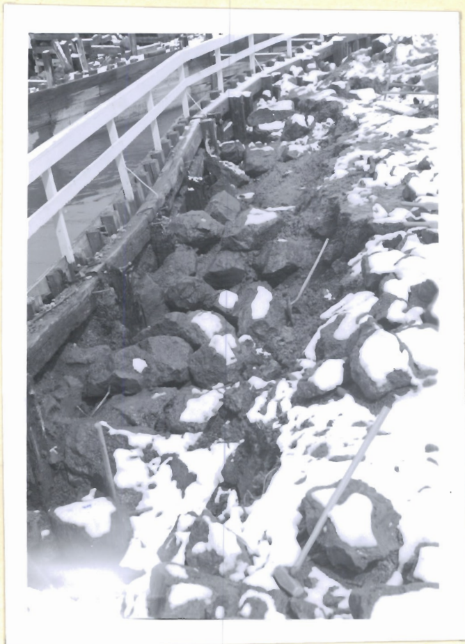
Looking northerly along east side of Intake No. 3 Flume. Rock rip-rap place east of flume.
