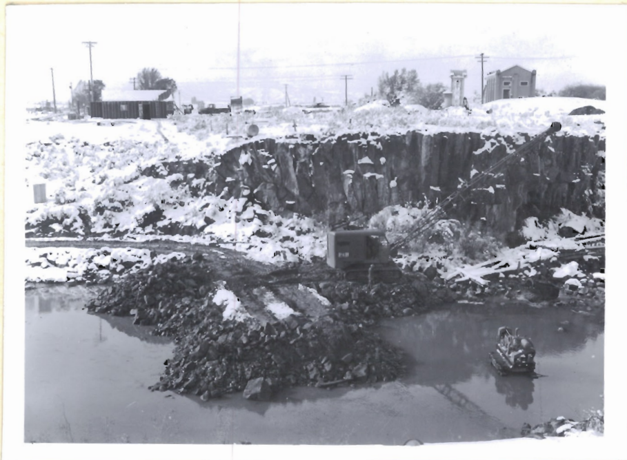
10-21-49 First unwatering pump set in place at lower right. Dragline excavating loose material and placing in lower doffer dam. 39039 View west.
