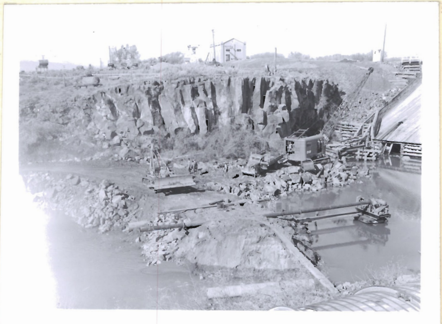
10-25-49 39040 Shows 12" pump installed at lower right. Crane setting 10" - 2 stage pump under old dam to pump water over dam into fore- bay.
