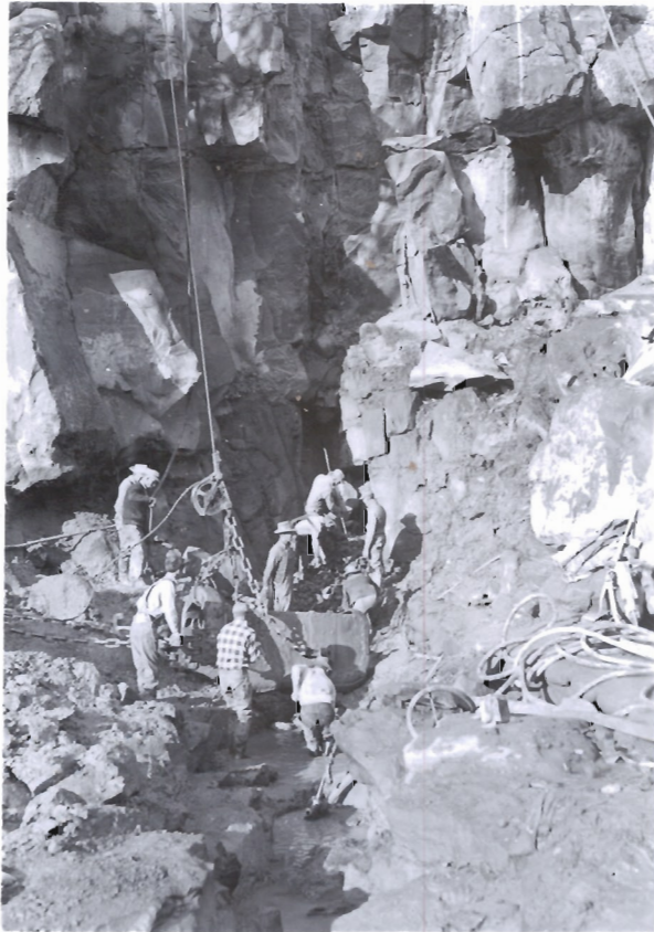
11-11-49 39047 #17 Cutoff wall excavation and channeling in west cliff.
