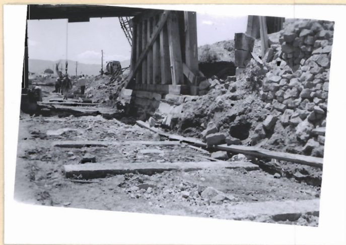
#9 RR Bridge over Grace #2 Flowline
