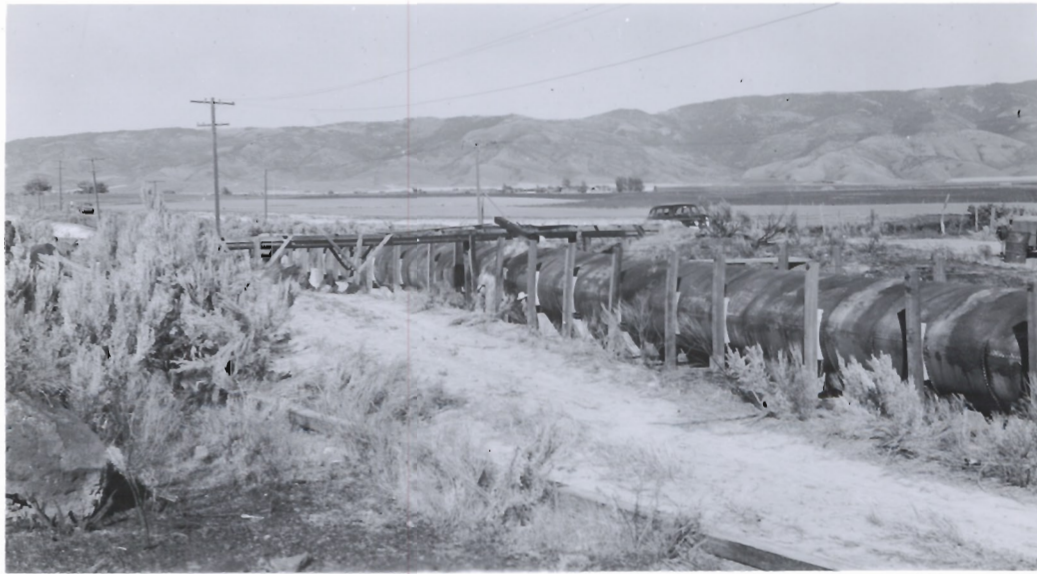
Steel section of Flowline 1 crossing over Flowline 2 after restoration and during filling. Note overflow from relief valve in front of irrigation flume crossing at center of picture. Also note vertical side braces with pillow blocks supporting pipe against distortion and egg shape of pipe at point of contact with pillow blocks. 7-27-48
