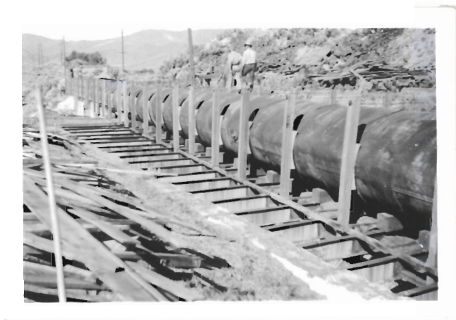
Inspecting restored section during filling. 7-27-48
