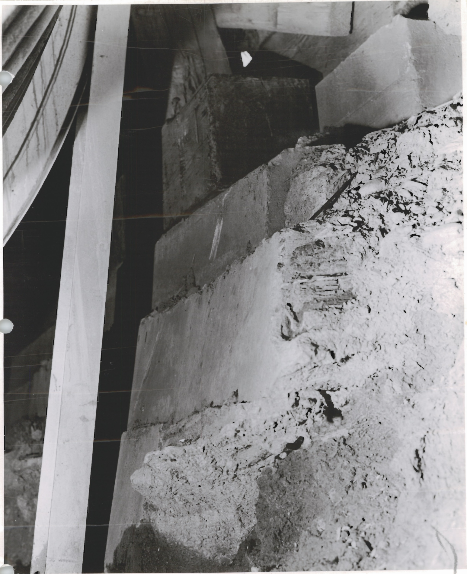
#6 UPRRCO. Bridge over Grace Flowline showing bridge footings east side of RR bridge - No. side of pipe looking down stream.
