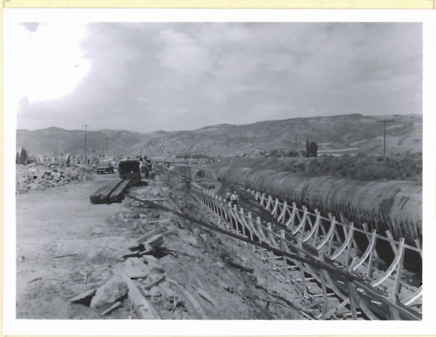
8-8-50 39025 Pipe erection in progress.
