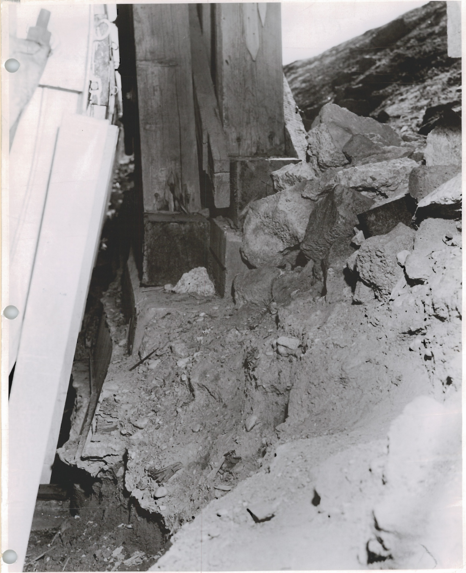
#1 UPRR Co. Bridge over Grace Flowline showing bridge footings
