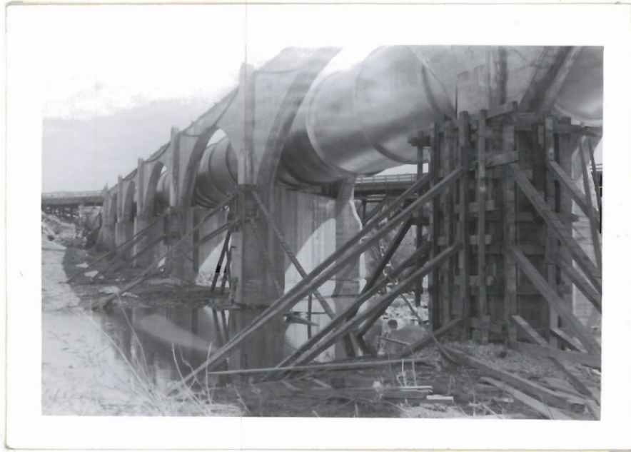
Pier #6 Right tangent - formed and ready for concrete. 8-12-52
