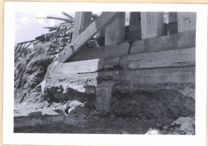
#10 RR Abutment over Grace #2 Flowline.
