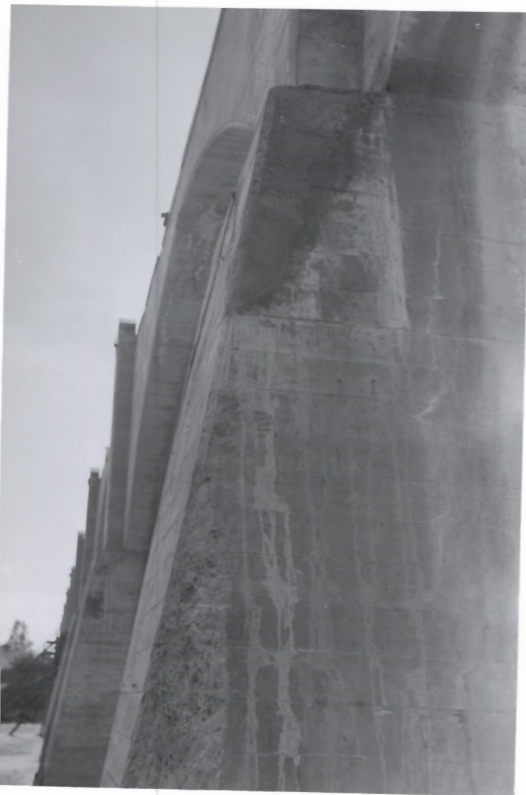
Pier #5 left tangent. Top repairs completed. 8-14-52
