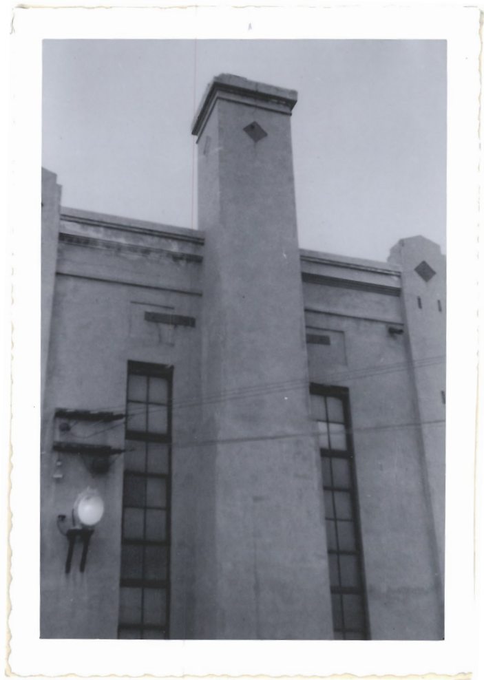
View of East wall and stack
