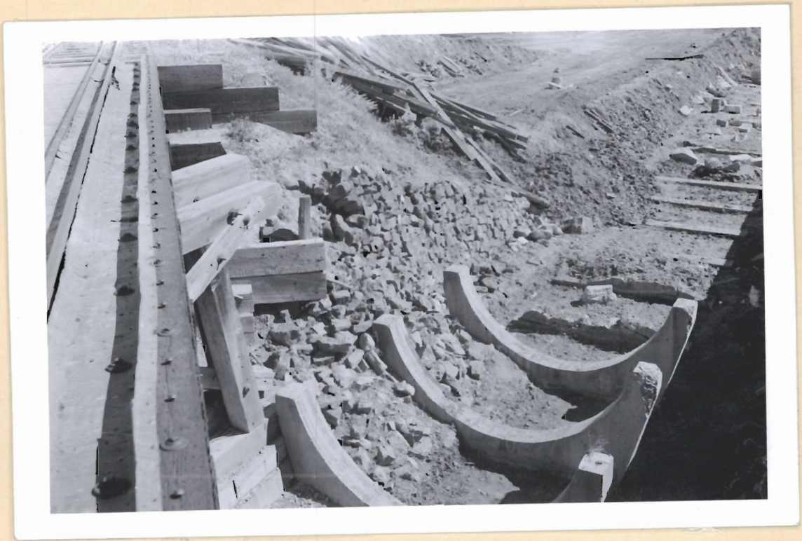
#8 Pipe removed from under OSL RR Bridge.
