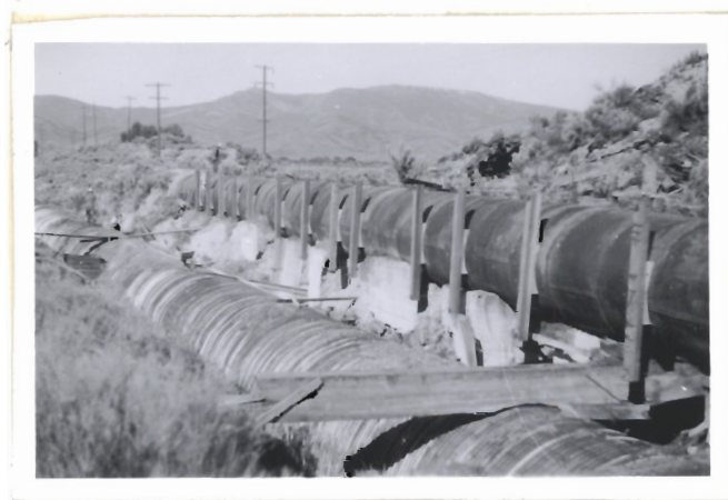
Portion of section collapsed 7-14-48 after restoration and filling and after replacing and tightening braces loosened in filling. Note rounded out appearance of top arc of pipe. It was this rounding out that pulled the egg shaped sides back to place and loosened the braces during last stages of filling. 7-28-48
