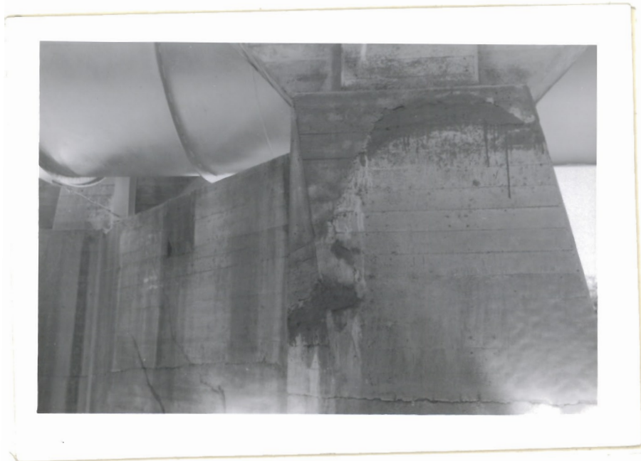
Pier #4 right tangent. Repairs complete. 8-14-52
