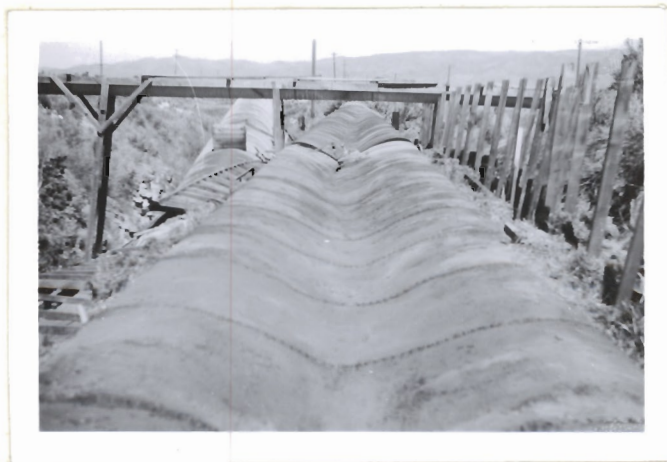
Flow line #1. Collapsed while draining 7-14-48 Protecting shed and straw mostly removed. Some shed studs standing or lying on sides. 7-16-48
