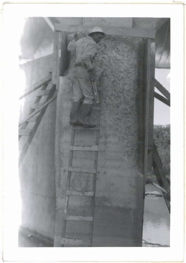
Pier #5 right tangent. Chipped & ready for forms. 8-9-52
