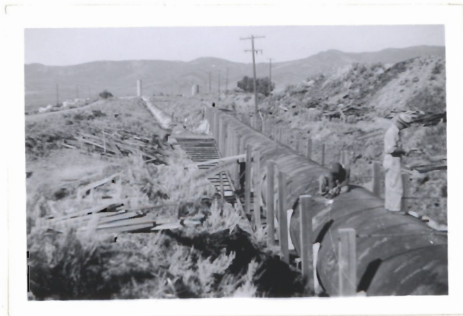
Tightening turnbuckled tension rods on protective bracing. 7-27-48
