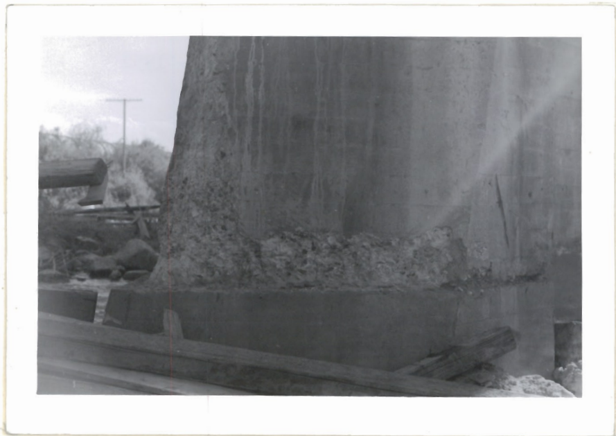
Pier #5 left tangent. Base deteriorated concrete chipped away, ready for forming. 8-10-52
