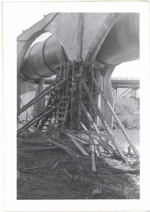
#6 Pier Rt. Tan. looking SE. Formed, ready for concrete. 8-12-52
