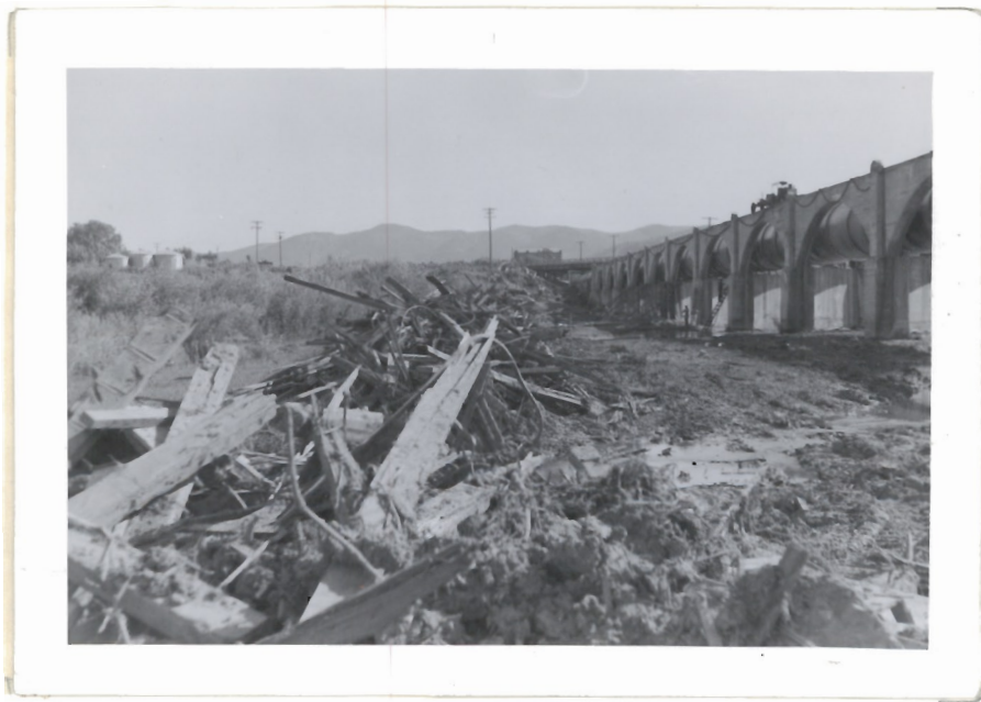
View of debris in river bottom downstream from pipe crossing. Looking NW 8-7-52
