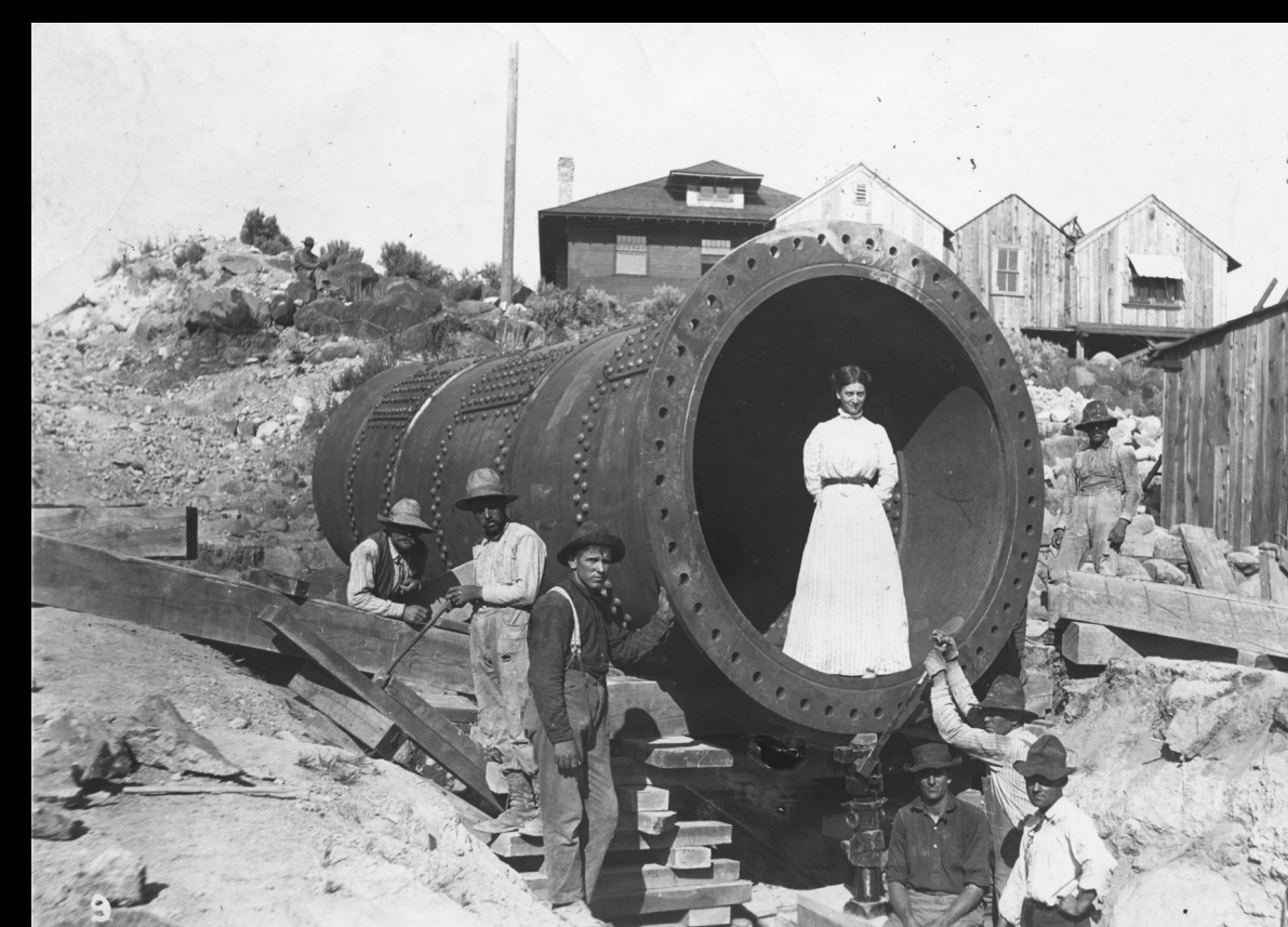
Construction crew transporting penstock section.
