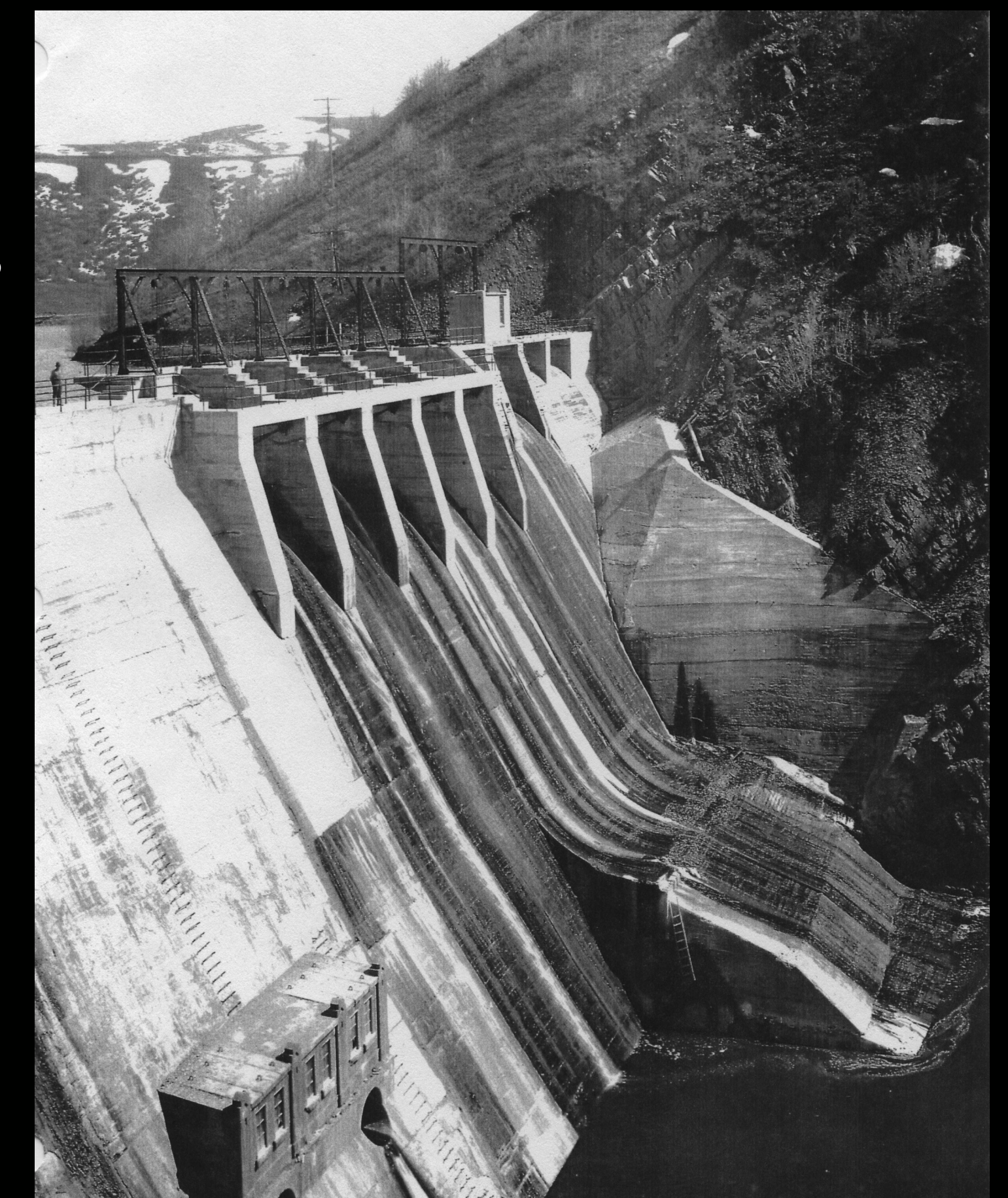
Overview of the Oneida concrete dam showing overflow control gates.
