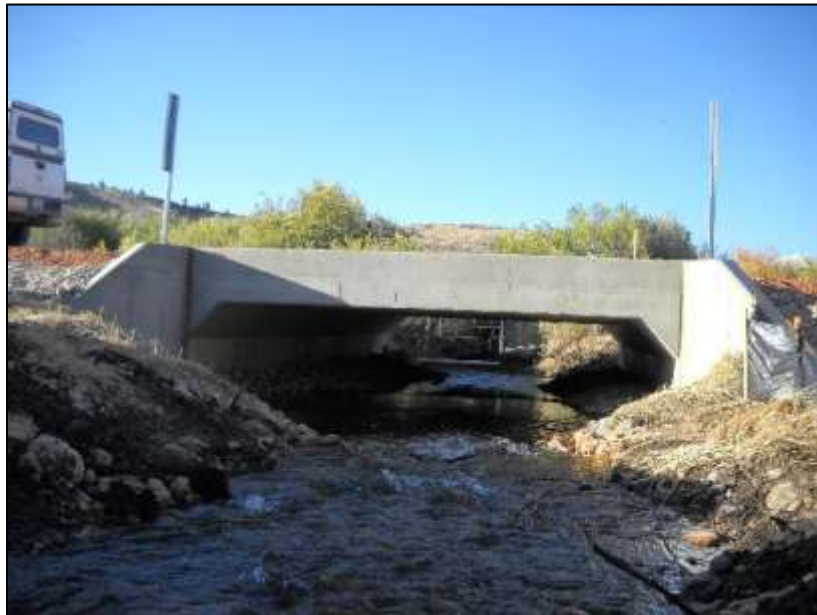
Eightmile Creek/Nounan Road crossing after culvert replacement
