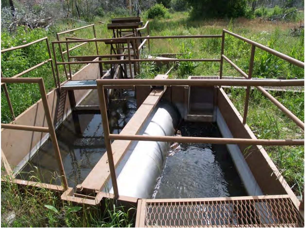
Lower Cottonwood Diversion
