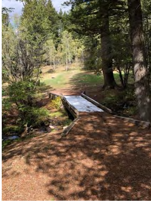
Eight Mile Canyon #5 Bridge #1
