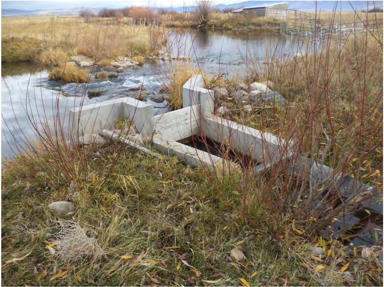
Roy Bunderson Irrigation Structure
