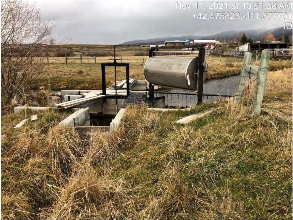
Alleman Dam Removal
