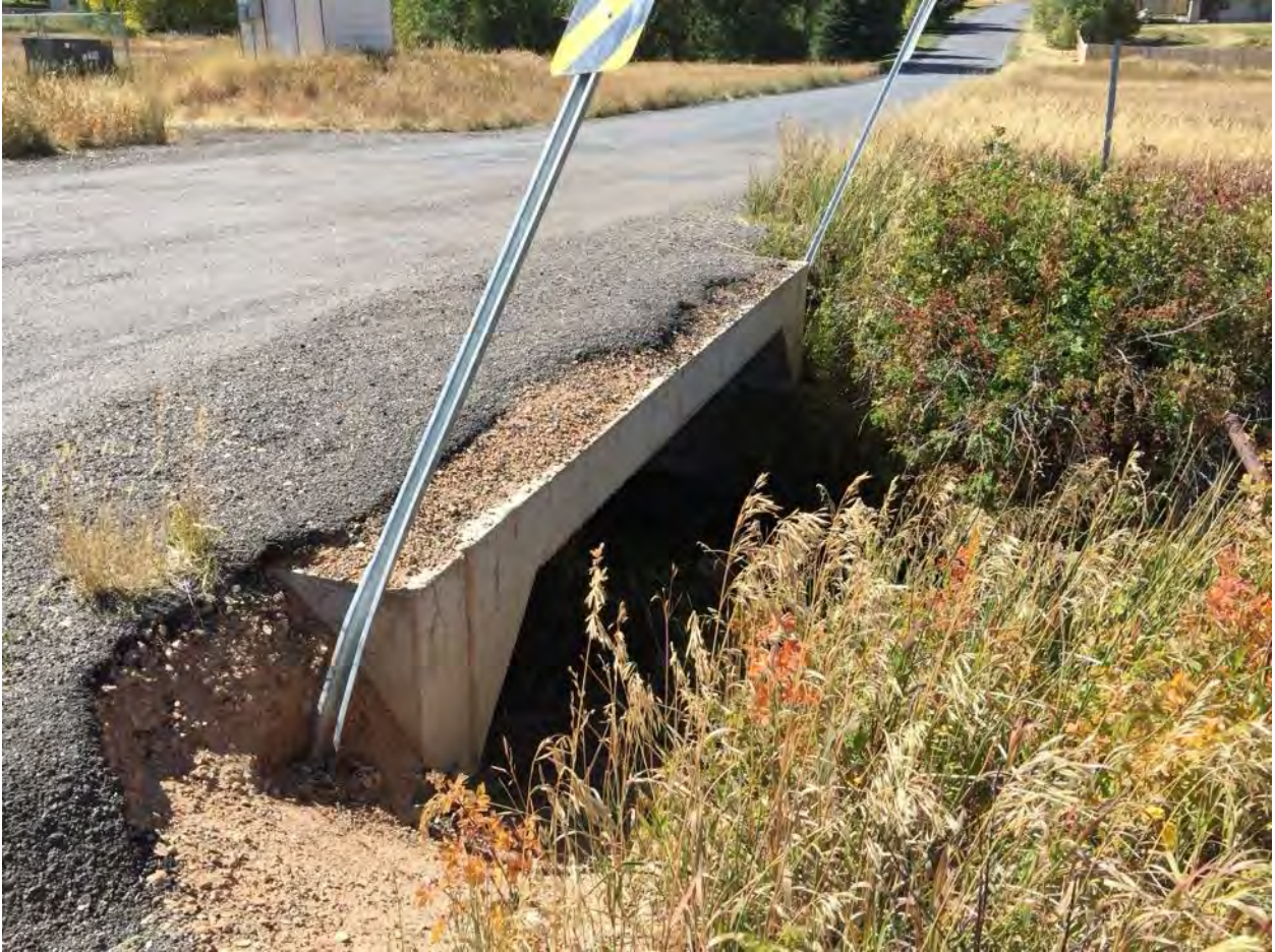
Bailey Creek Culvert
