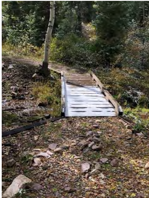
Eight Mile Canyon #5 Bridge #2
