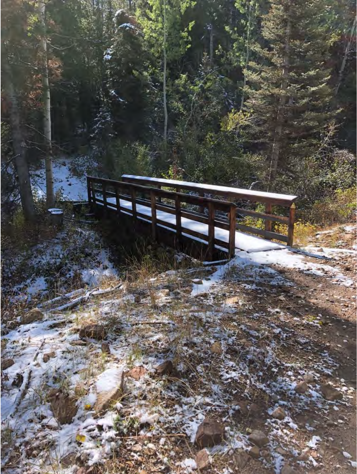
Coop Trail Crossing Bridge
