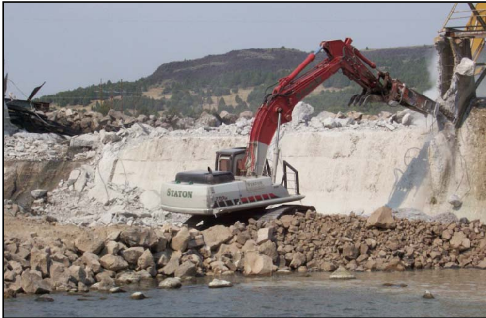
Demolition of the Cove Dam near Grace, Idaho, during late summer 2006.
