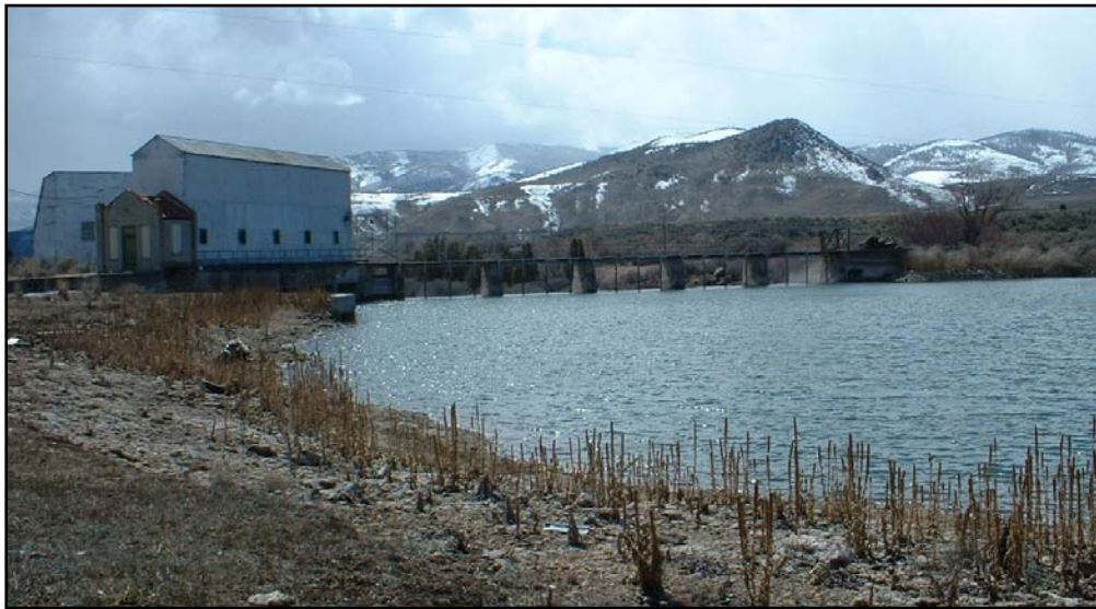
The Cove Hydroelectric Development forebay near Grace, Idaho, during summer 2005.
