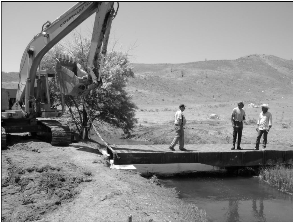
Figure 3. Bridge placed over a tributary to the Bear River to move the Harris's cattle wintering operation away from a sensitive spring complex.
