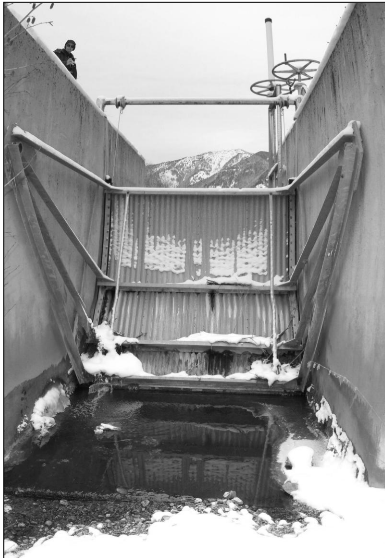
Figure 5. Headgate to the hydroelectric facility's water diversion on Georgetown Creek.
