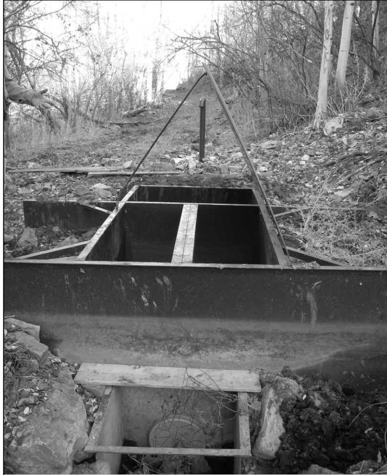
Figure 4. Fish screen installed on Hoops Creek to prevent Bonneville cutthroat trout from entering an irrigation diversion.
