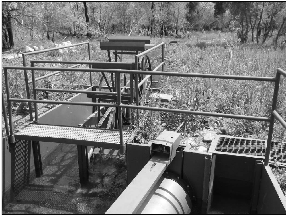
Figure 3. New headgate on Cottonwood Creek designed to prevent Bonneville cutthroat trout and other fish from being lost when water is diverted to irrigate pastures. This project, now complete, was funded by the ECC in 2005.
