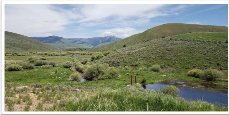
View of diversion with ponded water upstream and straightened ditched channel downstream.
