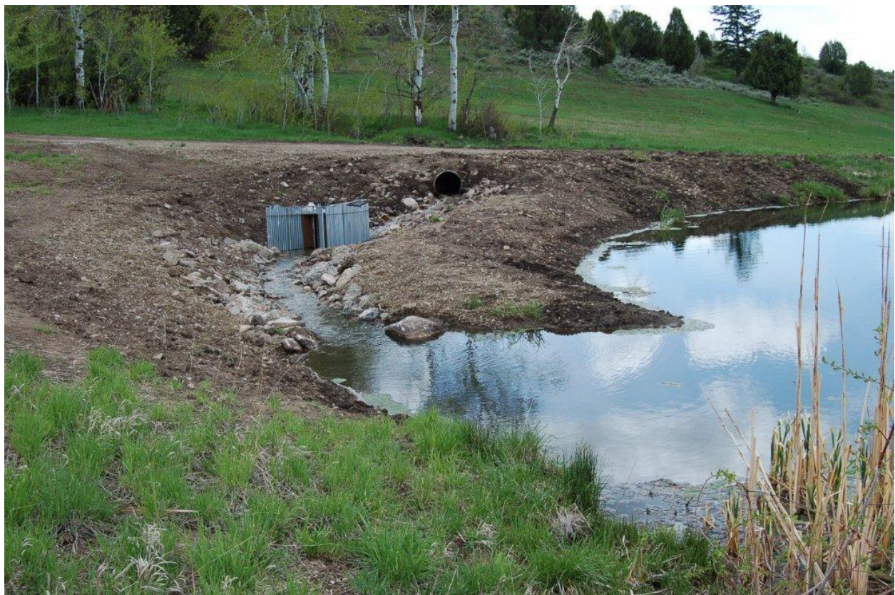
Figure 2. Attraction channel and trap box used to collect mature BCT that swim out of the pond at maturation.
