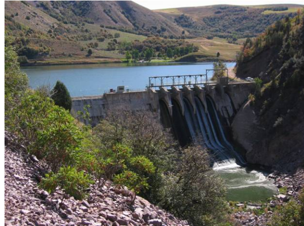
Photo 1. Oneida Reservoir and dam.
