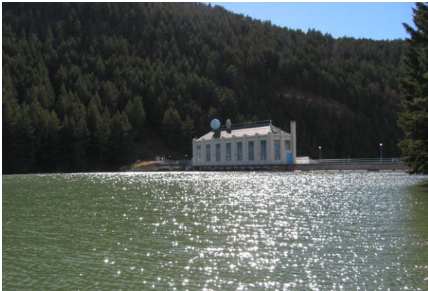
Photo 2. Soda Powerhouse and Alexander Reservoir.
