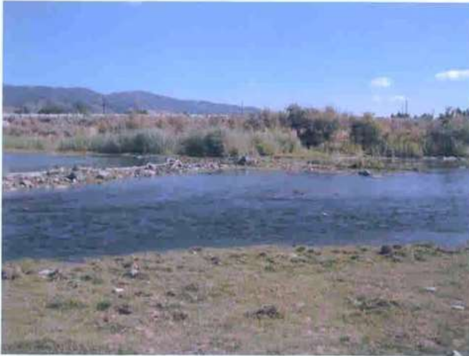
Figure 5 - Gravel and Rock Berm from river right with plastic installed to consolidate flows.
