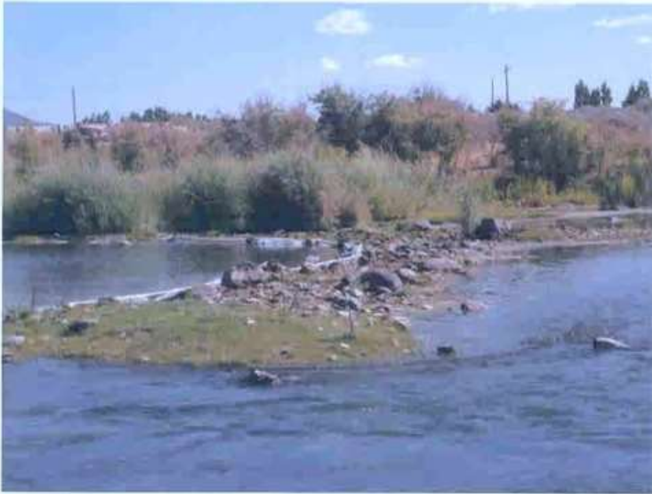
Figure 3 - Gravel and Rock Berm from river right with plastic installed to consolidate flows.
