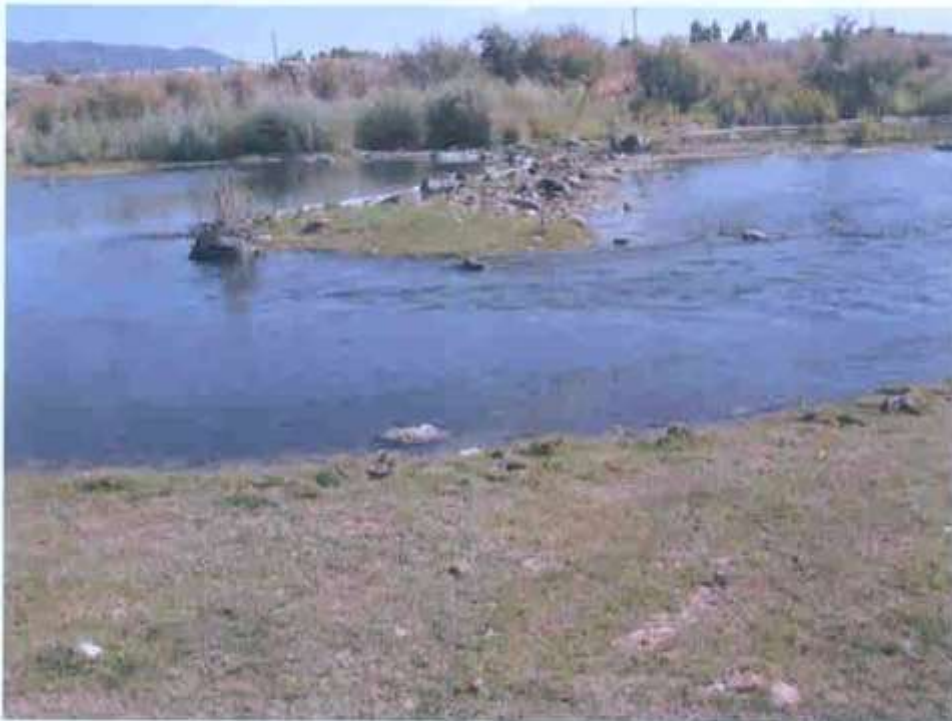
Figure 4 - Gravel and Rock Berm from river right with plastic installed to consolidate flows.
