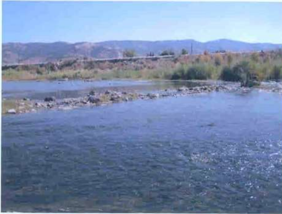
Figure 1 - Grace Gage site gravel and rock berm in river.
