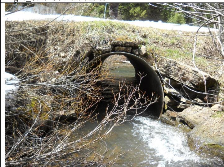
Eight_8.47 Culvert Inlet and Rip-rap
