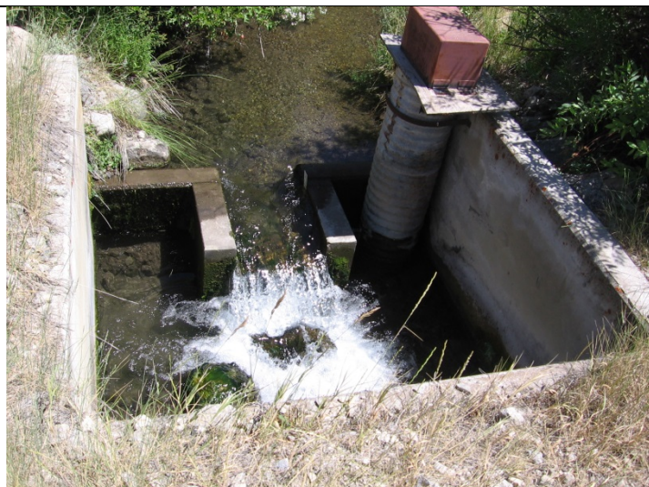
Gtown_4.85 Culvert Inlet and flow measuring weir
