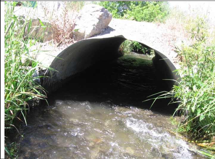
Gtown_2.19 Culvert inlet and rip-rap
