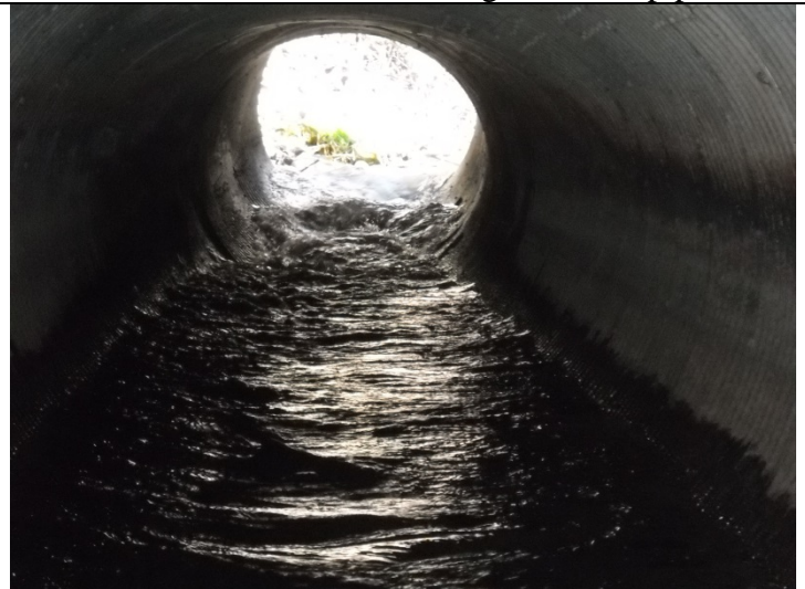
Gtown_3.91 Culvert inlet, grade break in culvert
