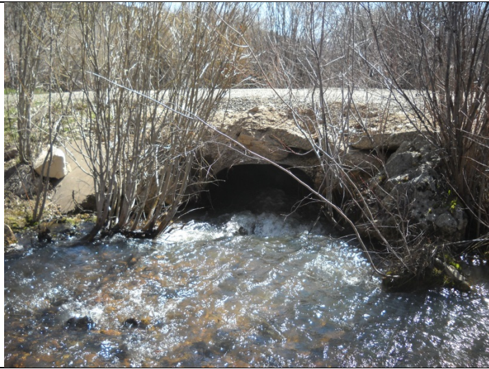
Stauf_7.5 Culvert Inlet with rip-rap
