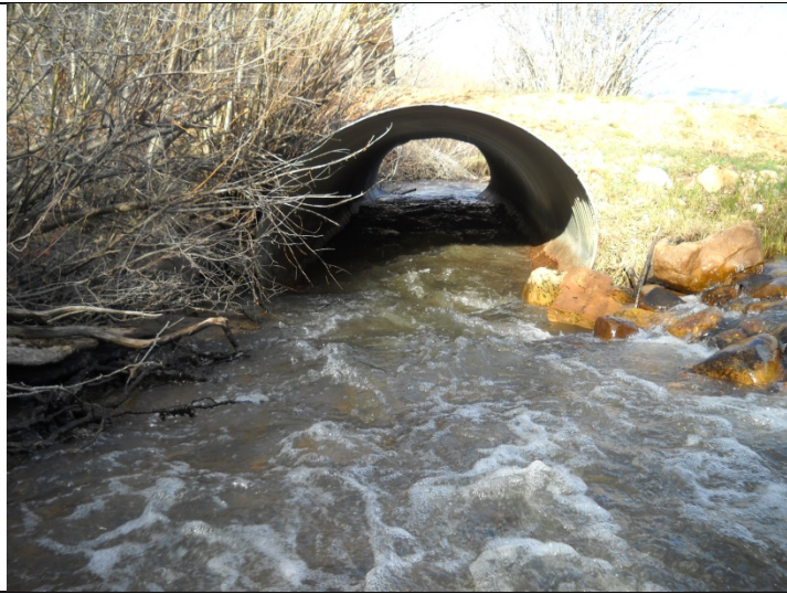
Stauf_7.71 Culvert Inlet with rip-rap
