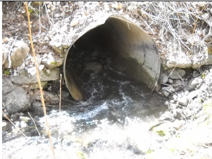
Gtown_3.91 Culvert inlet, poor alignment
