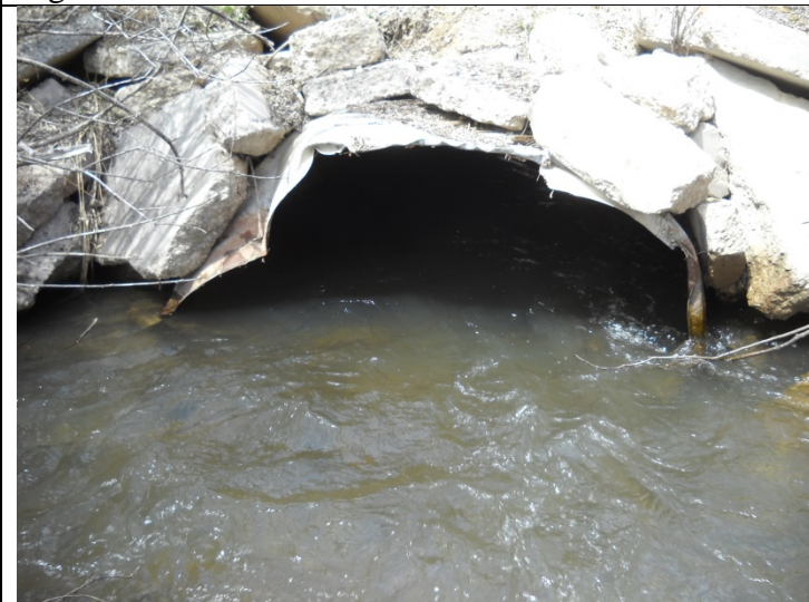
Eight_2.42 Culvert Inlet (bent inlet, armor present)
