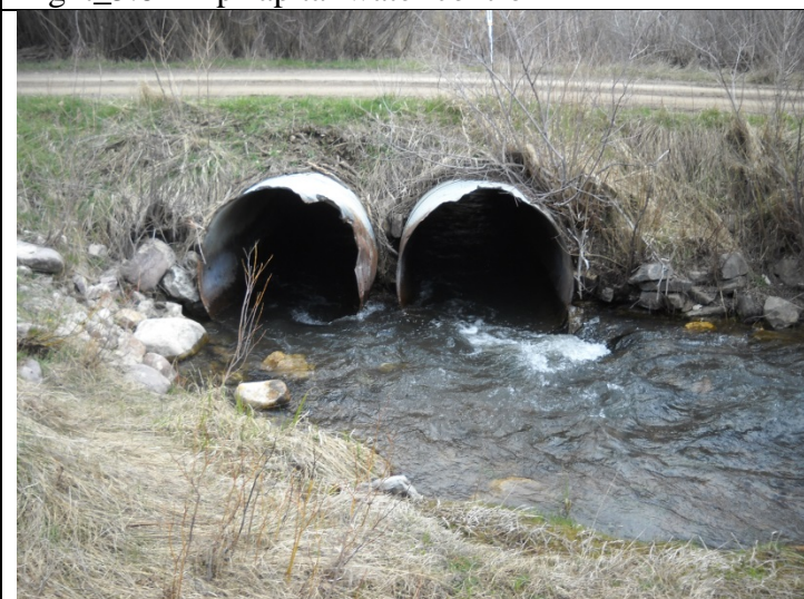
Eight_5.81 Culvert Inlet, poor alignment with stream
