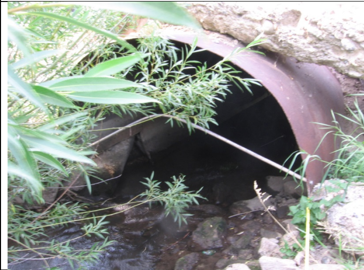
Gtown_1.35 Culvert inlet and rip-rap
