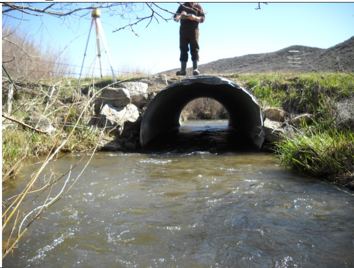
Gtown_0.07 Culvert inlet and rip-rap
