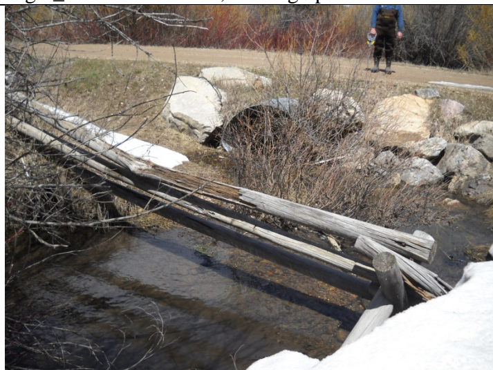
Eight_7.69B Culvert Inlet, poor alignment with stream
