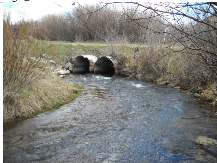
Eight_5.81 Culvert inlet, poor alignment with stream
