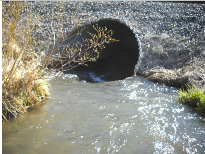
Gtown_0.04 Culvert inlet and rip-rap
