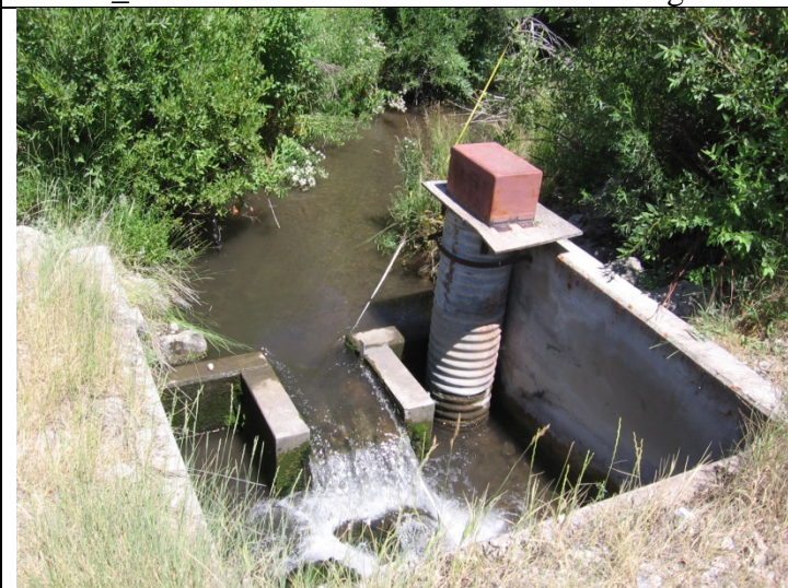
Gtown_4.85 Flow measuring weir
