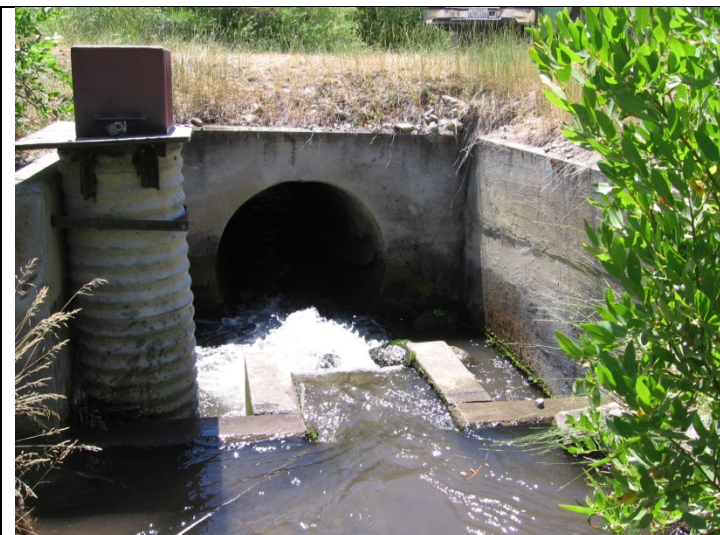
Gtown_4.85 Culvert Inlet with flow measuring weir
