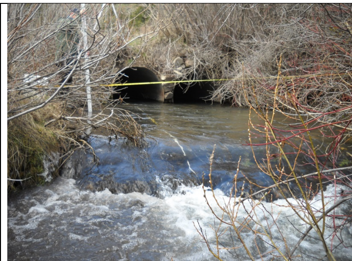
Eight_5.81 Culvert outlet and rip-rap Tailwater control
