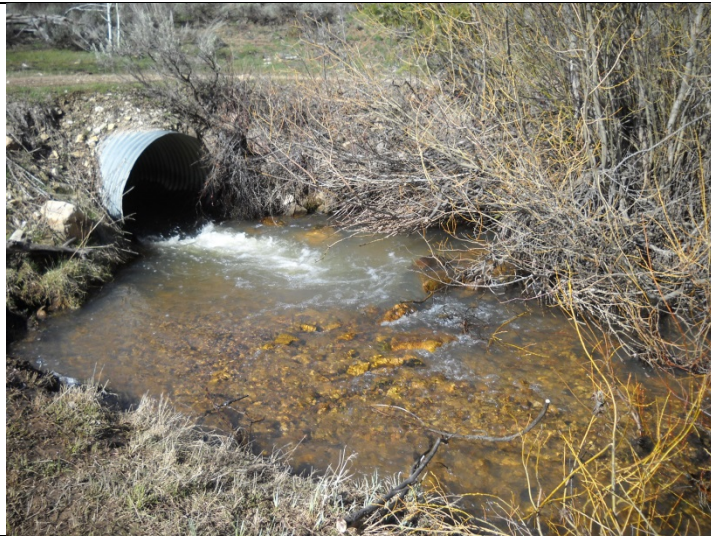
Stauf_8.66 Culvert outlet and tailwater control
