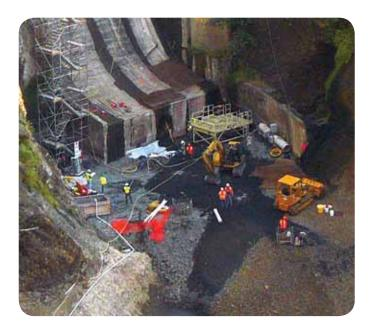
In early August 2011, Northwestern Lake and its associated boat ramps were closed to all activities, in order to ensure public safety. The water level was also drawn down 10 feet in order to allow the drain tunnel at the base of the dam to be constructed prior to the breaching of the dam in late October.
