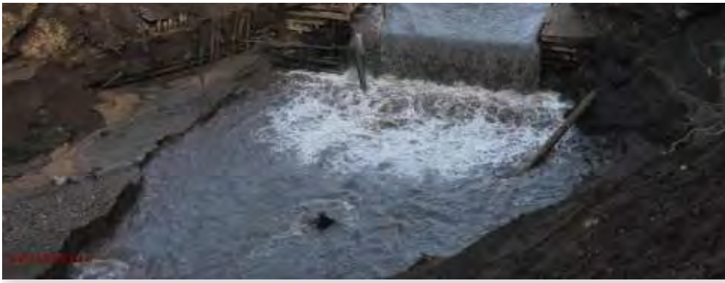
November 2011 View of #2 (upstream) coffer dam.
