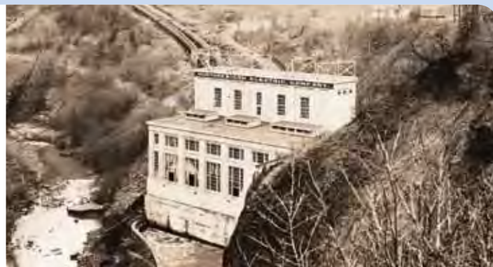
Condit Powerhouse during the early years of operation
