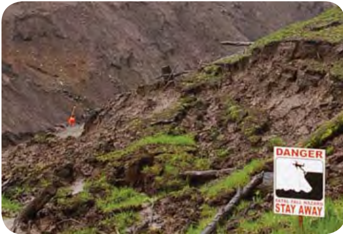
Public safety is PacifiCorp's top priority and we ask the public to obey all signs in the construction areas.
