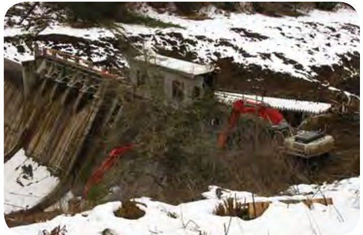
Decommissioning work continued throughout the winter at Condit Dam.
