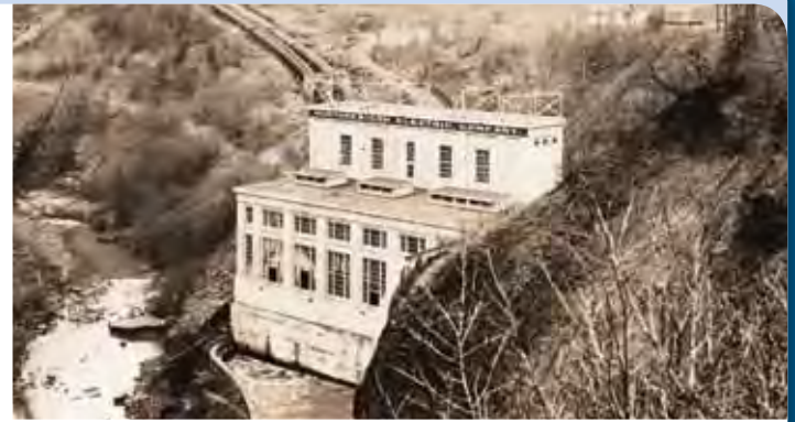
Condit Powerhouse during the early years of operation
