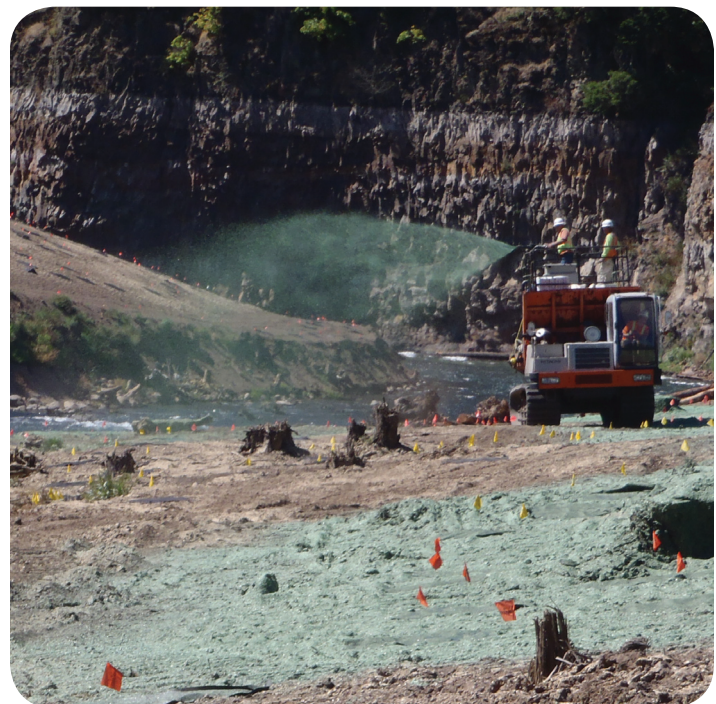
Recently, hydroseeding and mulching work has taken place to further restore the landscape along the river.
