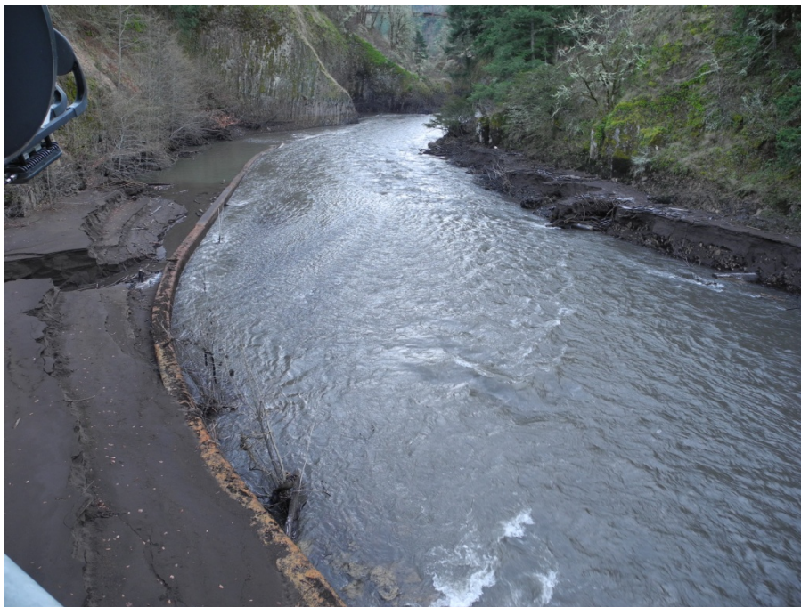
Photo 1. Downstream view of the White Salmon River at the powerhouse. Temporary bed sediment levels can be inferred from the deposition on river right. On river left the powerhouse tailrace is filled with sediment. Photo date December 7, 2011.
