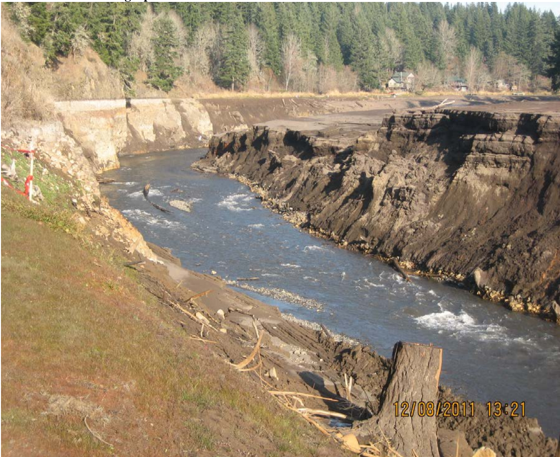
Photo Point #3 Looking Upstream 12.08.11 (Significant reservoir erosion ceased)
