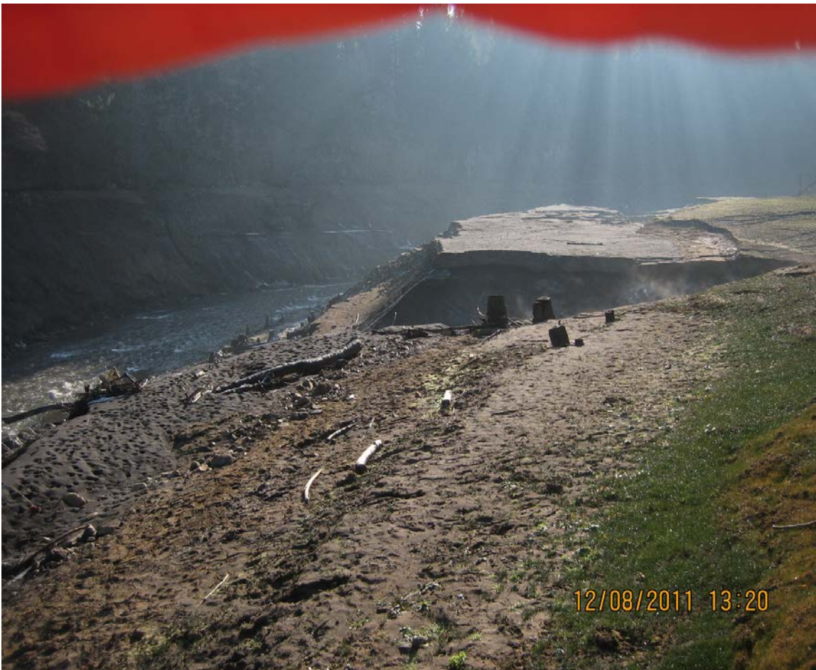
Photo Point #3 Looking Downstream 12.08.11 (Significant reservoir erosion ceased)
