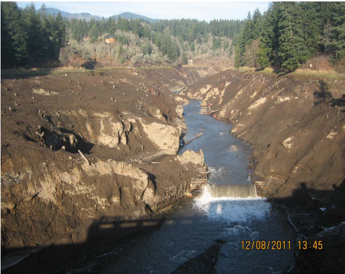
Photo Point #6 Looking Upstream 12.08.11 (Significant reservoir erosion ceased)
