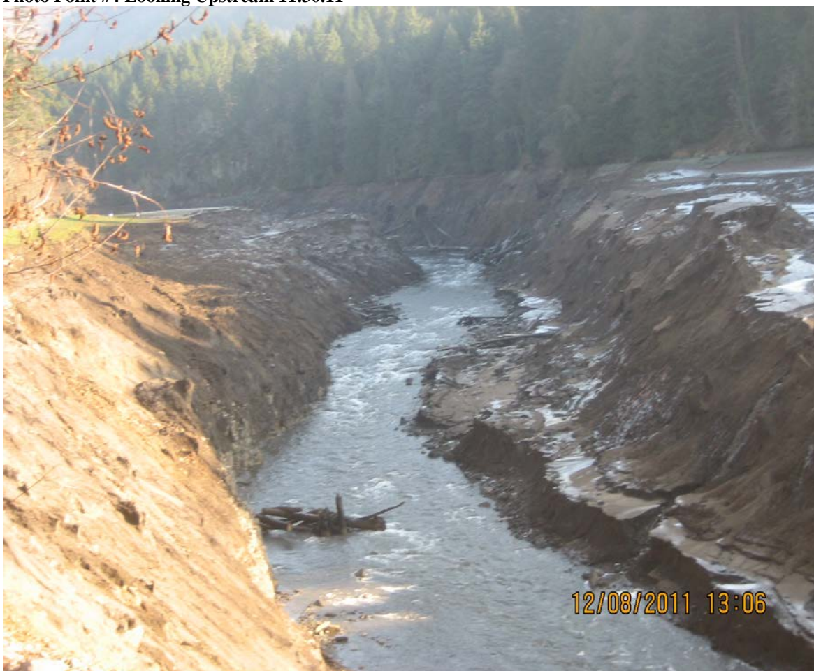
Photo Point #4 Looking Upstream 12.08.11 (Significant reservoir erosion ceased)
