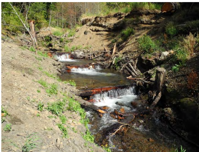
Log check dams installed on Mill Creek.
