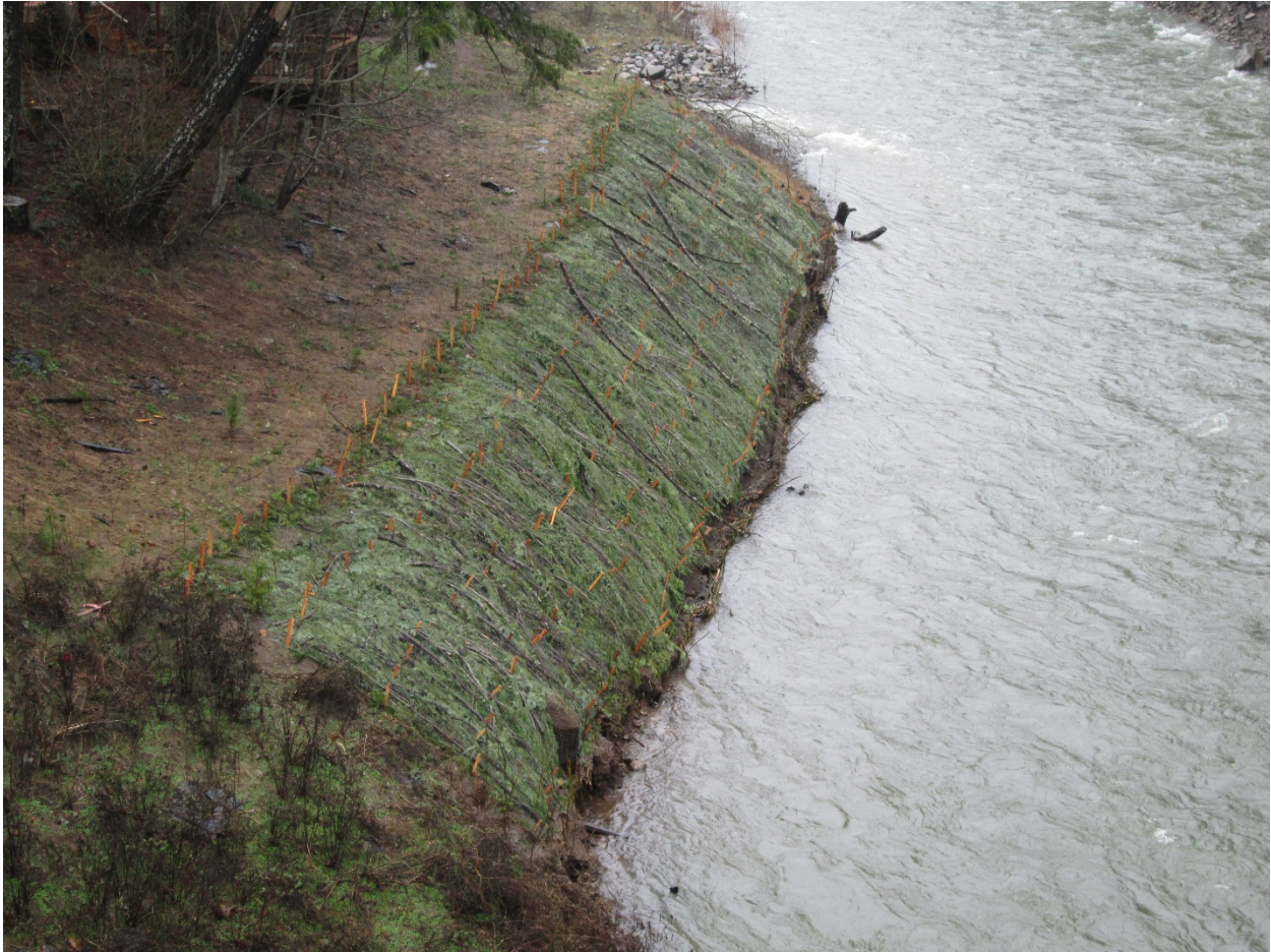
View of right bank just upstream of Northwestern Lake Bridge in the area repaired during the fall of 2014. Photo taken on February 9, 2015 during the highest-flow event of the reporting period. Flow was approximately 2,200 cfs at the time of the photo and the flow peaked at 2,820 cfs on February 10.
