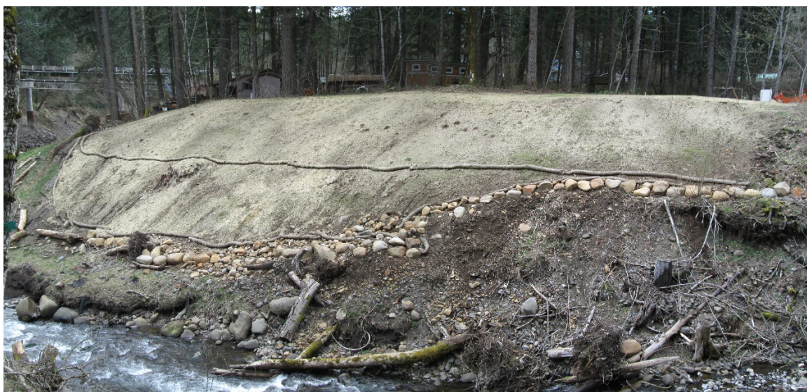
Cabin 9DF Removal Site at the confluence of Buck Creek and the White Salmon River
