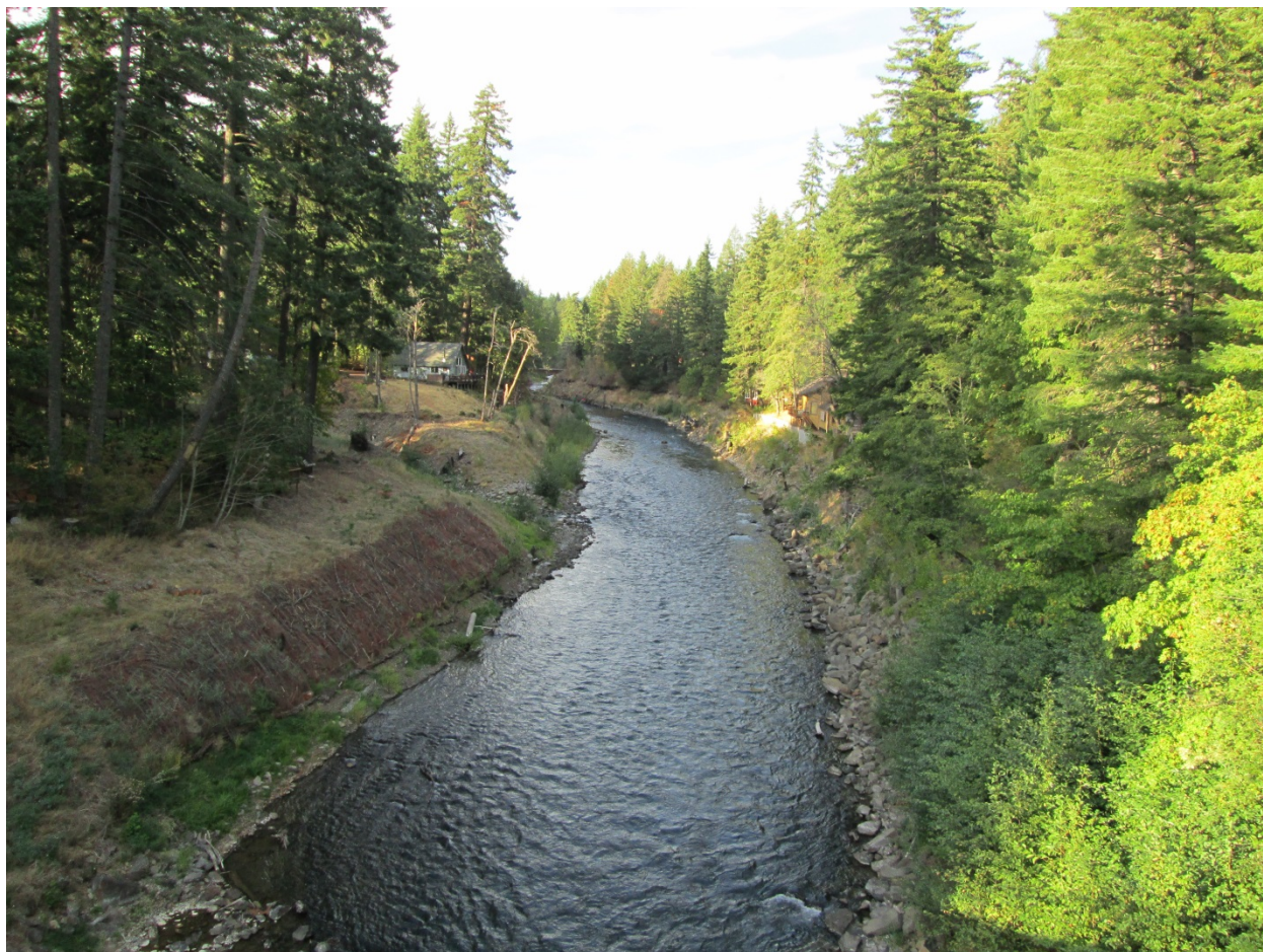
View upstream from Northwestern Lake Bridge – September 9, 2015.
