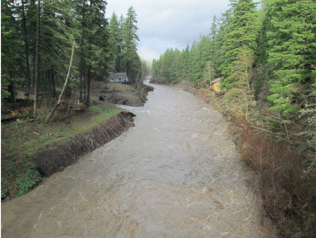
View upstream from Northwestern Lake Bridge during 50-year recurrence flow event. Bank repair measures on the right bank were undermined. - December 9, 2015
