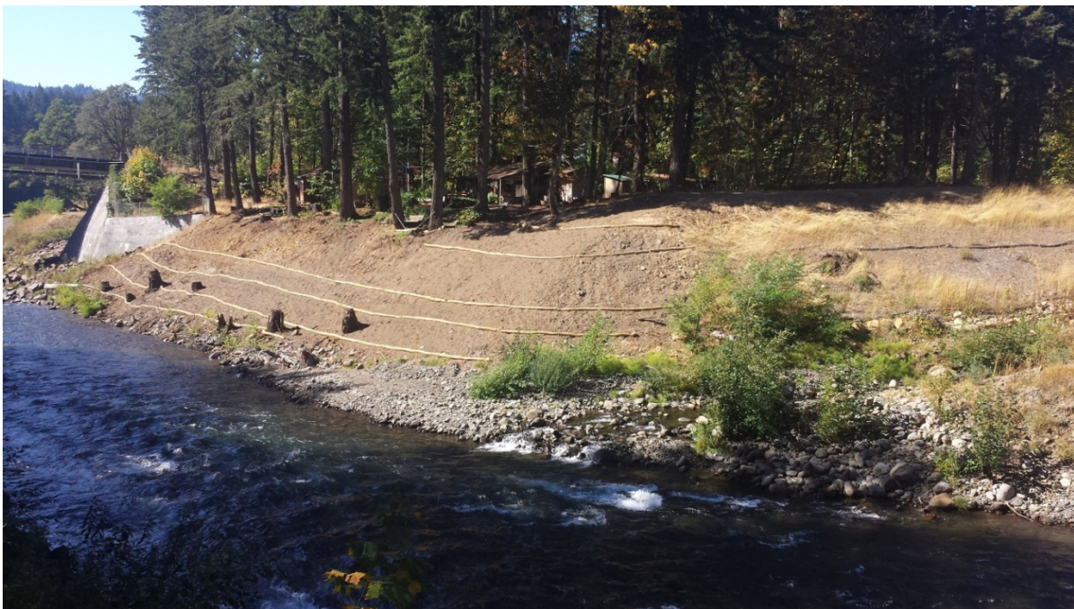
Right bank from Buck Creek to Northwestern Lake Bridge after grading the bank during August 2016. September 21, 2016
