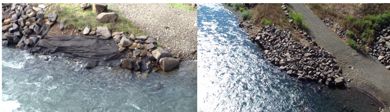
Views of the Northwestern Park boater take-out before and after repairs to the riprap slope protection. March 3, 2016 and September 21, 2016
