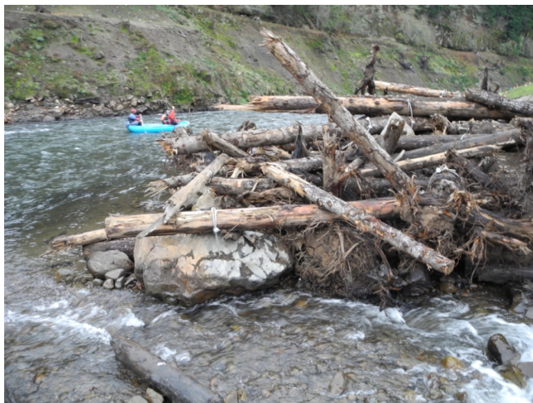
ELJs constructed at the side of the White Salmon River.
