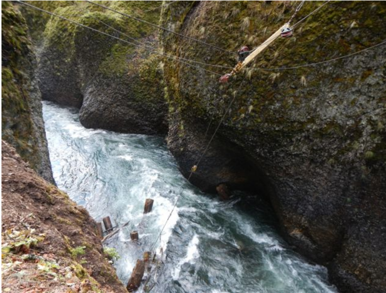
Logjam at The Narrows September, 2012. Cable yarder and wire slings were used to pull out logs.
