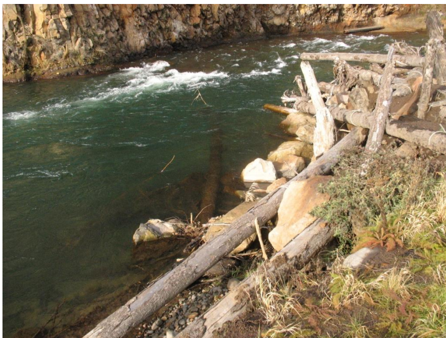
Engineered Log Jam No. 4 on the banks of the White Salmon River – December 2013
