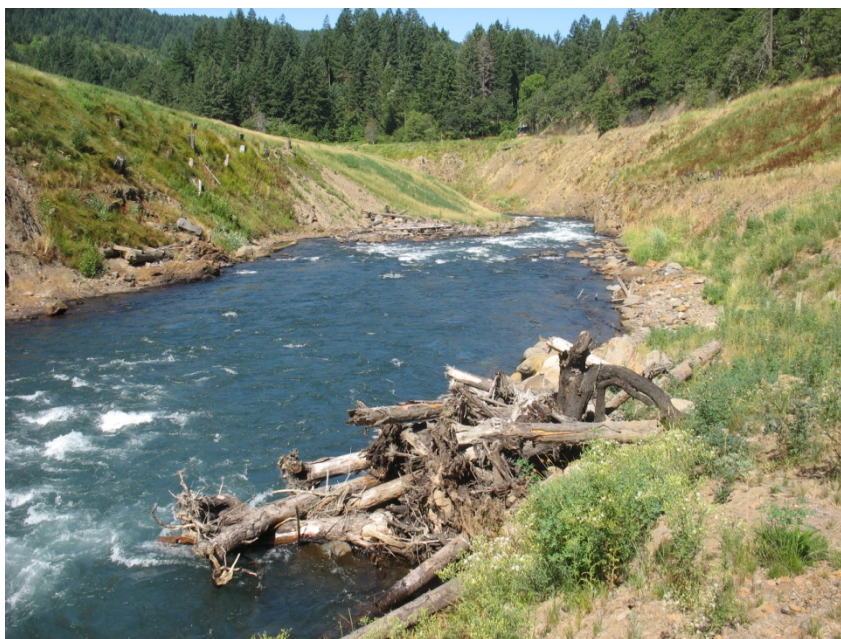
Engineered Log Jams constructed on the banks of the White Salmon River within the former reservoir area – December 2013.
