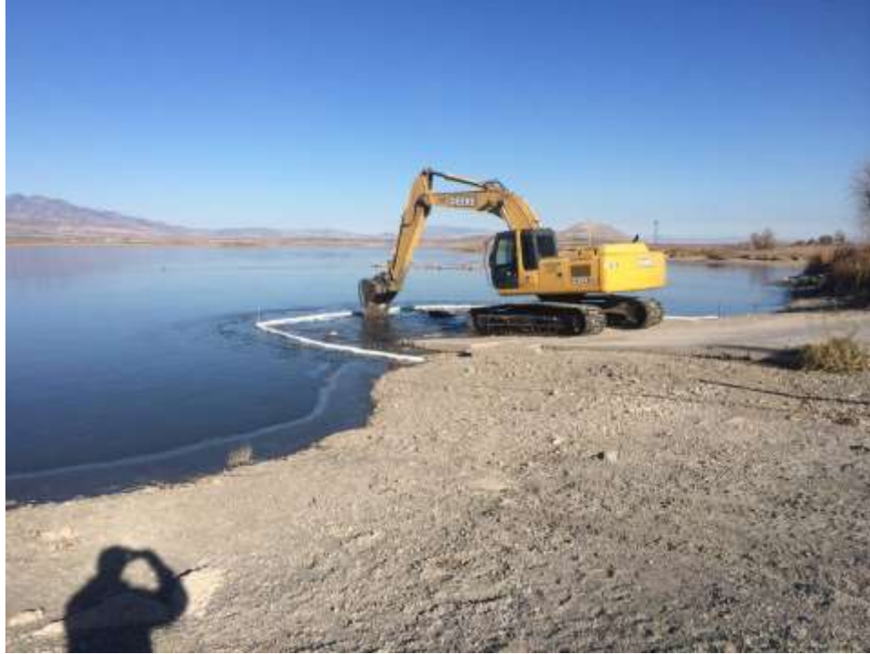
Photo D-7. Major ramp repair work at Benson Marina during reservoir draw down.
